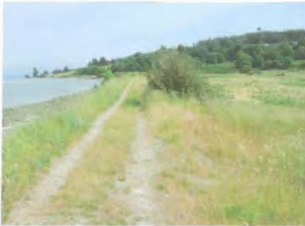
Figure 5. View of Dike on the property.
