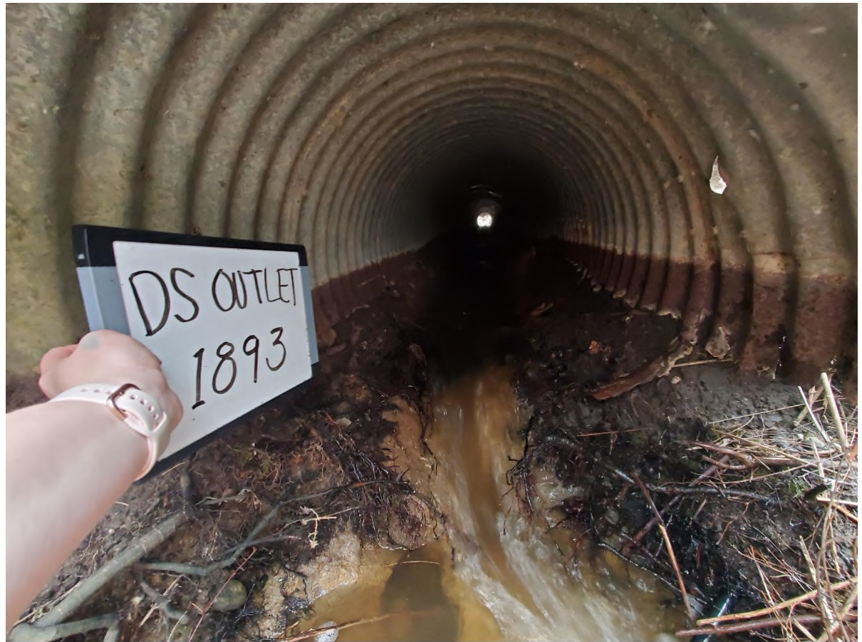
Figure 5 The outlet of the Western culvert.
