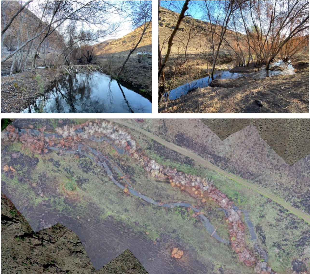
Figure 8. Example of a beaver dam analogues built on the mainstem of Charley Creek (top left- view from downstream; and top right – view from upstream) that forced a side-channel connection of over 250 m (bottom photo). Multiple smaller BDAs were built in side-channel to inundate more floodplain and connect other side-channels. Stream is flowing left to right, mainstem is mostly obscured by riparian trees, and the side-channel is in the open.
