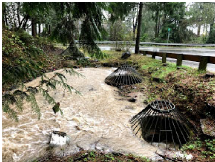
Photo 3. Bypass activated during high flow event (12/20/19)
