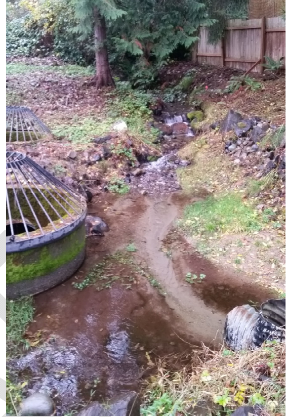
Photo 2. Sedimentation basin upstream of ELSP
