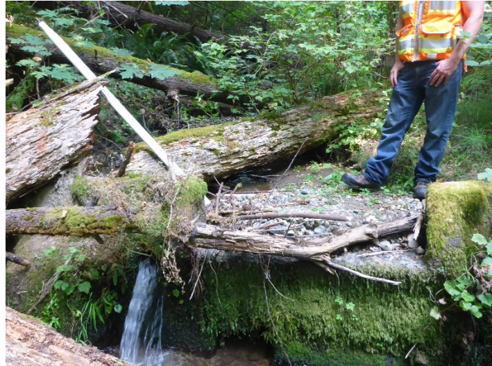
Photo 5. Diversion dam 500 feet upstream of ELSP
