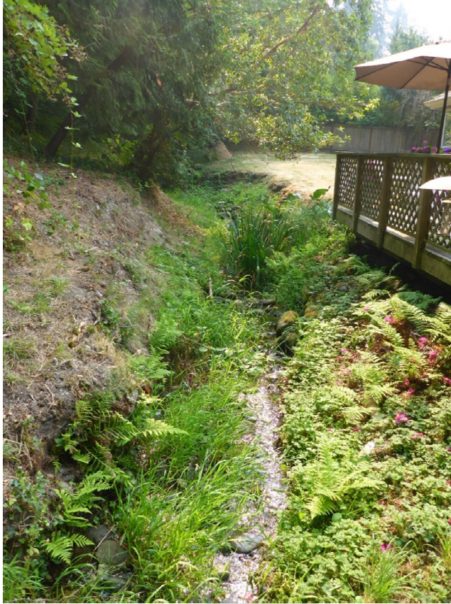
Photo 1. Creek channel at exit of ravine
