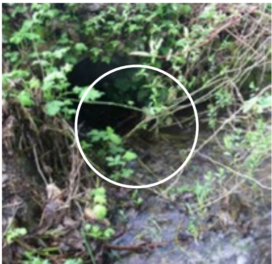
3 Looking downstream at culvert under East Lake Sammamish Parkway. The stream channel takes a 90° turn into the culvert, which creates problems with sediment transport and debris accumulation. In addition, velocities in this culvert are high during moderate peak flows, and the culvert outfall has a drop that impedes fish passage.
