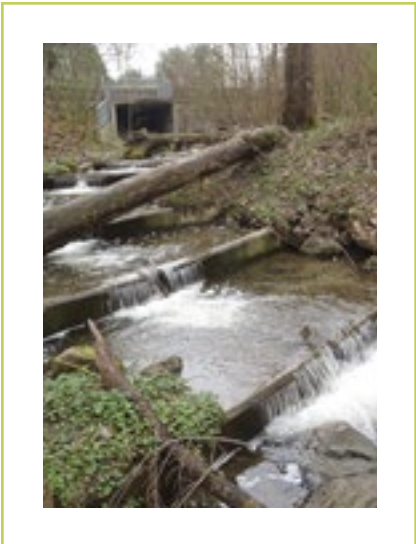
Figure 18. Concrete weirs downstream of West Lake Sammamish Parkway (photo credit: Tom Hardy, City of Redmond).
