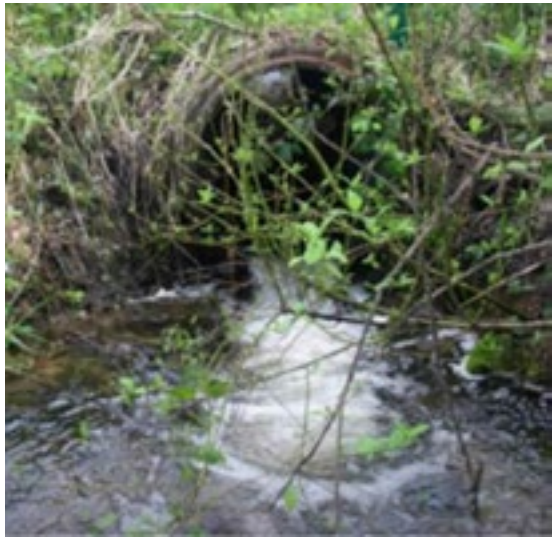
2 Looking upstream to culvert under multi-use path. This culvert impedes fish passage due to vertical water drops at both the inlet and outfall, as well as high velocities within the pipe itself during high water streamflows.
