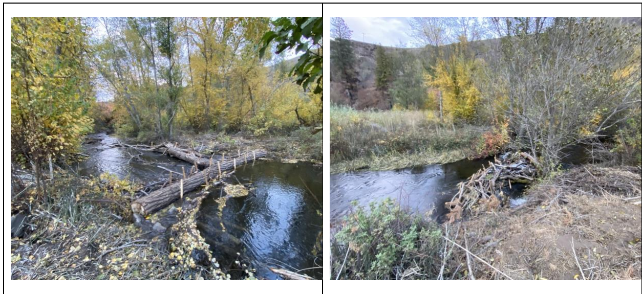
Figure 11. Example of a new post-assisted log structure (left) and the addition of a LWD and posts added to an existing PALS (right) to increase channel complexity, promote increased overbank flow frequency and floodplain connection on the North Fork.
