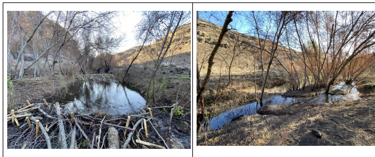
Figure 9. Example of a primary and secondary beaver dam analogue on the mainstem of Charley Creek viewed from downstream (left) and the mainstem and reconnected side-channel viewed from upstream (right).
