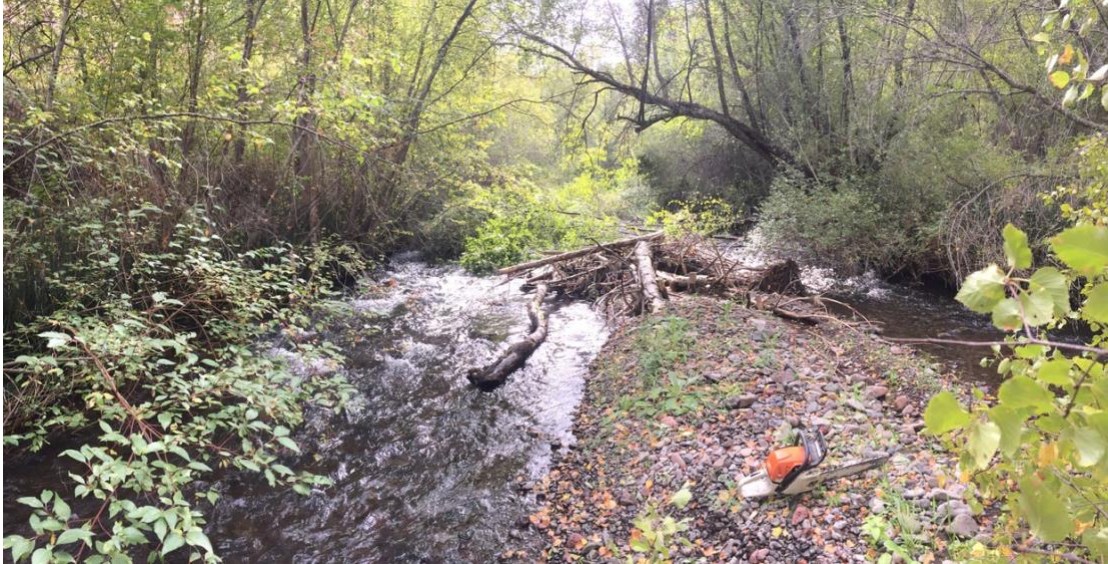
Figure 15. Post -restoration conditions in North Fork Asotin Creek – mid-channel post assisted log structure splitting flow and creating downstream mid-channel bar.
