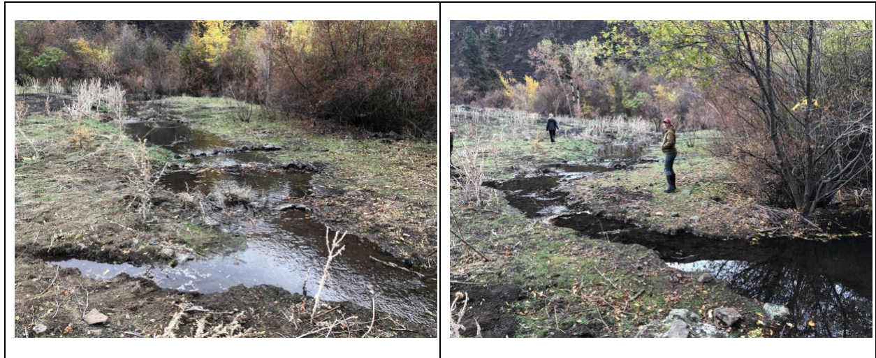
Figure 10. Examples of a newly connected side-channels in Charley Creek with a series of small beaver dam analogues to create pools and spread water across floodplain.
