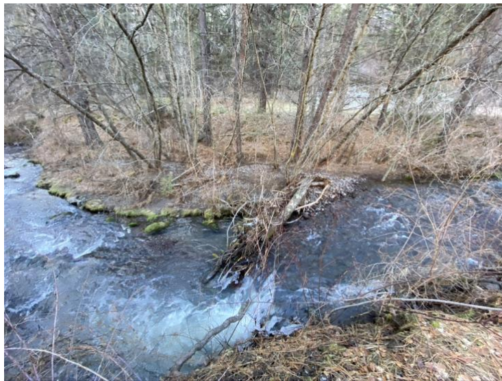
Figure 14. Post -restoration conditions in Charley Creek – bank attached post-assisted log structure forcing flow against river left bank, creating eddy pool downstream, and forcing overbank flow and forming upstream and downstream bars on river right.
