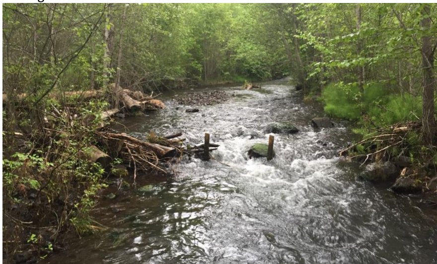
Figure 3. Example of a partly intact post-assisted log structure that was enhanced with the addition of more large woody debris.
