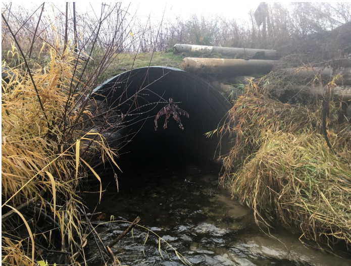
Lower project area – culvert to be replaced with bridge. Note concrete tubes used to stabilize the bank on the adjacent yard.
