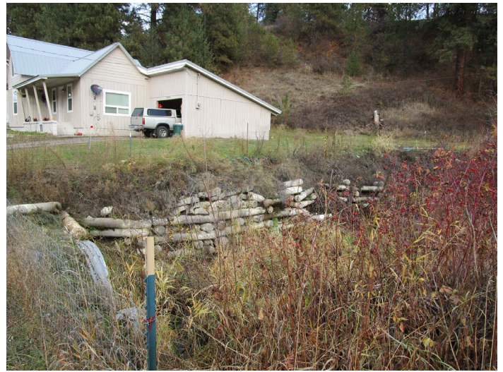
Concrete tubes stabilizing streambank on the lower project area. Bridge replacement and natural soil lifts will improve stabilization of the bank and allow vegetation to grow.
