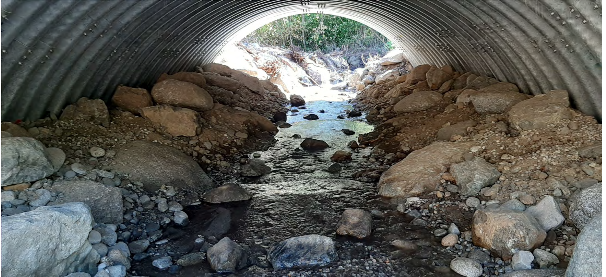
14. (detail) Looking downstream from inlet at constructed streambed in structure (pre-construction not depicted)
