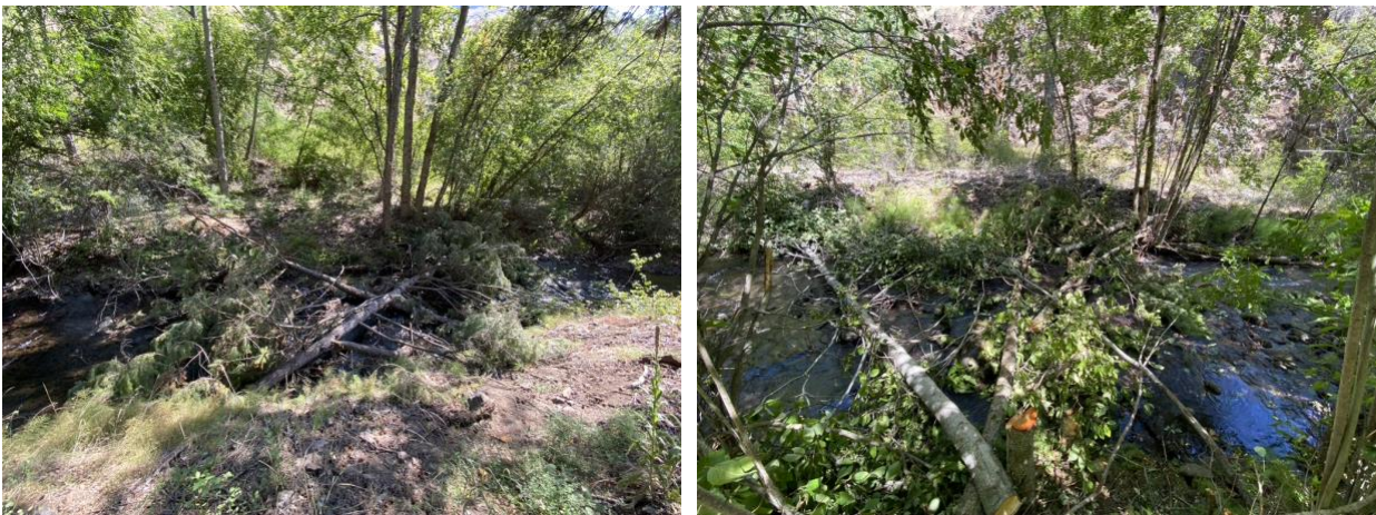
Figure 11. Example of structures enhanced with the addition tree falling (left - South Fork structure #679, right - #157). We felled mostly subdominant Douglas-fir and alder along the stream channel to maintain shading and cover.
