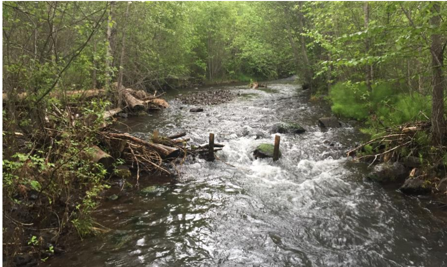
Figure 3. Example of a partly intact post-assisted log structure that were enhanced with the addition of more large woody debris.
