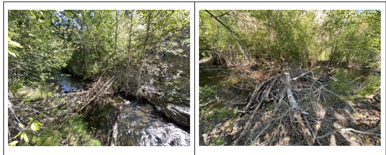
Figure 9. Example of structures enhanced with the addition of large woody debris (left – South Fork structure #124 , right – South Fork # 672). Most of the wood was collected on the Umatilla Forest and donated by the USFS but occasionally we collected trees cut down along the road by road maintenance crews.
