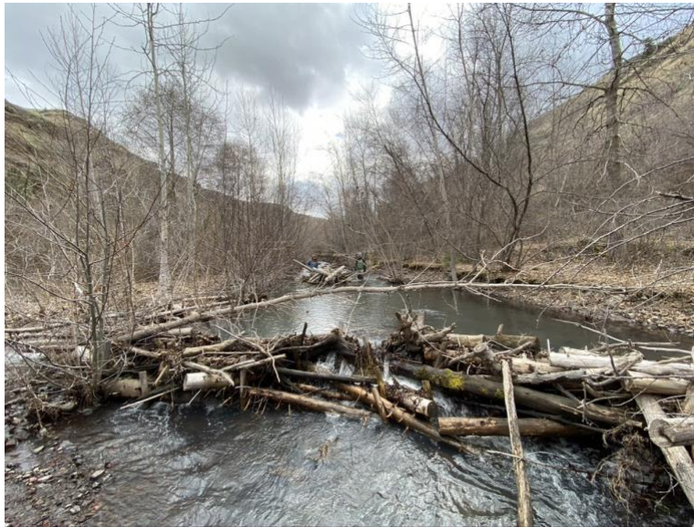
Figure 12. Post-restoration conditions in South Fork Asotin Creek – channel spanning post-assisted log structure forcing overbank flow (during receding high flow) and ponding water upstream of the structure.
