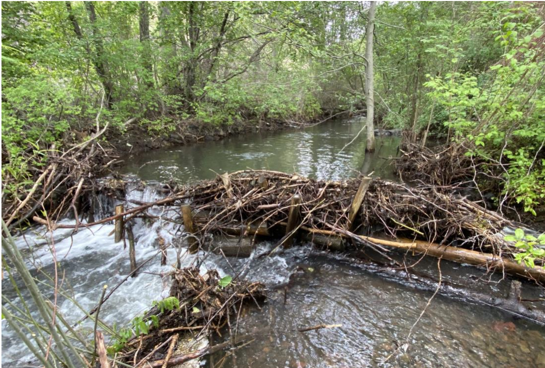
Figure 6. Example of hydraulic and geomorphic diversity created by a channel spanning PALS on South Fork Asotin Creek. A large dam pool was created upstream, a plunge pool and gravel bar formed downstream, and overbank flow is being forced, connecting a portion of floodplain.
