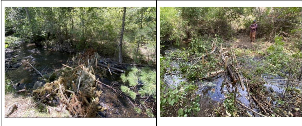
Figure 10. Example of structures enhanced with the addition of posts and large woody debris (left – South Fork structure #42, right - Charley #61) . A hydraulic post driver was used to drive posts into streambed and secure wood. Most of the wood was collected on the Umatilla Forest and donated by the USFS.
