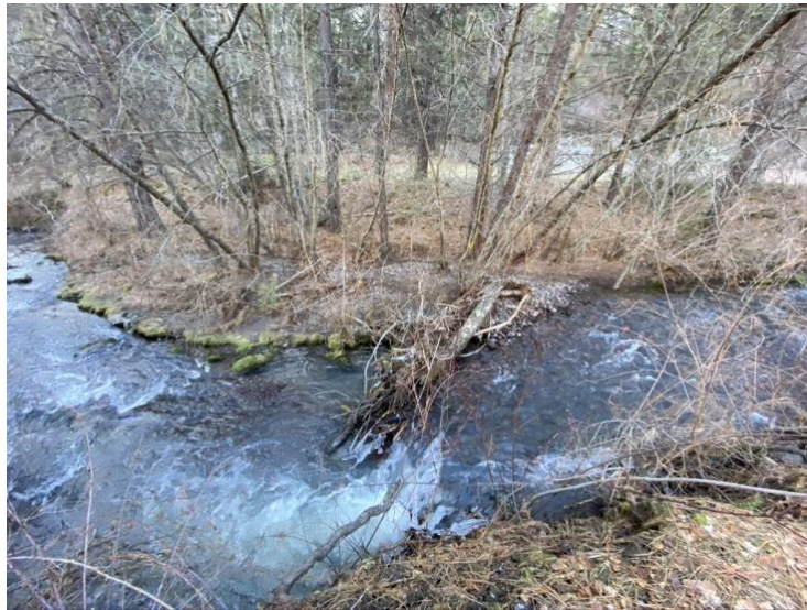
Figure 13. Post -restoration conditions in Charley Creek – bank attached post-assisted log structure forcing flow against river left bank, creating eddy pool downstream, and forcing overbank flow and forming upstream and downstream bars on river right.
