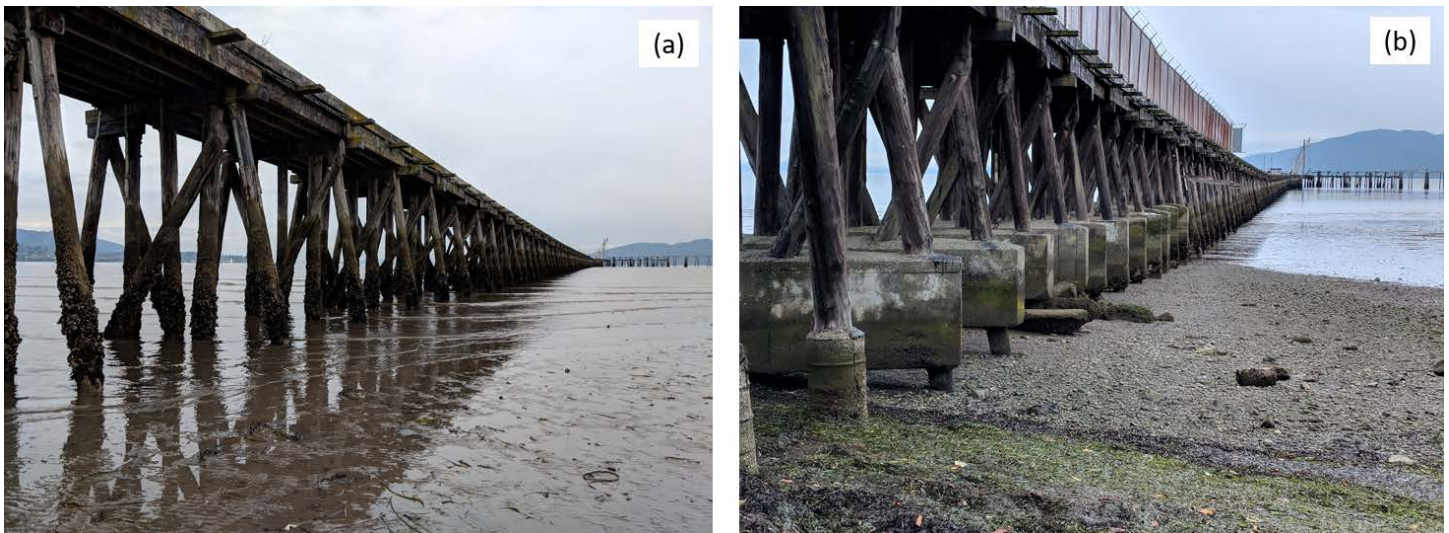
Figure 1: Squalicum Pier consists of a timber deck supported by structural piles. Photos taken by a M&N coastal engineer on Oct 5, 2018 show (a) pile density, looking southwest and (b) concrete footing encasing the first few rows of structural piles, looking southwest.
