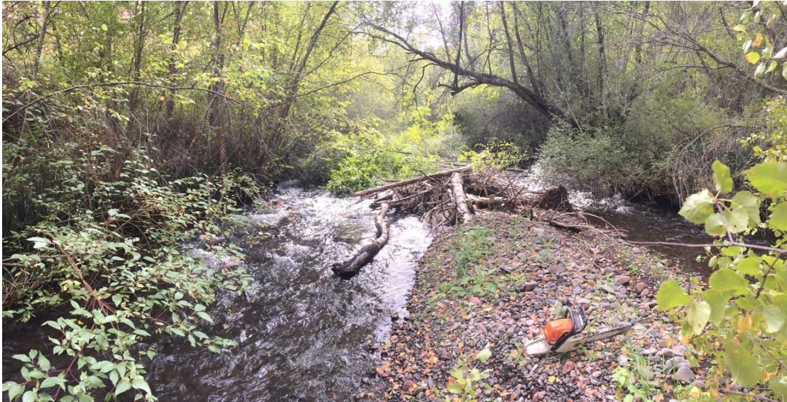
Figure 12. Post -restoration conditions in North Fork Asotin Creek – mid-channel post assisted log structure splitting flow and creating downstream mid-channel bar.
