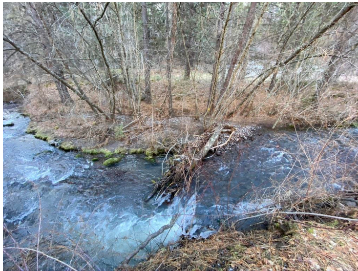
Figure 11. Post -restoration conditions in Charley Creek – bank attached post-assisted log structure forcing flow against river left bank, creating eddy pool downstream, and forcing overbank flow and forming upstream and downstream bars on river right.
