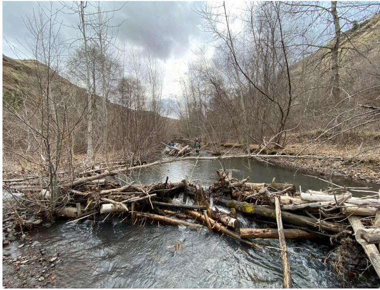
Figure 10. Post-restoration conditions in South Fork Asotin Creek – channel spanning post-assisted log structure forcing overbank flow (during receding high flow) and ponding water upstream of the structure.
