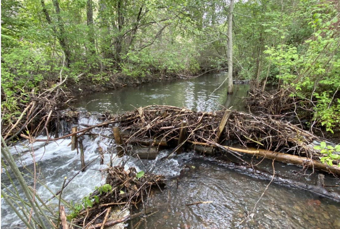
Figure 7. Example of hydraulic and geomorphic diversity created by a channel spanning PALS on South Fork Asotin Creek. A large dam pool was created upstream, a plunge pool and gravel bar formed downstream, and overbank flow is being forced, connecting a portion of floodplain.
