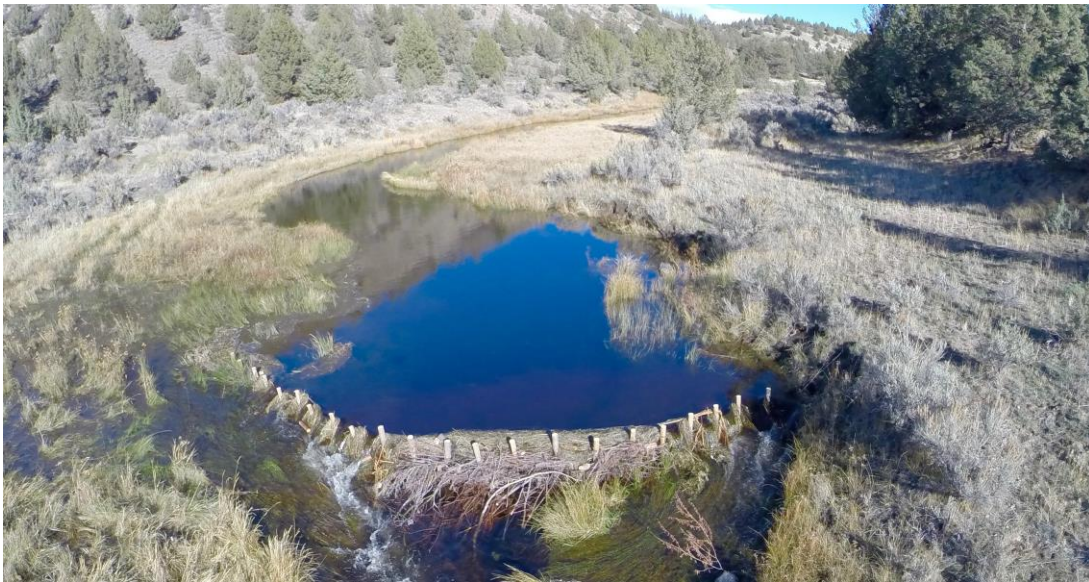
Figure 13. Beaver dam analog on South Fork Crooked River, Oregon forcing overbank flow during low flow.
