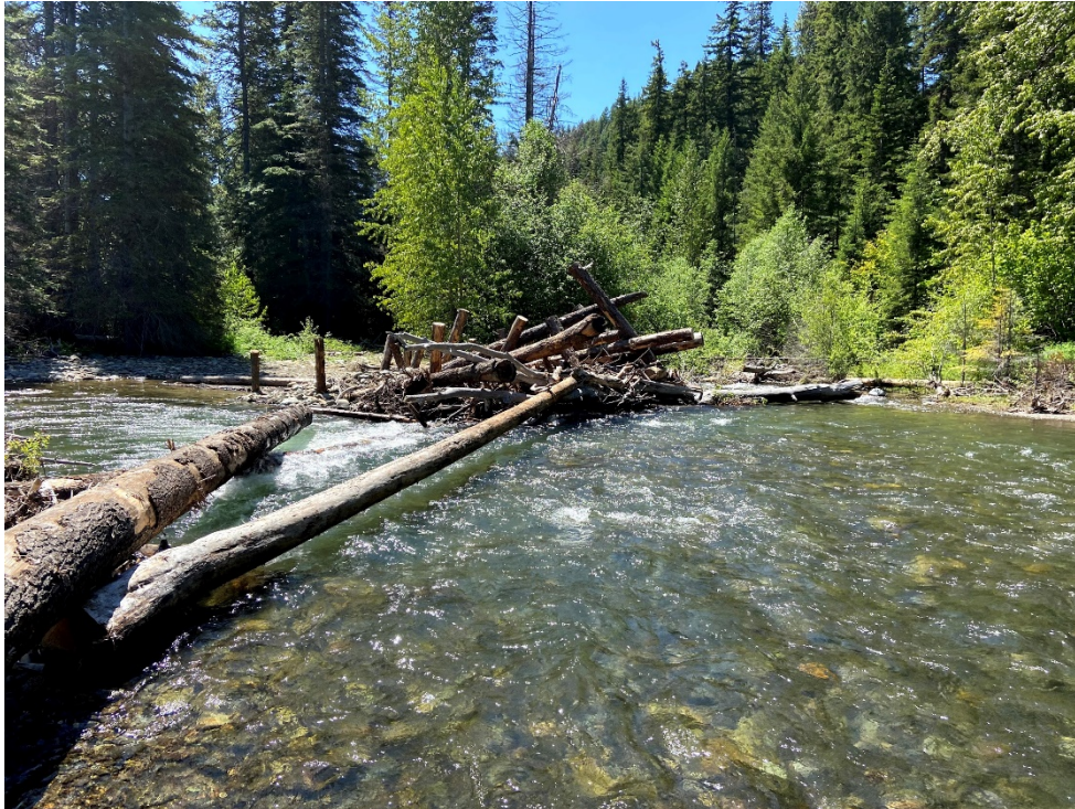
Photo 3 – Wood trapping structure, ballasted with excavated material. Logs across channel were from loose wood placement before a 10-year flood.
