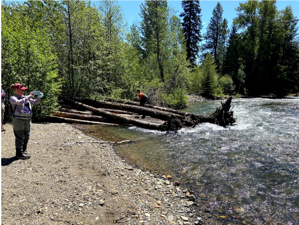
Photo 1 – Example of LWD complexity structure. Logs extend back into trees using weight of rootwads to ballast.
