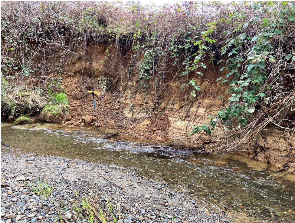
Photo 7 – Cut bank 12-foot-high just downstream of bridge.
