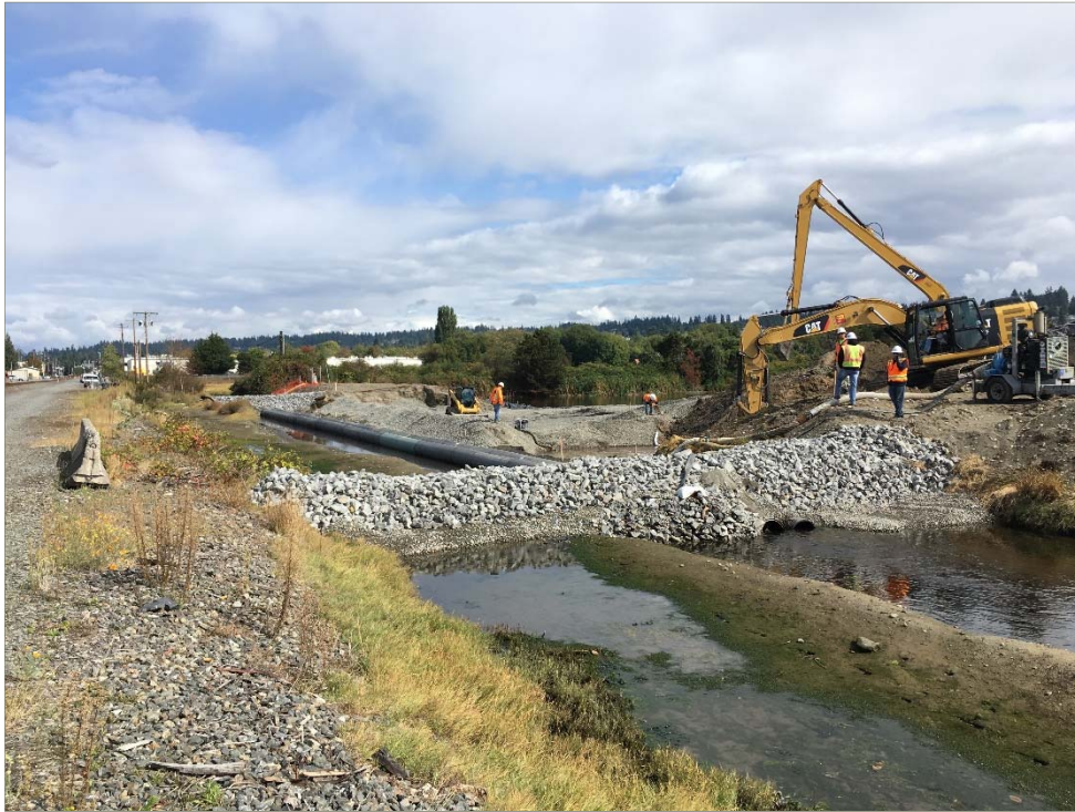
Sample location WC-02. Photo taken September 20, 2017.
