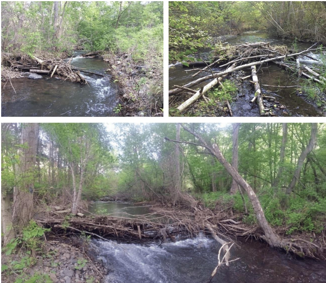
Figure 7. Example of the three post-assisted log structure types (PALS) built in the Asotin Creek IMW. Top left = series of Bank-attached, top right = Mid-channel, and bottom picture = Debris Jam PALS.
