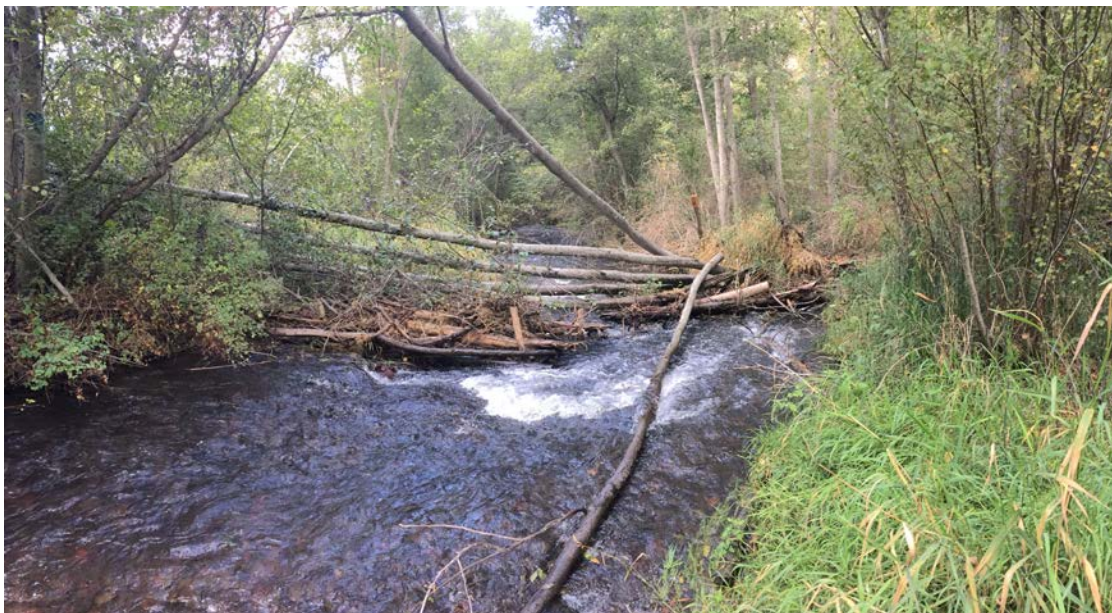
Figure 8. Group of alder trees that have bene recruited into North Fork Asotin Creek as a result of a river left bank-attached post-assisted log structure (PALS) directing flow against the river right bank.
