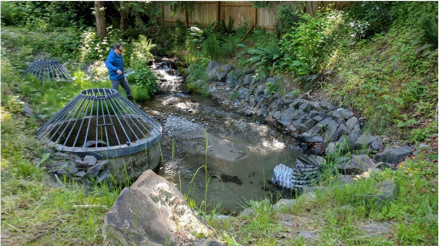
PHOTO 4: In-line sedimentation pond and culvert inlets on east side of E Lake Sammamish Pkwy, on City of Sammamish property. Birdcages on left are entrances to the high-flow bypass system. Corrugated metal standpipe on right side of pond passes low-flows of George Davis Creek. The pond in this photo has been recently maintained, with excess sediment removed.
