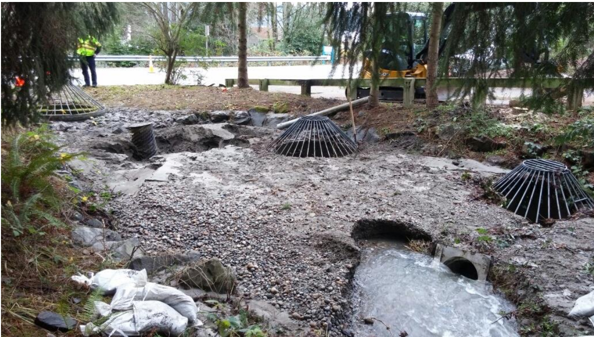
PHOTO 5: Same in-line sedimentation pond and culvert inlets on east side of E Lake Sammamish Pkwy. A landslide upcreek overwhelmed the sedimentation pond, and 100% of the creek is flowing into the high-flow bypass system.
