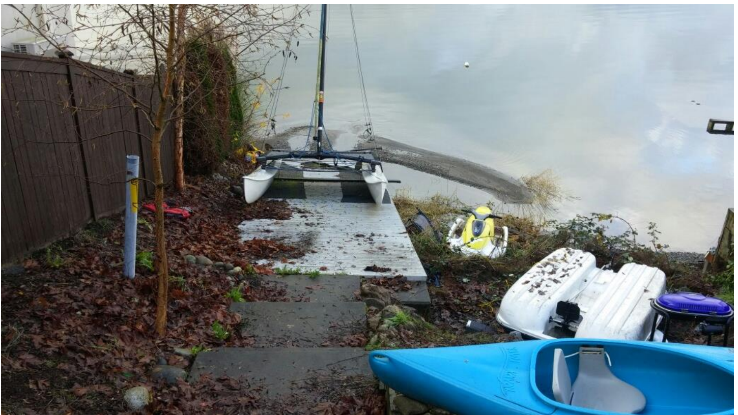
PHOTO 5: Outlet for high-flow bypass is under the boat ramp. This area becomes choked with sediment after storms, impacting adjacent private property.
