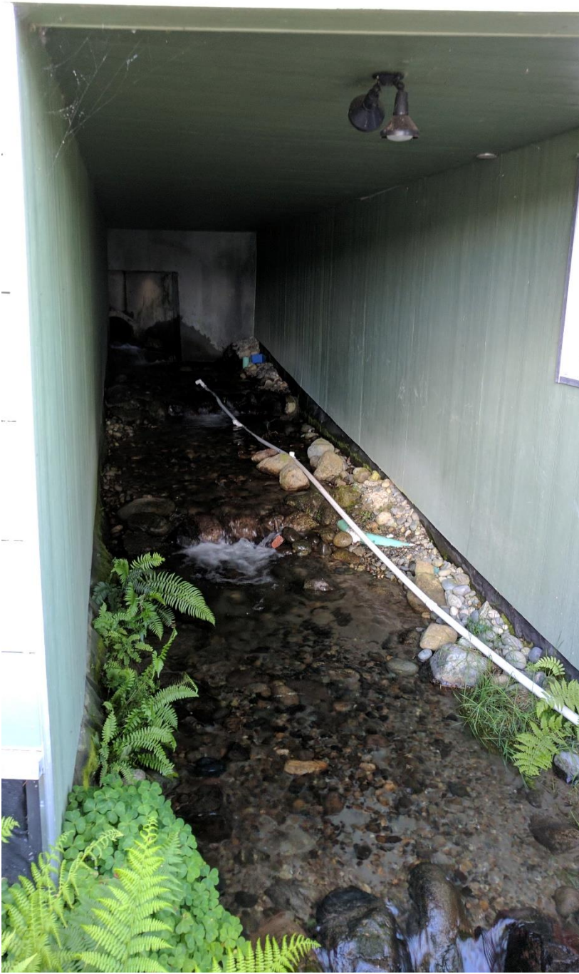
PHOTO 1: Culvert outlet on private property, under a house. This is the first of three barriers between the creek mouth and the east side of East Lake Sammamish Parkway, and is shown as Fish Barrier #1 on the Vicinity Map. This barrier will be abandoned and replaced with a new, open-stream channel on the adjacent property to the north.
