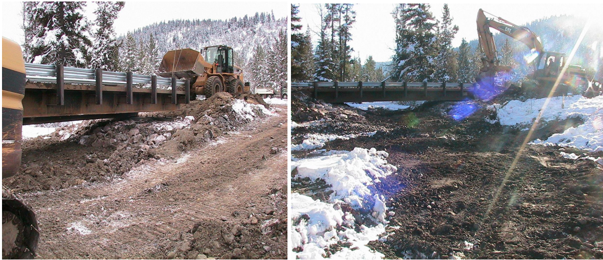
Figure 11a. The modular steel bridge on a similar project in Idaho. Pre-cast concrete abutments are set in the “dry”. Standard heavy equipment sets the modular steel superstructure on the abutments.
