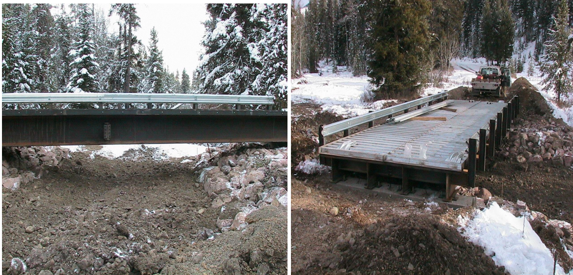
Figure 11b. Modular Steel Bridge
