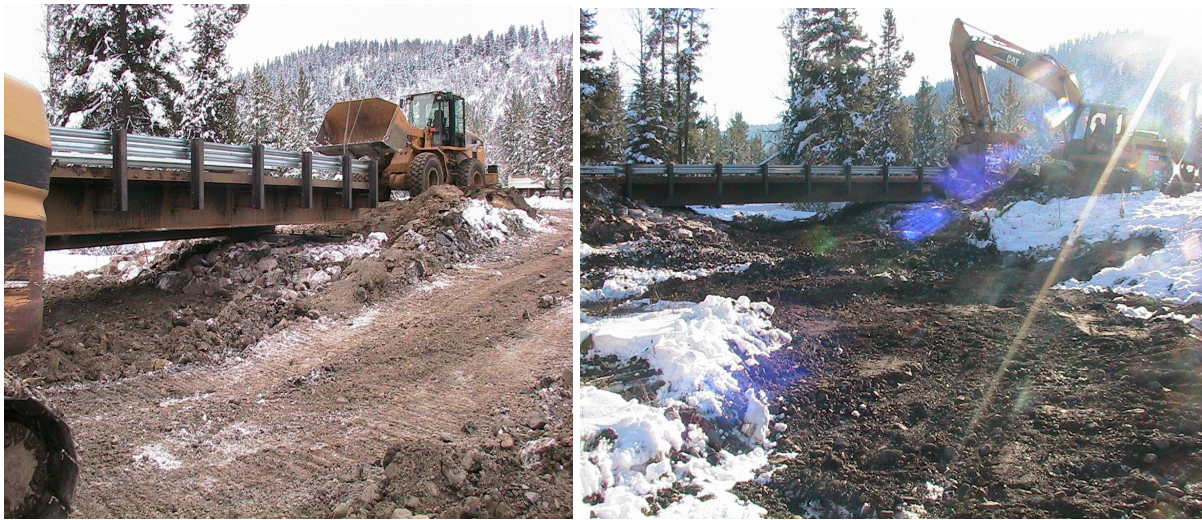
Figure 3a. The modular steel bridge on a similar project in Idaho. Pre-cast concrete abutments are set in the “dry”. Standard heavy equipment sets the modular steel superstructure on the abutments.
