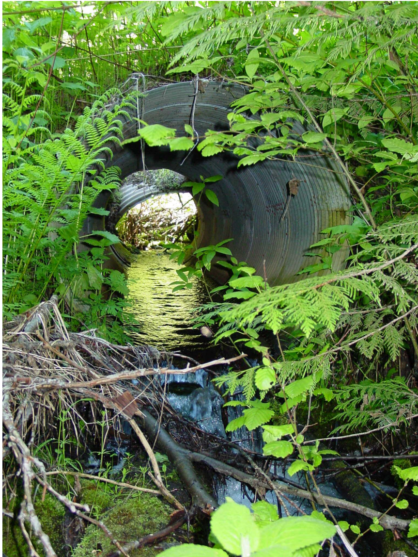
Figure 9. Clear Creek #3 (Note pipe failure)
