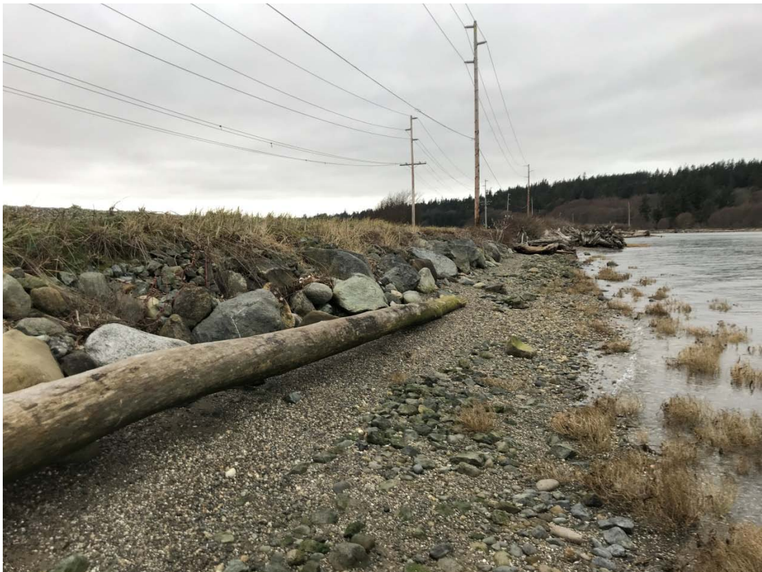
Figure 4: View of woody debris on the shore and rip rap along the base of the dike.
