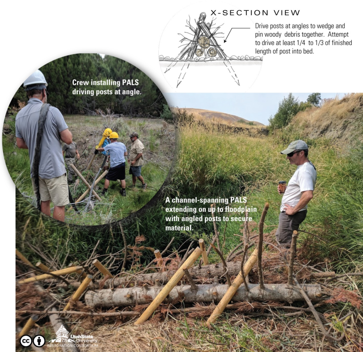
Figure 28 – Installing posts at an angle (as opposed to plumb or vertical) is a helpful way to wedge woody material together and keep it from rafting up and floating away in high flows. It is also physically easier to install because the post-driver does not have to be lifted and held as high above the ground.
