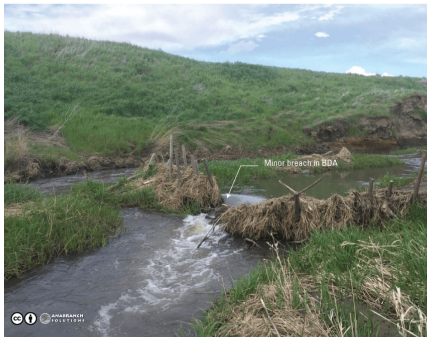
Figure 17 –Example of a beaver dam analogue (BDA) that needs maintenance if the goal is to build a large pond upstream of the structure. The BDA has been partially breached in the center and would need more posts and wood material to function fully. Note this BDA could also use a better mattress on the downstream side of the BDA to reduce the potential for water undercutting the structure.
