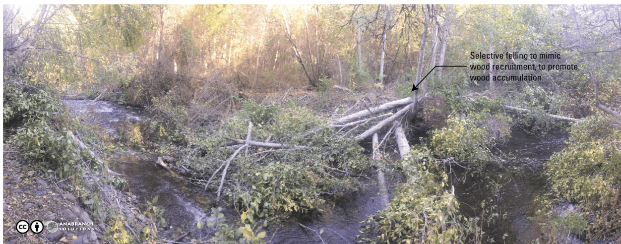
Figure 15 - Maintenance in a high-density large woody debris treatment section where alder trees were directly felled into the riverscape amongst existing post-assisted log structures.
