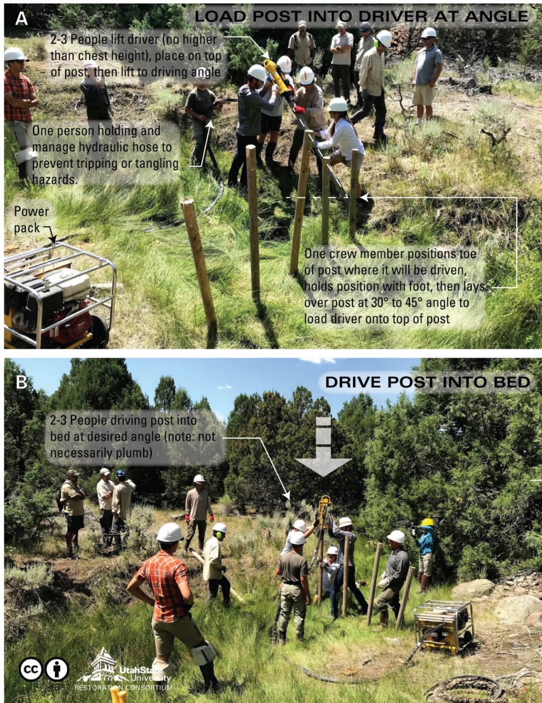
Figure 20 – Best practices for working with a manually operated hydraulic post driver are illustrated above in a small stream.
