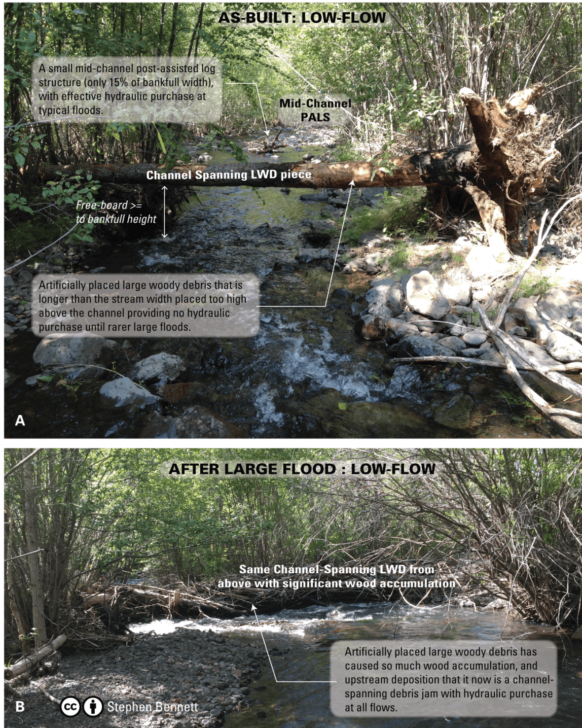
Figure 15 – A key placement consideration is defining at what flow stage the structure will engage with hydraulics or obstruct flows (i.e., hydraulic purchase). At the design stage, there is a choice about whether to build for immediate (i.e., low-flow) hydraulic purchase (e.g., mid-channel PALS in background of A), or only to activate at typical floods or rarer floods (e.g., channel-spanning piece in A). Wood that is long enough that it spans past the entire width of the channel, will only be engaged in overbank flows. Here, there was no wood accumulation for three years through typical floods, but a larger rare flood eventually came through and impressive responses associated with wood accumulation resulted.
