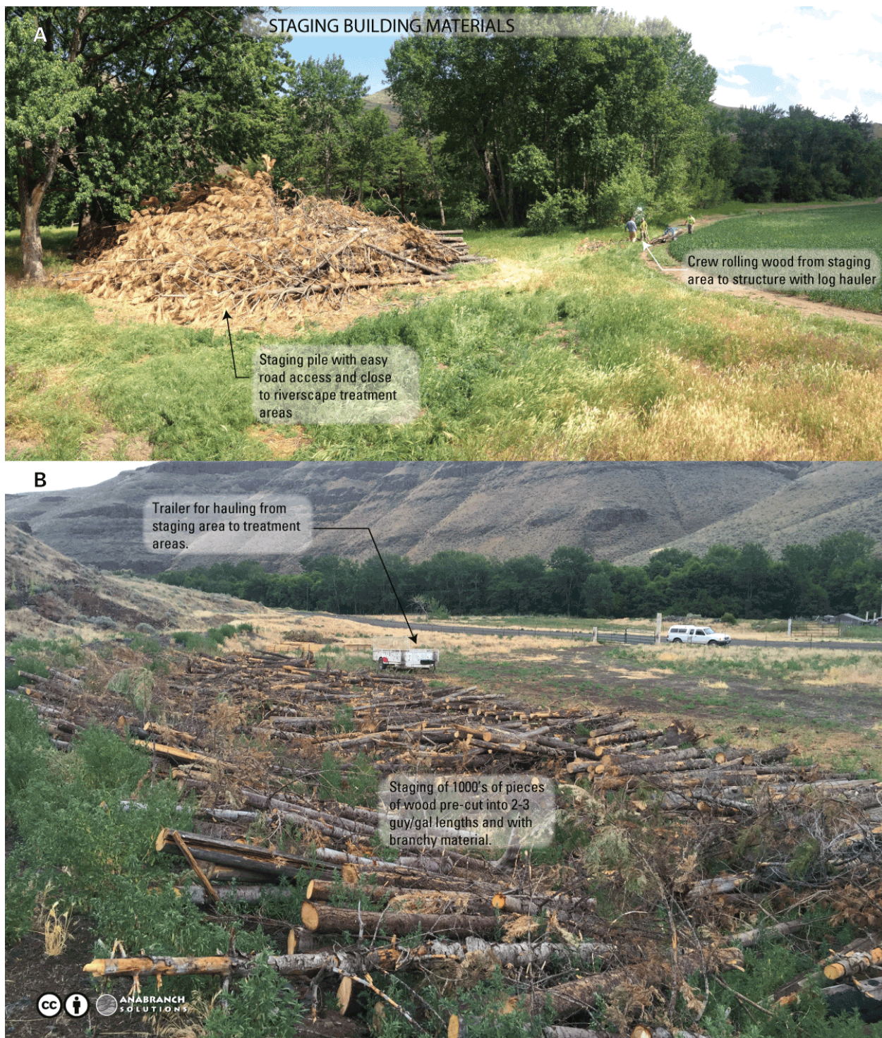
Figure 5 – Staging of woody building materials secured from off site into floodplain (A) and terrace (B) areas with easy access for unloading and loading, and subsequent moving into riverscapes treatment areas.
