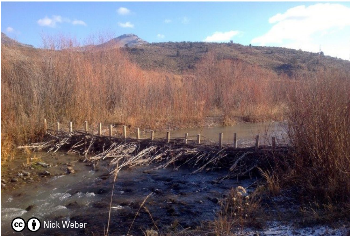
Figure 19 - Early generation BDA. The structure is characterized by a tight willow weave and limited downstream mattress, leaving it more susceptible to scour that can undermine the posts. The downstream mattress shown here was built by beaver, and provided the original inspiration for incorporating mattresses into BDAs which diffuses flows coming over the dam.
