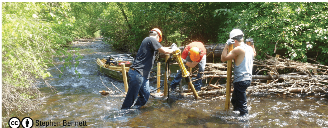
Figure 8 – A crew of three building a post-assisted log structure.
