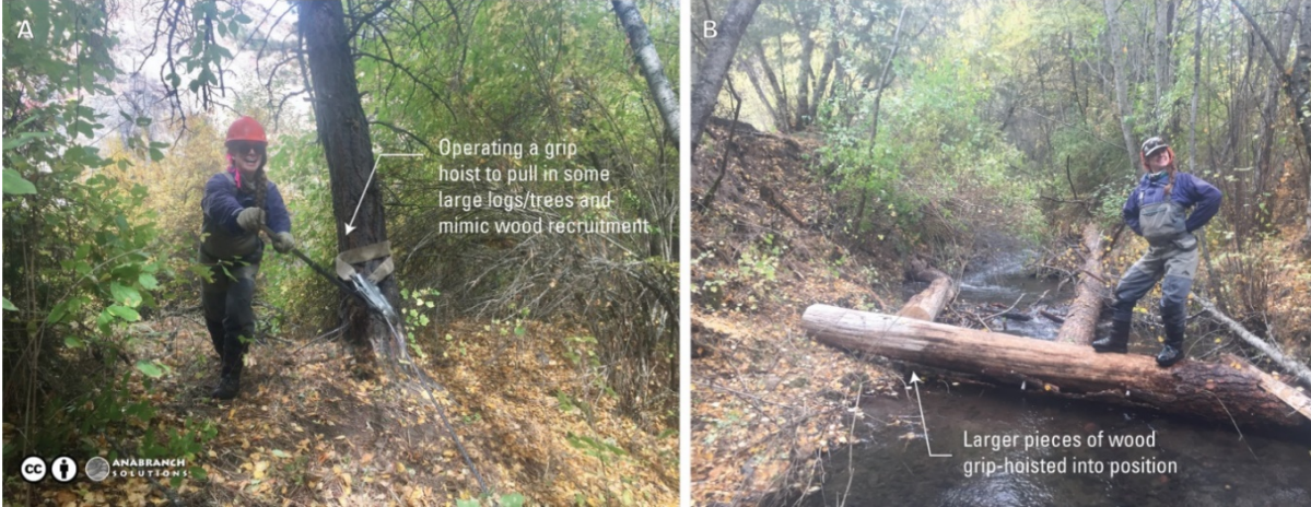
Figure 16 - Example of using a grip hoist to pull in wood into the riverscape (i.e. mimicking process of wood recruitment) to enhance or create a new wood accumulation (structure) in treatment sections as part of ongoing treatments until the processes of wood recruitment and wood accumulation are self-sustaining..
