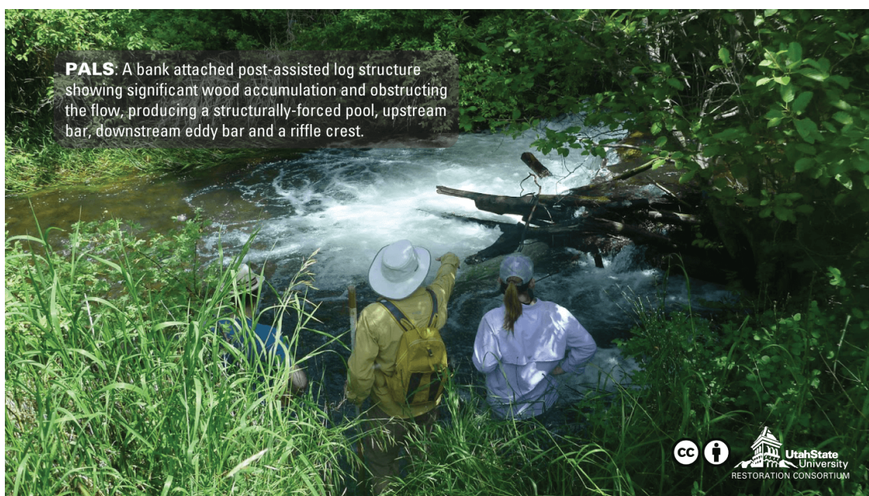
Figure 3 – A post-assisted log structure (PALS) so buried in wood accumulation and sediment, it is hard to recognize.
