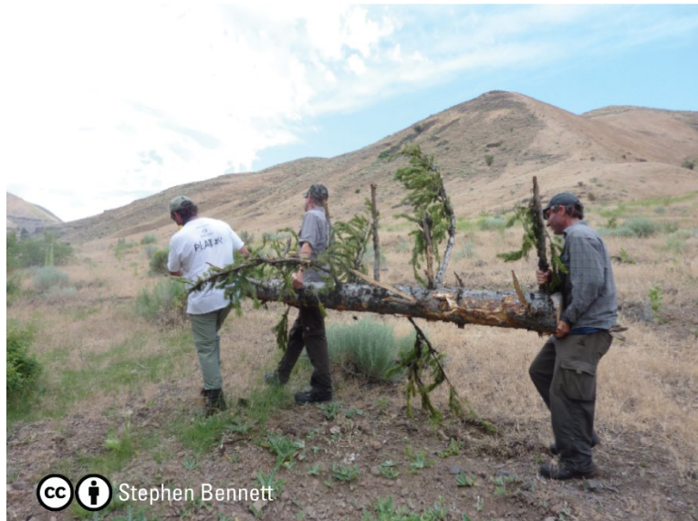
Figure 6 - Most materials will be moved by hand, so it is essential it can be moved by hand. Most of the material you work with is easiest if it is one-guy/gal wood (i.e., it can be carried by one person). The terms 2-guy/gal and 3-guy/gal have real physical meaning. In some cases, 'bigger' wood can be simulated by creatively combining a bunch of smaller pieces together, meaning more can be done by less people. However, after moving enough 2-guy/gal or 3-guy/gal wood, you will want to make sure you use it sparingly and only where necessary. Note limbs removed on underside of log to lie in contact with the stream bed (i.e. increased hydraulic purchase).
