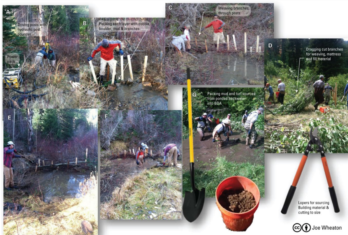
Figure 11 – Example of the construction process of a beaver dam analog including driving posts, and adding woody material, packing in fill material.
