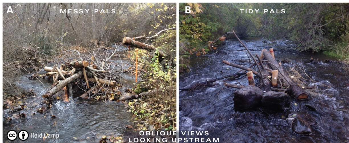
Figure 12 - Example of a ‘messy’ mid-channel post-assisted log structure (PALS) (A) versus a ‘simple’ mid-channel PALS (B). Natural wood accumulations are messier.
