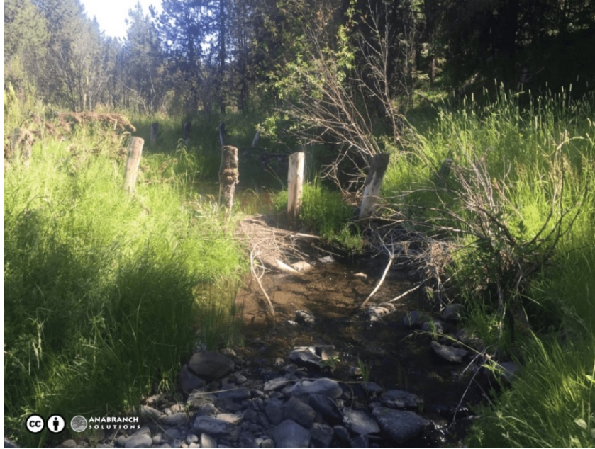
Figure 18 –Example of a beaver dam analogue (BDA) that could have some maintenance to plug it back up. Most of the original ponded area from the BDA has been buried by sediment and there are only the top of the posts left visible. As shown in Figure 19, this would be the point at which the functional lifespan of the structure is over, the process of beaver dam activity is not yet self-sustaining, but it is deemed it could be with additional treatments. This is a good demonstration of how restoration can be staged – by adding more woody material to this structure the system would continue to aggrade and may force more floodplain connection, which may attract and make it easier for beaver to take over the process.
