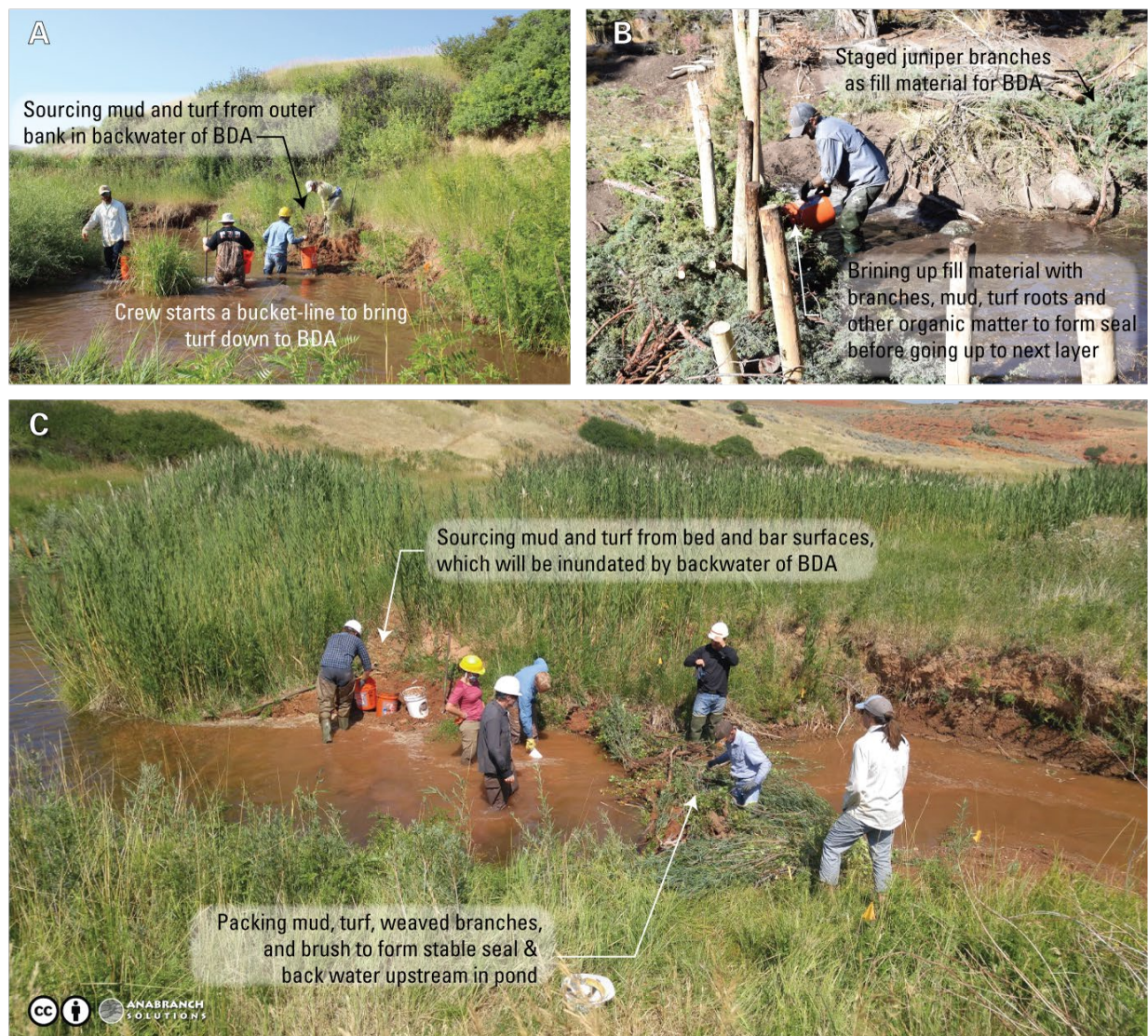
Figure 10 – For BDAs, mud, bed sediment, turf mats, leaves and organic matter are very useful for plugging up leaks and making the BDA hold back water. It is helpful to have lots of 5-gallon buckets, a few shovels and a small crew to get a bucket line from the source area to the crew members packing the dam material.
