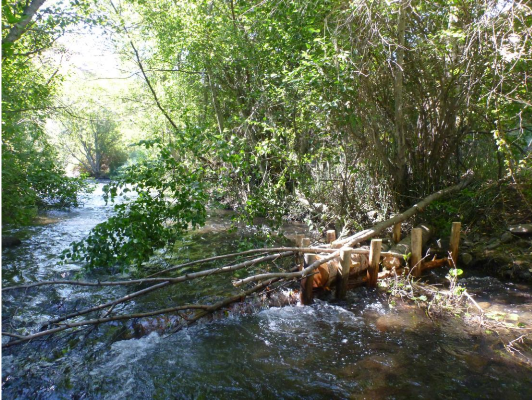
Figure 33. Example of a trial DWS on North Fork Creek (NF-TX1). This is an example of a more complex structure as the posts were driven in an off-set pattern. LWD was then added diagonally between the posts to lock the pieces together. Flow is towards the reader and structure is placed on river left. Note the extensive riparian vegetation, wide and shallow channel, and LWD extended beyond the posts to constrict flow.
