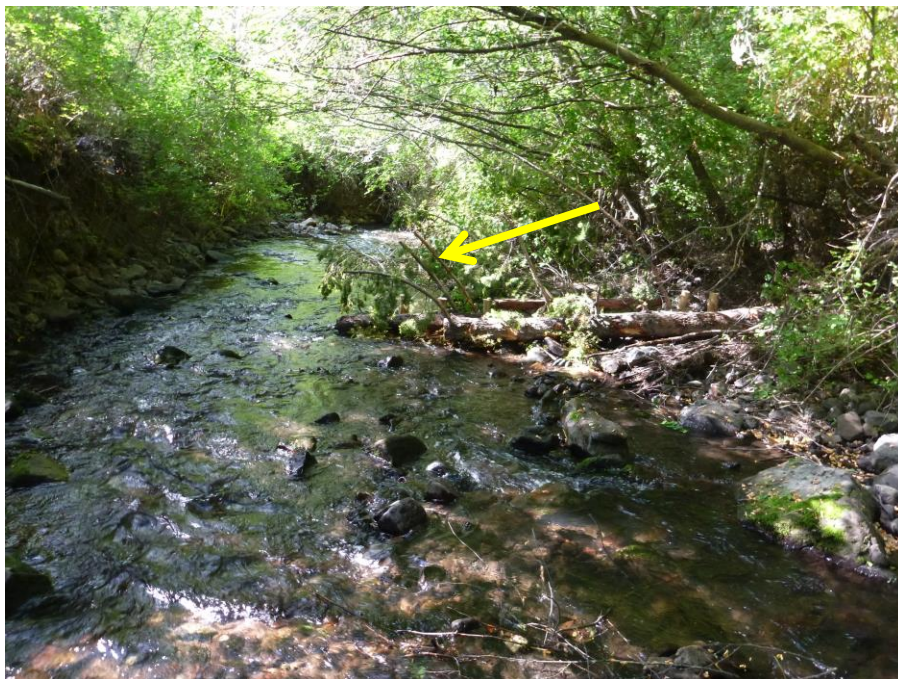
Figure 16. Example of a) the installation of posts and trial structure using a hydraulic post driver and b) the completed structure with LWD added in South Fork Creek trial site TX-2. Yellow arrow indicates location of completed structure. Posts cut to average high flow level after installation.
