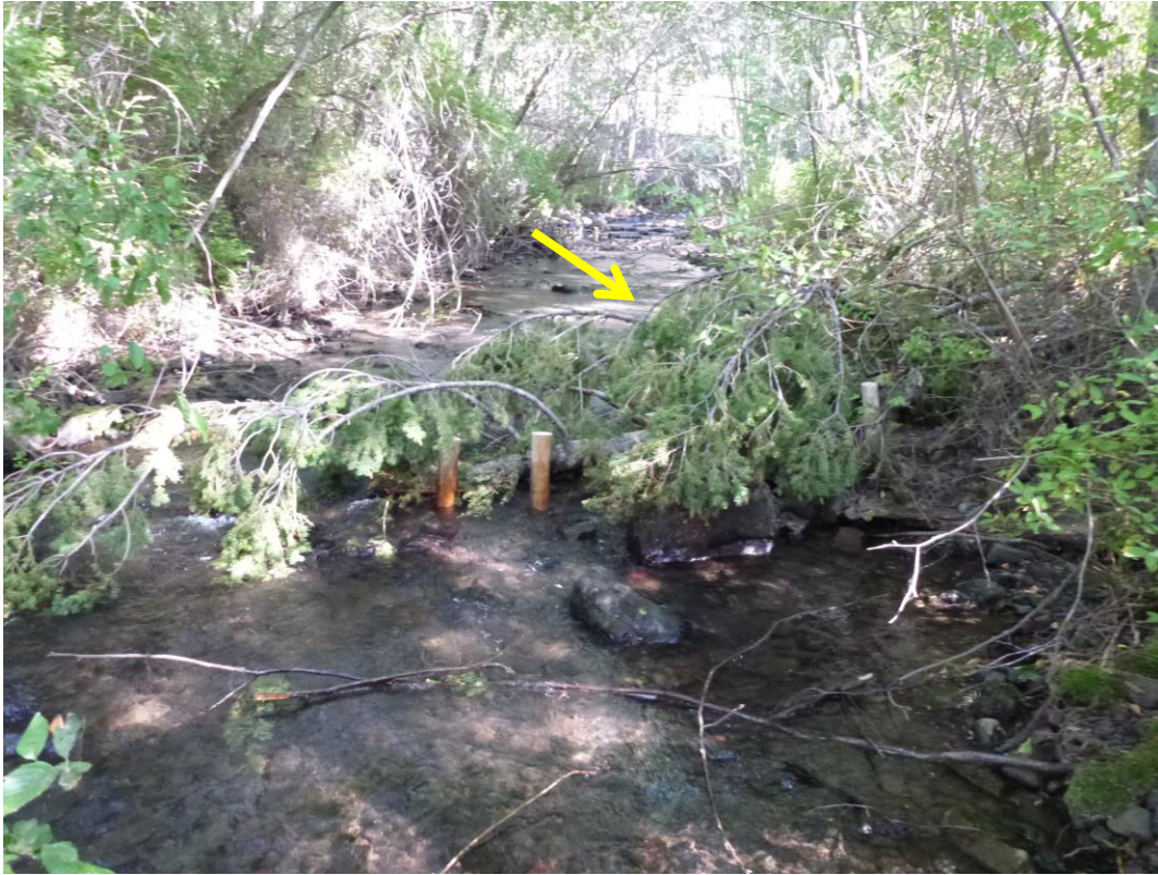
Figure 30. Example of a trial DWS on South Fork Creek (SF-TX3). A green piece of LWD with branches was added to this structure to increase the likelihood it will trap other debris washed downstream. Flow is towards the reader and structure is placed on river left. Note the extensive riparian vegetation, wide and shallow channel, and large substrate of cobble and boulders. Yellow arrow points to SF-TX4 50 m upstream on river right from SF-TX3.
