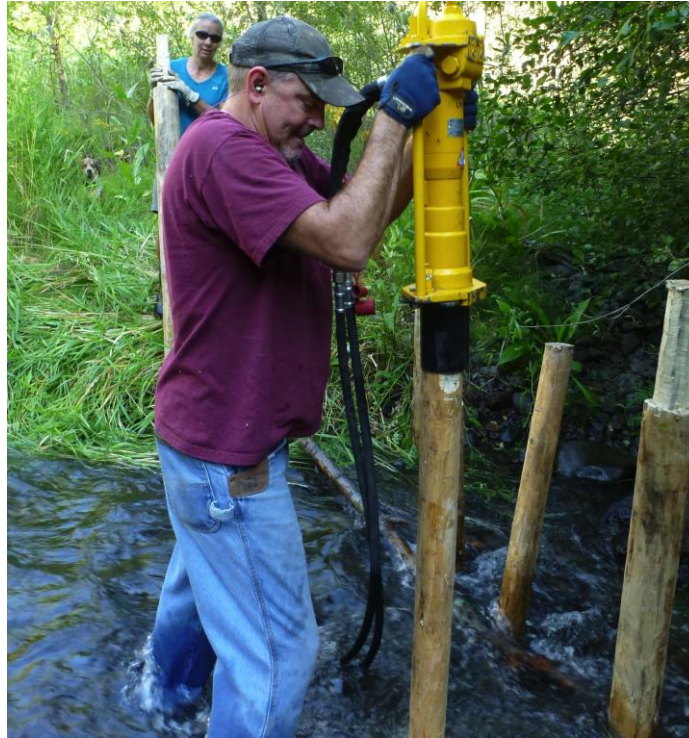
Figure 42. Example of the hydraulic post driver that will be used to install DWS in Asotin Creek.
