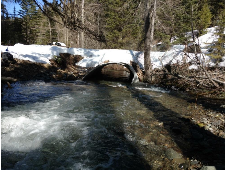
Photo 1 taken upstream looking downstream at the culvert showing the flow constriction under current conditions and deformed shape of the culvert.
