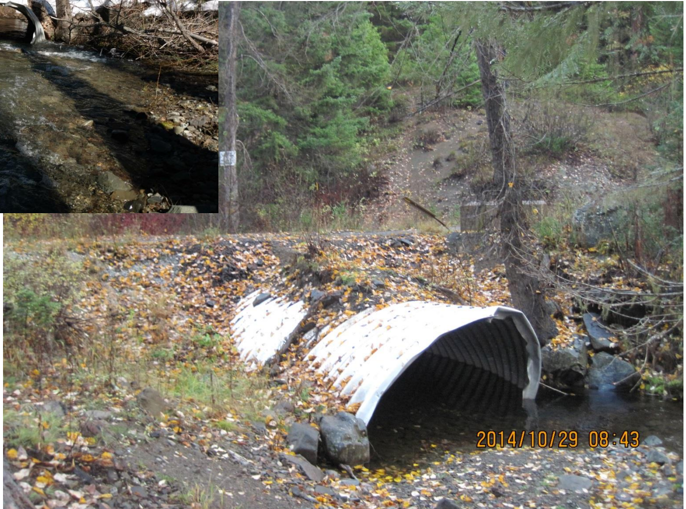
Photo 2 taken under low flow conditions showing the damage to the structure.
