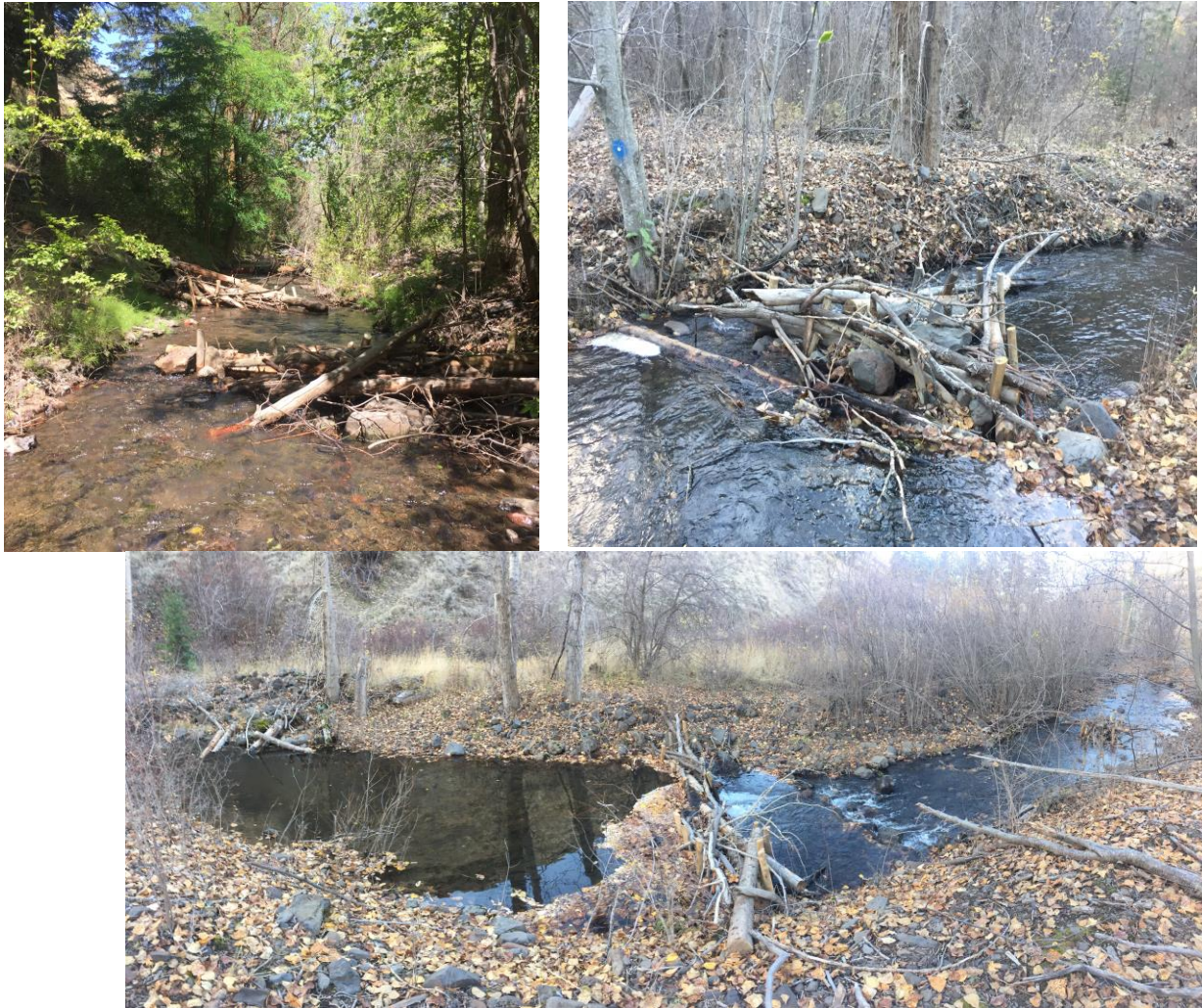
Figure 4. Example of the three most common post-assisted log structure (PALS) built in the new treatment section of the South Fork Asotin Creek in summer of 2016. Top left = series of Bank-attached PALS, top right = Mid-channel PALS, and bottom picture = Debris Jam PALS.
