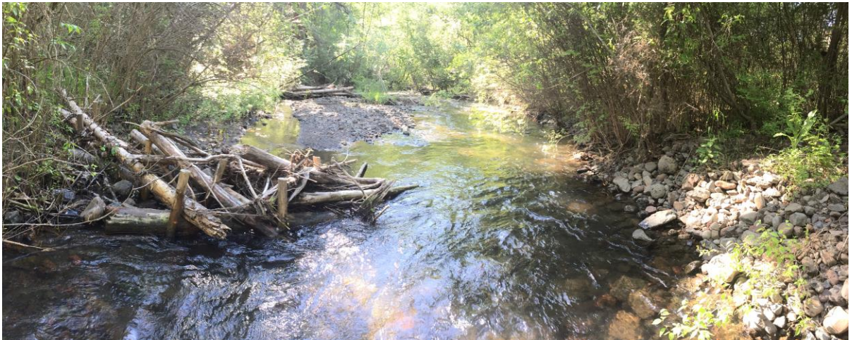
Figure 8. Example of post-assisted log structure built in 2016 in South Fork section 1 creating a large gravel and cobble bar downstream of the structure.
