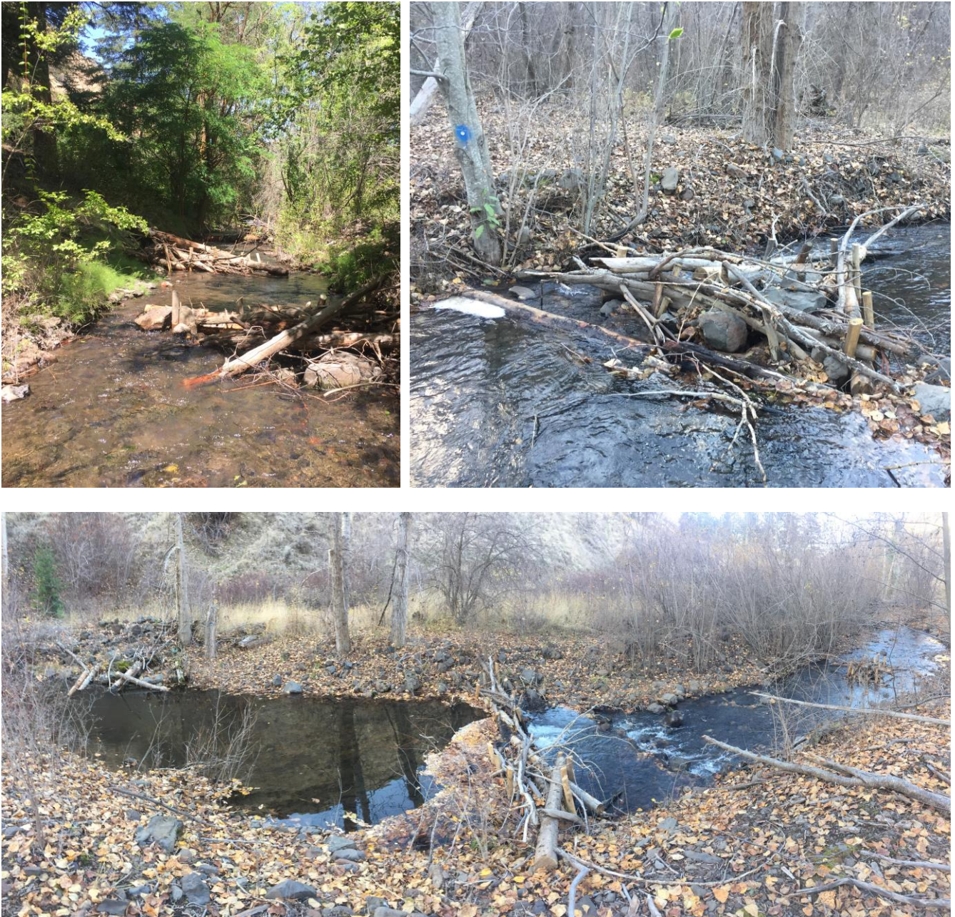
Figure 3. Example of the three most common post-assisted log structure (PALS) built in the new treatment section of the South Fork Asotin Creek in summer of 2016. Top left = series of Bank-attached PALS, top right = Mid-channel PALS, and bottom picture = Debris Jam PALS.
