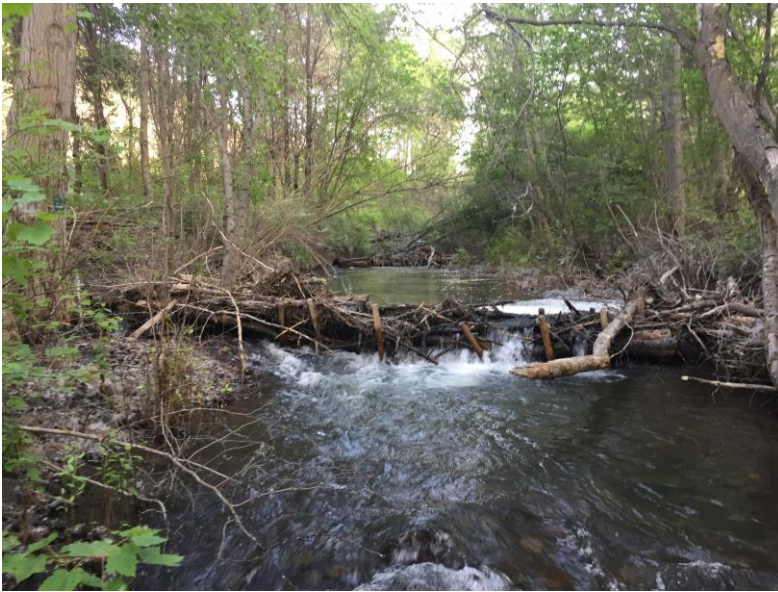
Figure 7. a) Debris jam built in 2016 and viewed in summer of 2017. Note large dam pool upstream. b) Upstream of debris jam large sediment deposit covered with cottonwood seeds.
