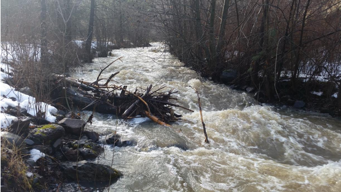
Figure 4. South Fork Asotin Creek, bank-deflector PALS during high flows: spring 2017.
