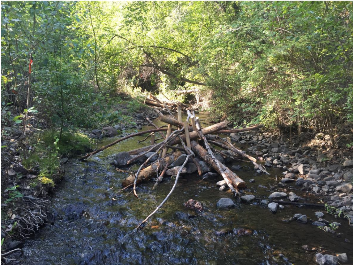
Figure 4. Example of post-assisted log structure (PALS) built in the new treatment section of the South Fork Asotin Creek in summer of 2016. Bank-attached PALS in background and Mid-channel PALS in the foreground.
