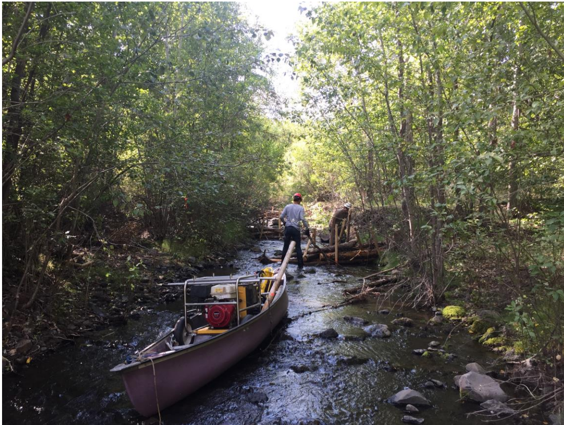
Figure 3. Example of post-assisted log structure (PALS) being built in the new treatment section of the South Fork Asotin Creek in summer of 2016.
