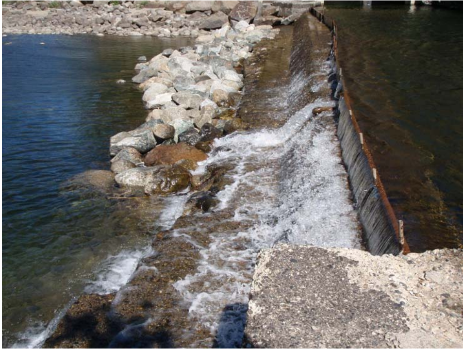
Figure 12 – Diversion Dam on Icicle Creek at low flow. Flashboards are 12” high.
