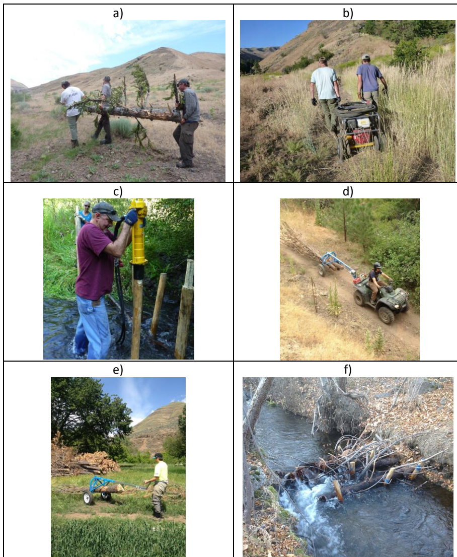
Figure 23. Example of the a) average size of LWD, b) hydraulic post driver that is used to install posts, c) installation of a post with the driver, d) transport of LWD with ATV, e) transport of LWD with log hauler, and f) completed bank attached post-assisted log structure (PALS).
