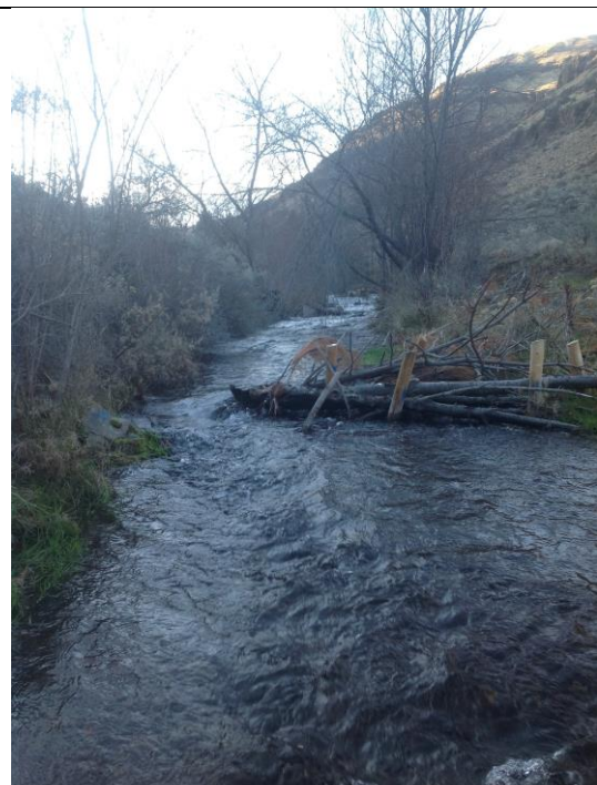
Deflector structure Charley Creek
