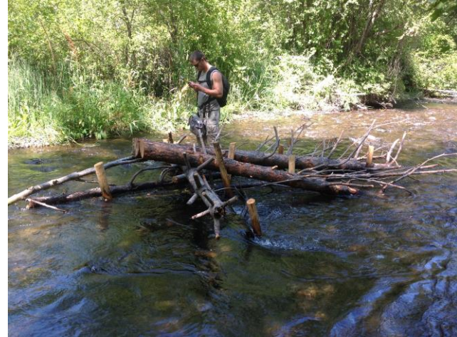
Mid-channel structure North Fork Asotin Creek
