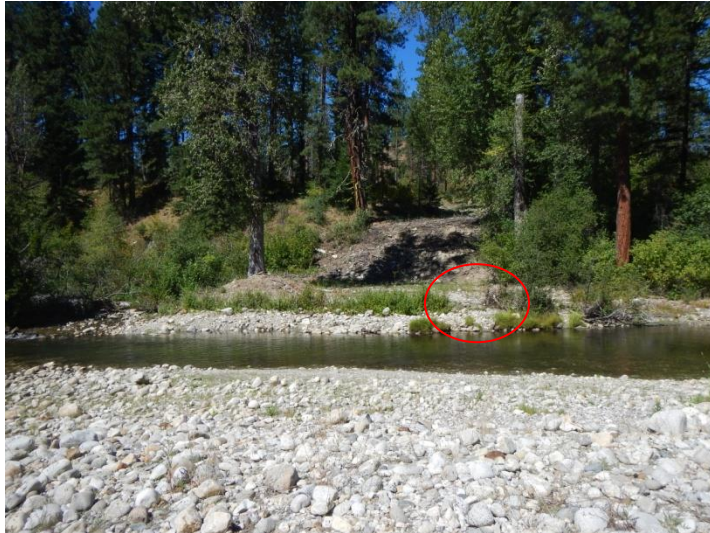
Figure 21. Breach in brush mattress circled in red.
