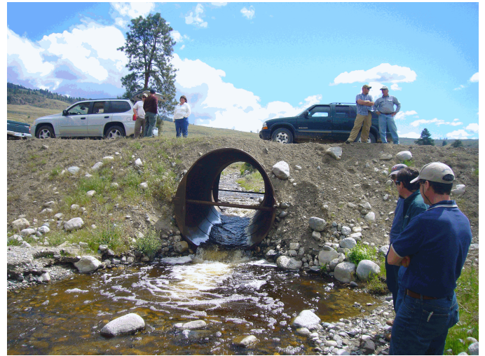
Trout Unlimited Inc.; Ninemile Creek Riparian Restoration (#12-1648), , 05/23/2012, Attachment #151173, Road Crossing Barrier to be Corrected, Pre-Work
