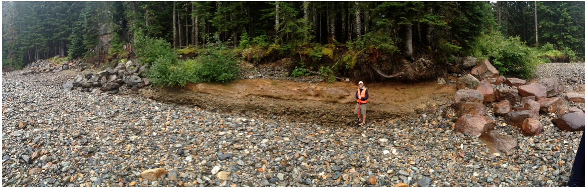
FIGURE 6 – Bank protection installed between RM 1.35 to 1.45
