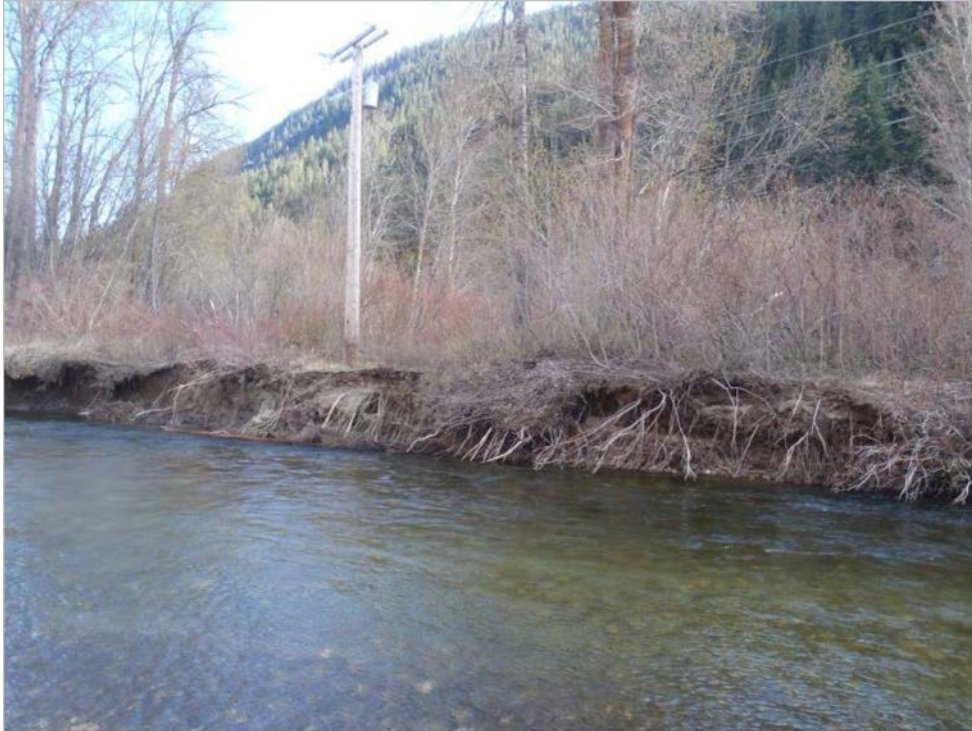
Figure 12. Power pole threatened by streambank erosion near RM 13
