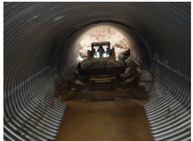
Contractor installing Engineered Streambed Material and Rock Bands.
