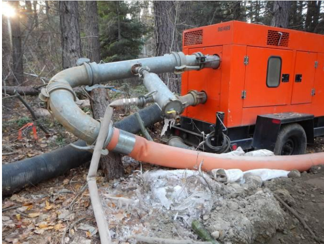
Stream bypass pump operated non-stop.
