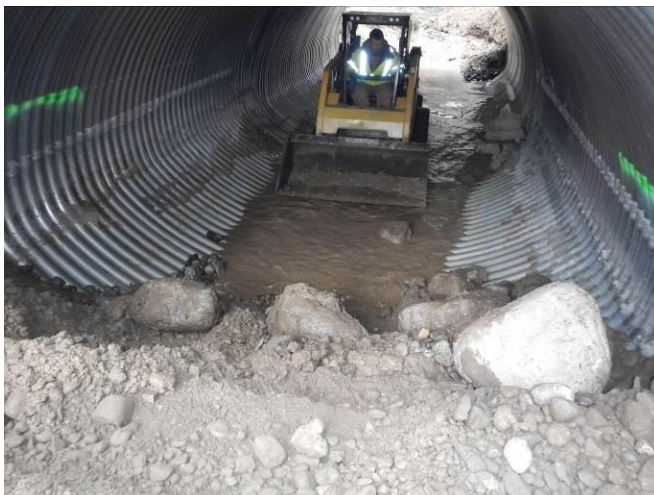
Contractor installing Engineered Streambed Material and Rock Bands.
