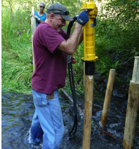
Figure 14. Example of the hydraulic post driver that is used to install large woody debris structures in Asotin Creek.
