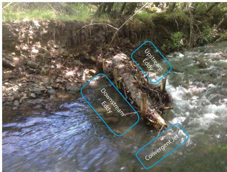
Figure 23. An example of hydraulic responses that significantly increased at restoration structures on the South Fork of Asotin Creek and Charley Creek since restoration (note flow direction is from right to left).
