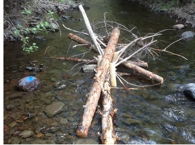
Mid-channel structure South Fork Asotin Creek
