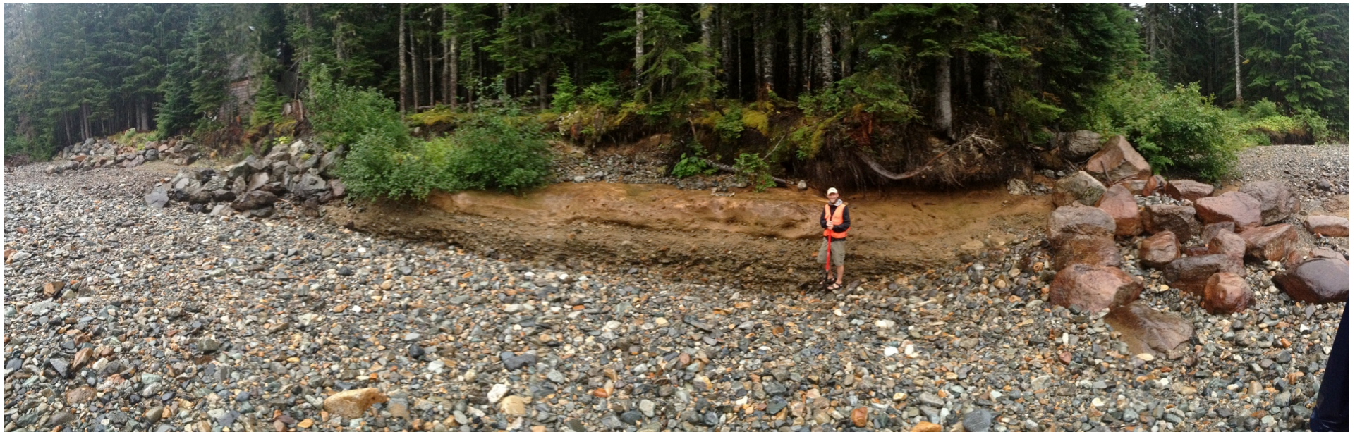
FIGURE 6 – Bank protection installed between RM 1.35 to 1.45
