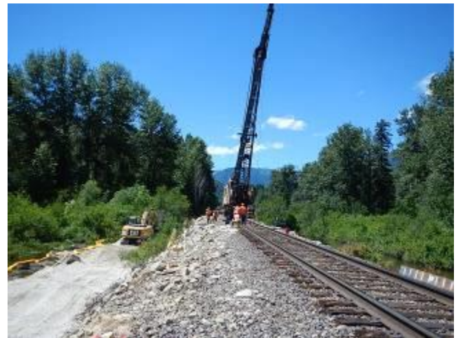
BNSF stockpiled “H” piles at bridge location. BNSF crew using track mounted pile driver to drive “H” piles.
