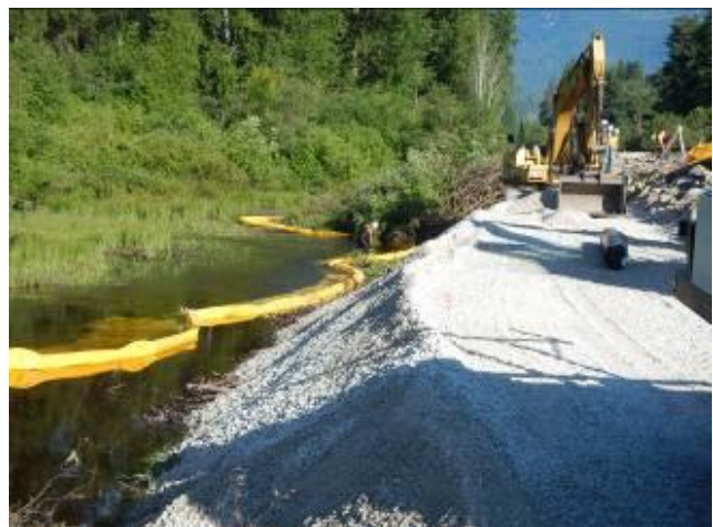
Hurst crew installing turbidity curtain to isolate the construction site from Nason Creek.
