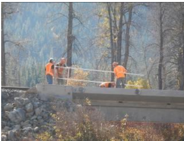
Hurst crew removing sandbag cofferdam BNSF crew installing handrail on new bridge
