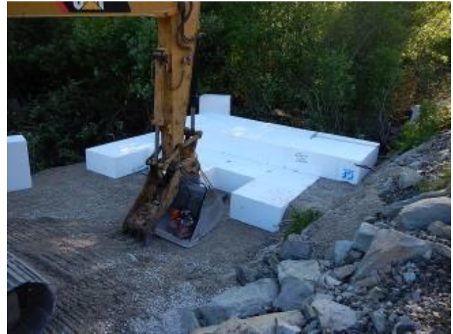
Construction of the access road required installation of geo-foam blocks adjacent to the bridge.
