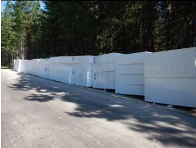
Construction of the access road required installation of geo-foam blocks adjacent to the bridge.
