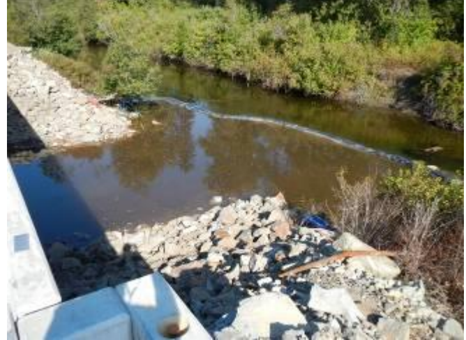
Excavation under the new railroad bridge required construction of a cofferdam isolating the work zone from Nason Creek.
