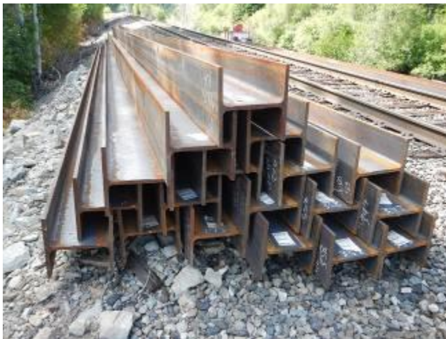
BNSF stockpiled “H” piles at bridge location. BNSF crew using track mounted pile driver to drive “H” piles.
