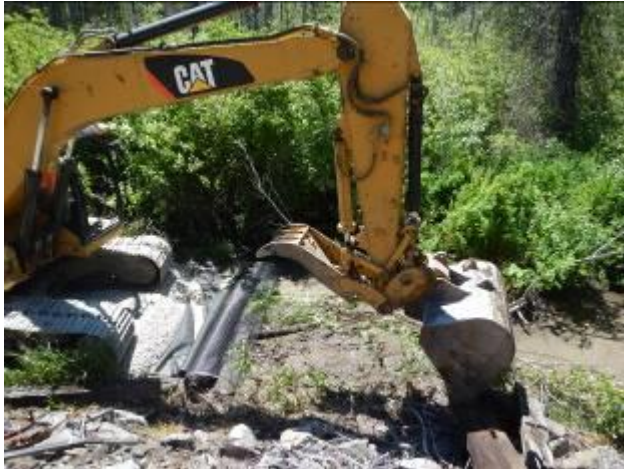
Hurst clearing vegetation and installing geo-grid as base for the access road.
