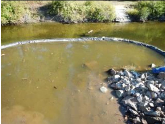
Excavation under the new railroad bridge required construction of a cofferdam isolating the work zone from Nason Creek.
