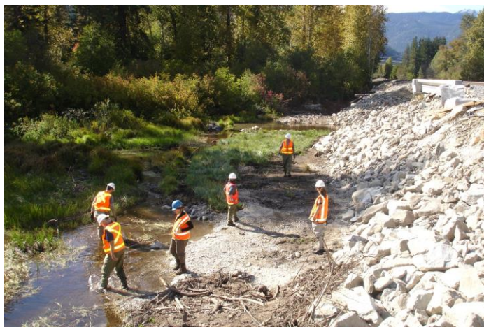
Chelan County and ICF staff complete sedge matt installation and final planting
