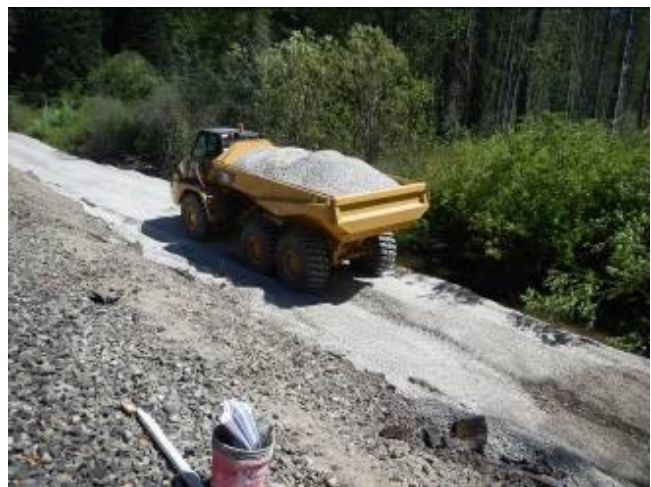
Hurst utilizes 30 Cubic Yard off road hauler to place road ballast material.
