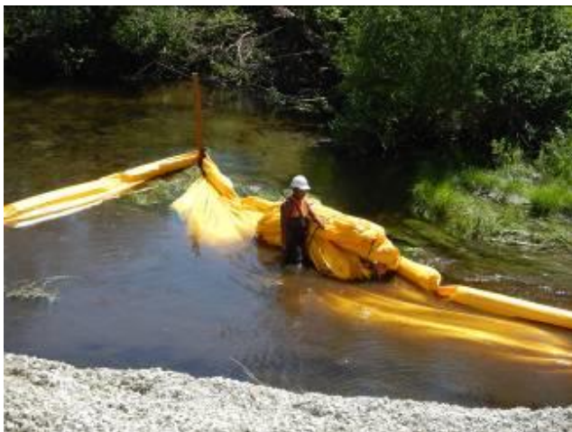
Hurst crew installing turbidity curtain to isolate the construction site from Nason Creek.
