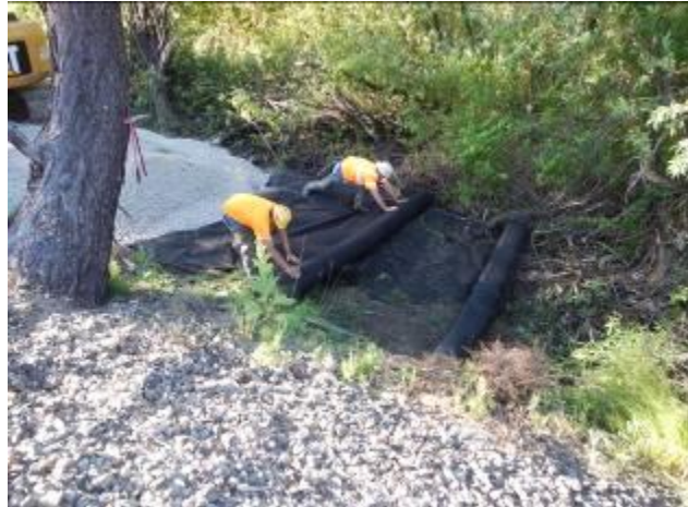
Hurst clearing vegetation and installing geo-grid as base for the access road.
