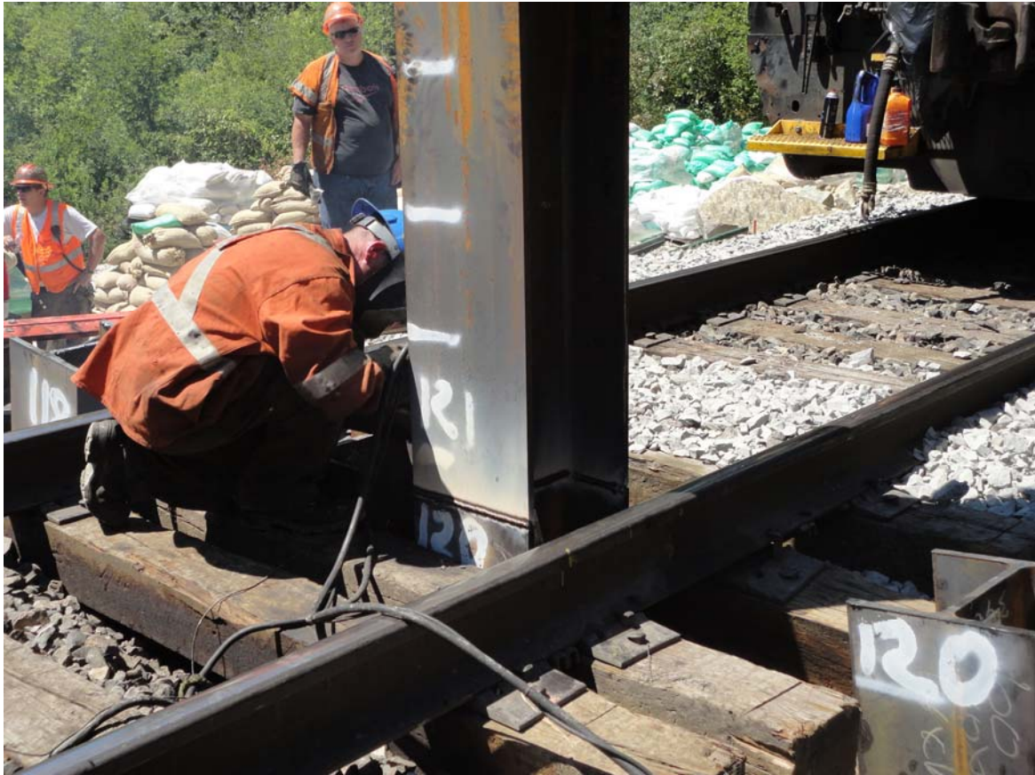
Photo 1: View of Bent 2 Pile 3 Segments 2 and 3 being welded together.
