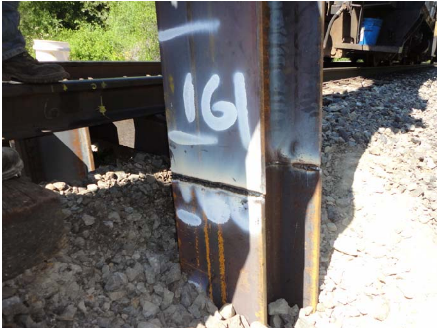
Photo 1: View of the weld on Pier 3 Pile 4 at 160 feet, between segments 3 and 4.
