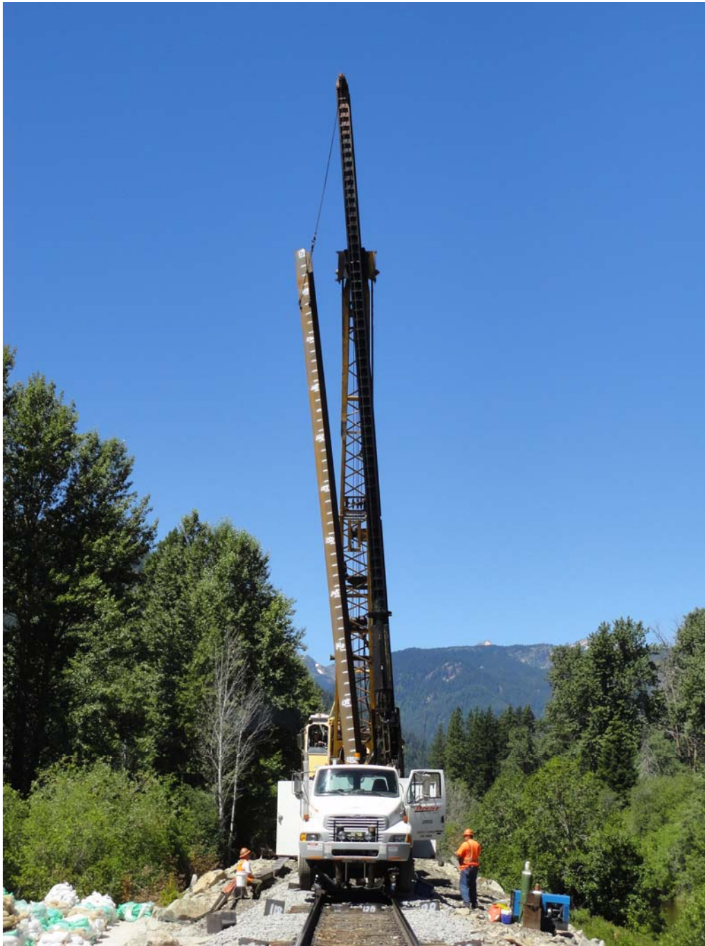
Photo 2: View of Bent 3 Pile 3 Segments 3 being positioned for pile driving.
