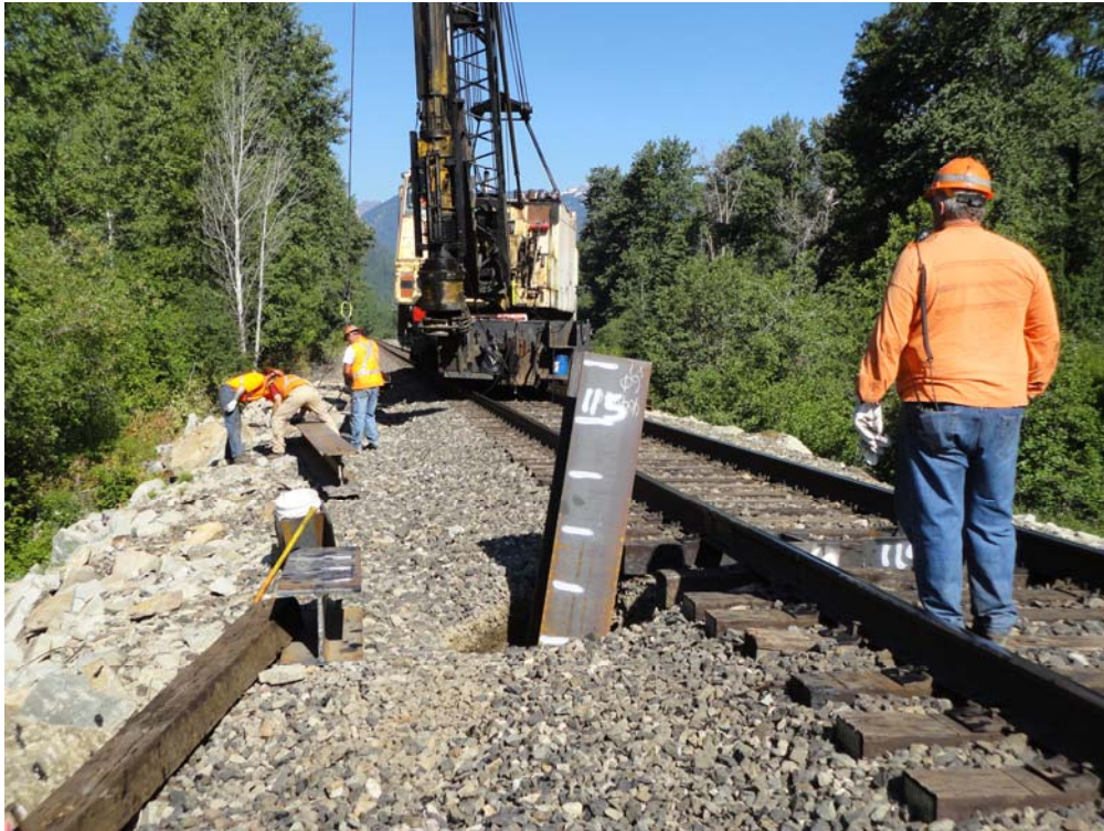
Photo 3: View of the Pier 3 Pile 1 during pile driving. BNSF is picking up their follower to drive the piles below the track level.
