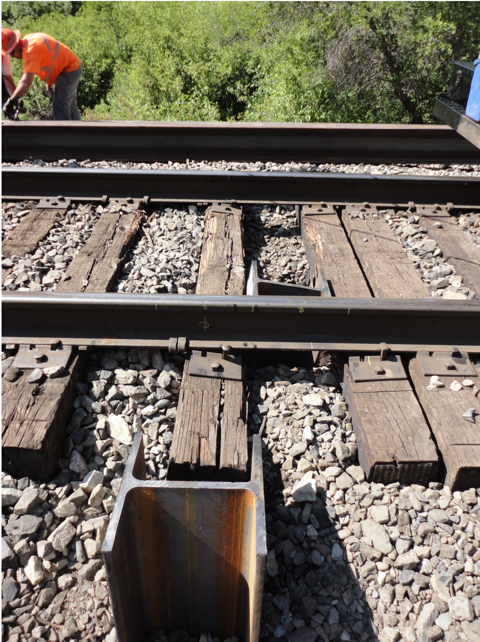
Photo 2: View of the piles at Bent 4. Note the batter on Pile 3 (top of photo) compared to Pile 4 (bottom of photo).
