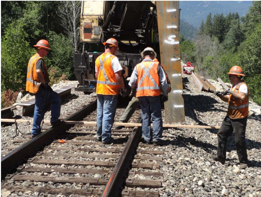
Photo 2: View of the pile being started at Pier 4 Pile 4.
