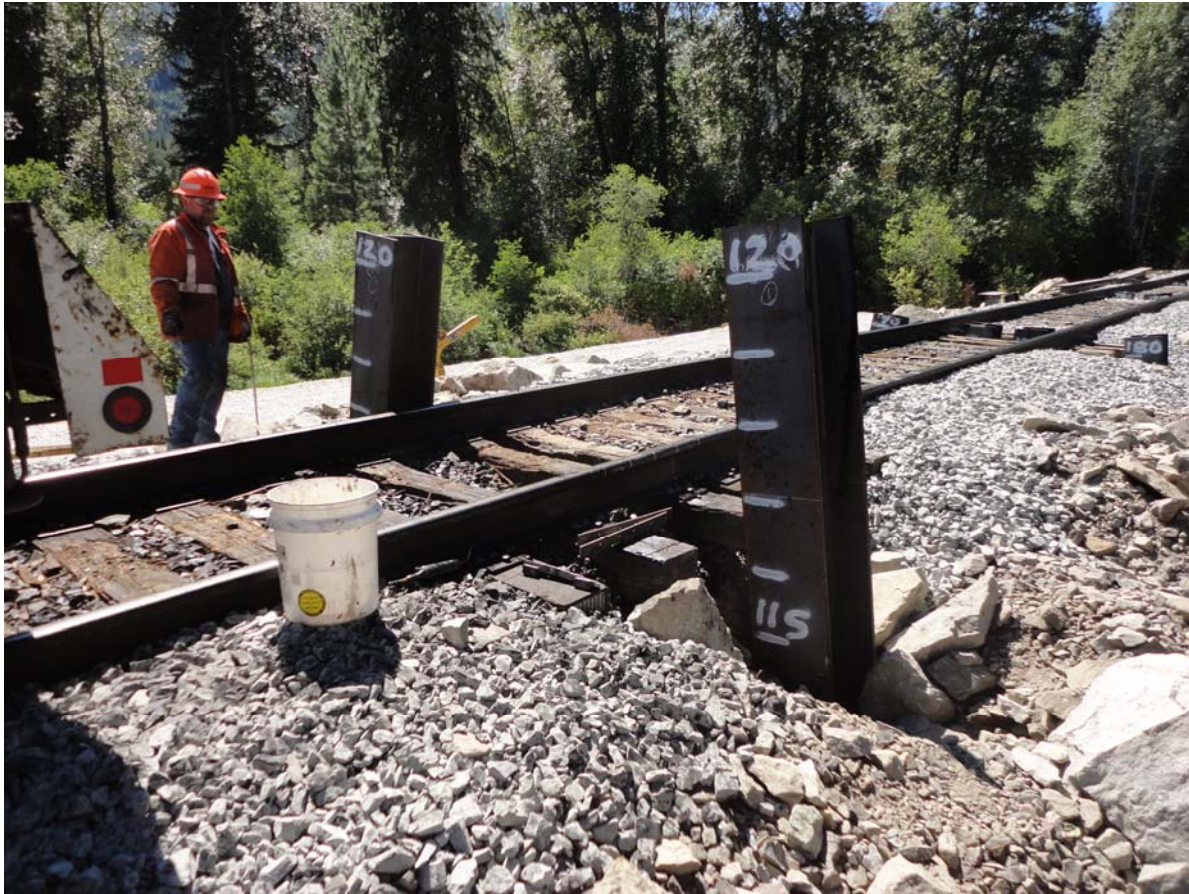
Photo 3: View of Bent 1 Pile 1 (left) and Bent 1 Pile 4 (right) at the end of driving before they were cut off at around 117 feet.
