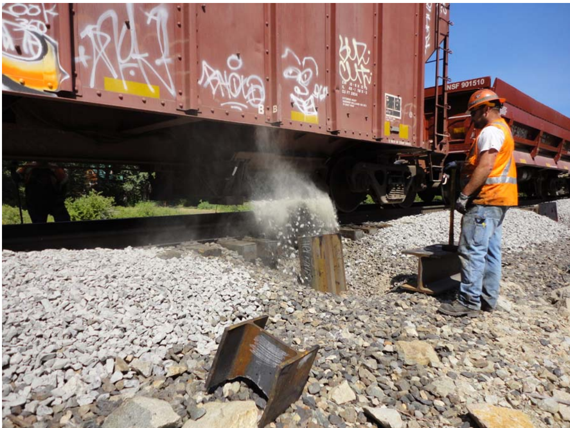
Photo 4: View of additional crushed rock being deposited to fill the holes beneath the railroad ties that developed during pile driving.
