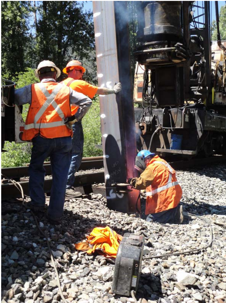
Photo 1: View of first and second segments of Pier 3 Pile 4 being welded together.
