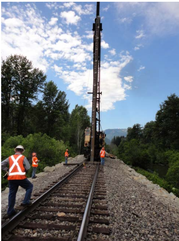
Photo 2: View of Pile 3 before the start of pile driving.
