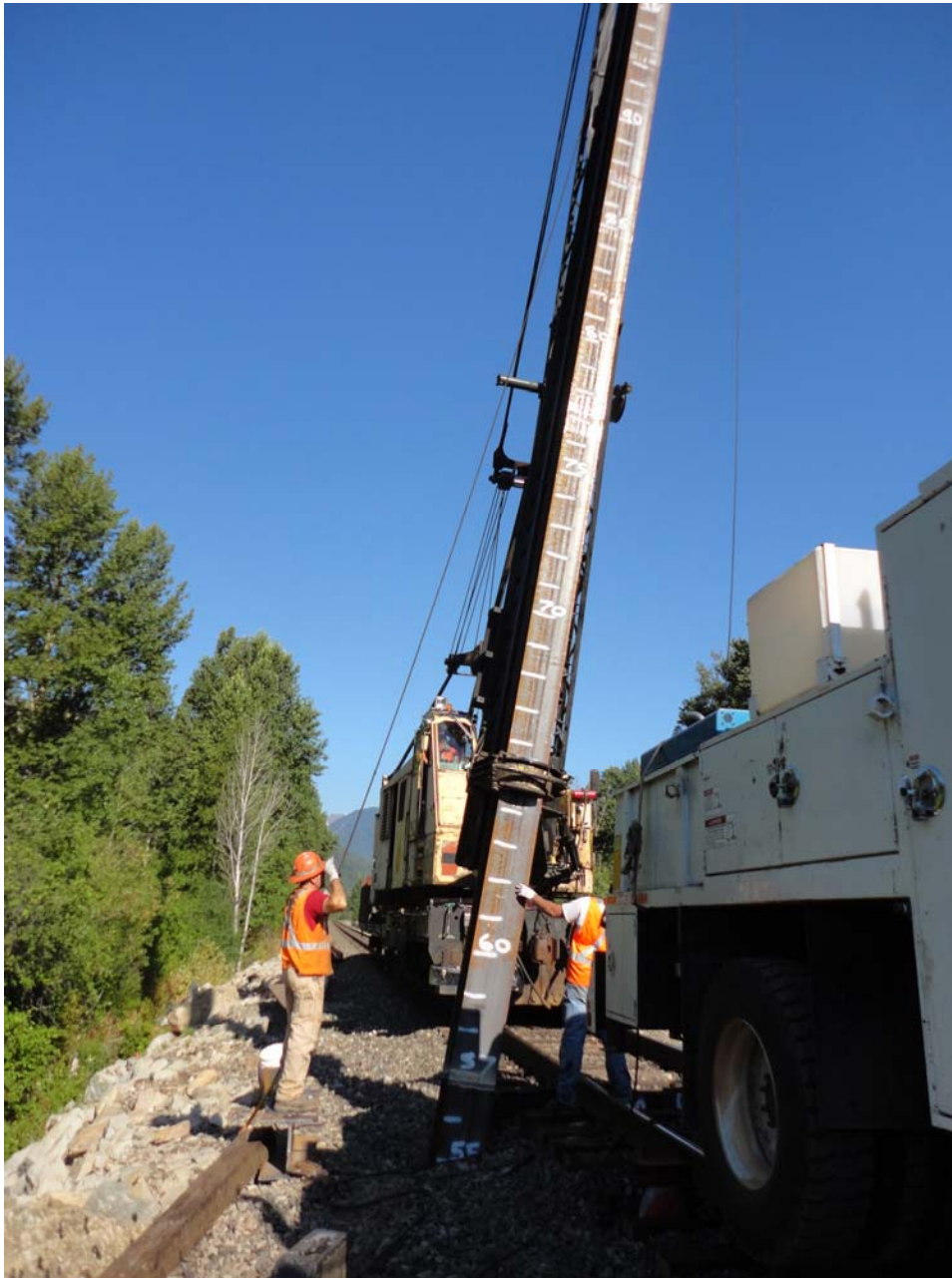
Photo 2: View of the Pier 3 Pile 1 at the start of pile driving.
