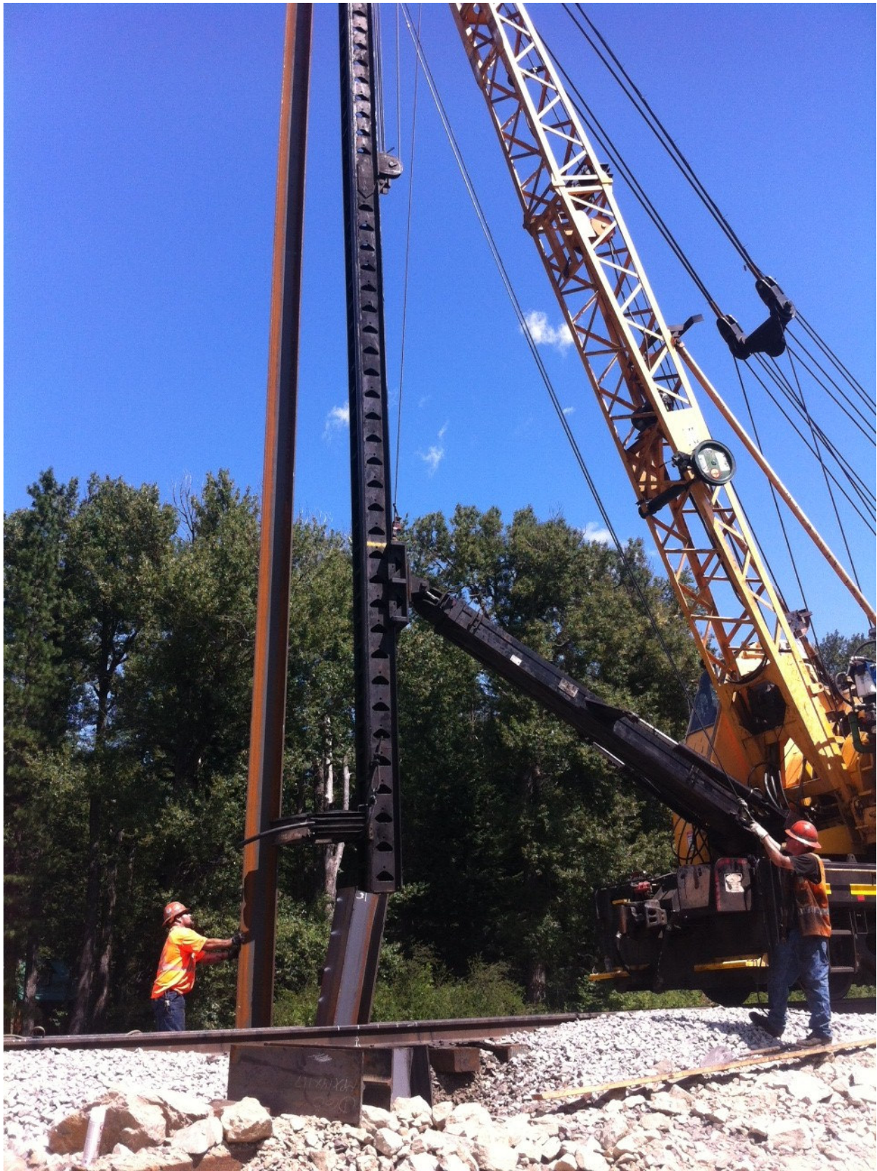
Photo 1: Preparing to set segment 2 of Pile 3, at Bent 1.
