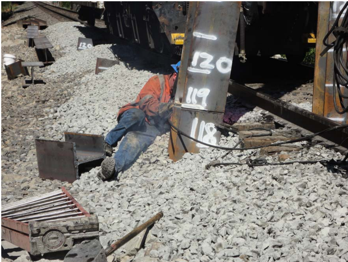
Photo 2: View of pile Segments 2 and 3 being welded together at Bent 2 Pile 1.
