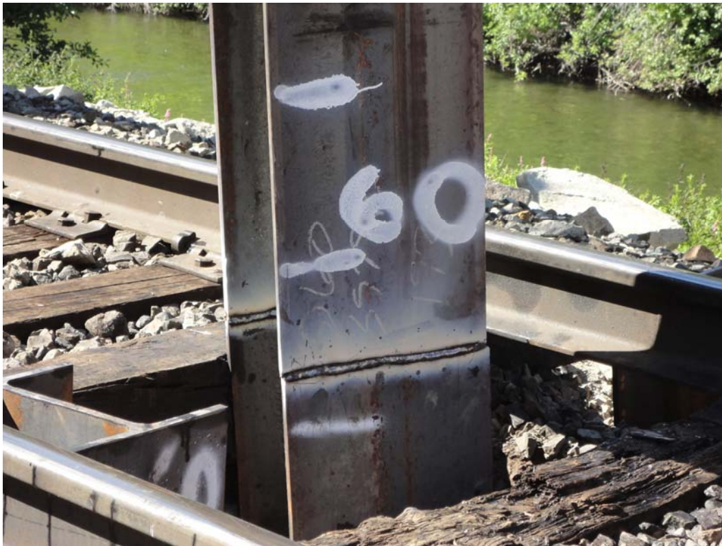
Photo 5: View of weld on Pier 3 Pile 3.
