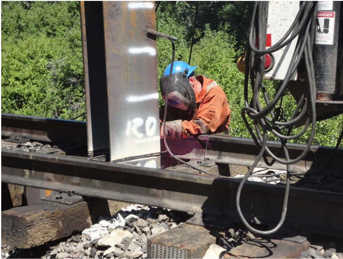
Photo 1: View of Bent 3 Pile 3 Segments 2 and 3 being welded together.
