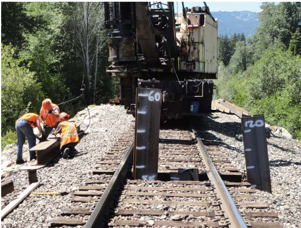
Photo 3: View of Pile 2 and Pile 4 advanced as far as they can be using just the hammer. BNSF crew is attaching cables to pick up the temporary pile section that they will use to drive the piles to below the track elevation.
