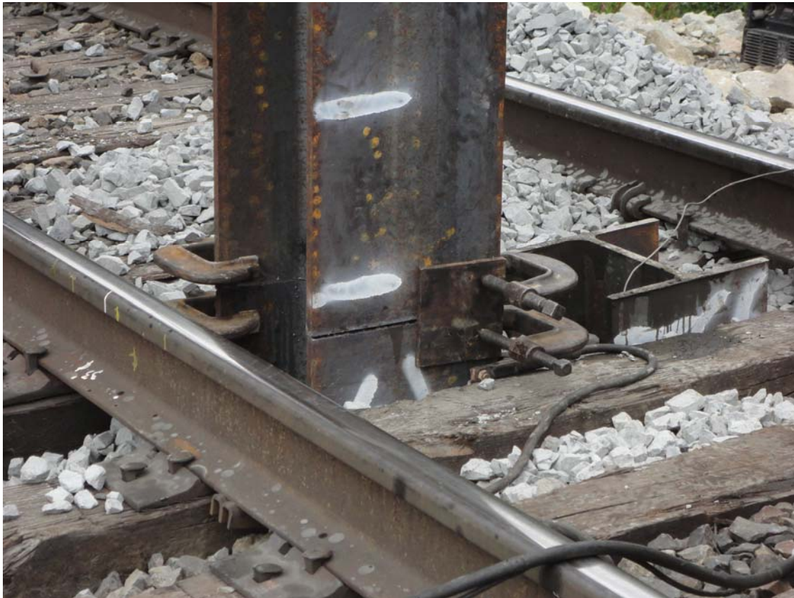
Photo 2: View of Bent 2 Pile 2. First and second segments are clamped together in preparation for welding.
