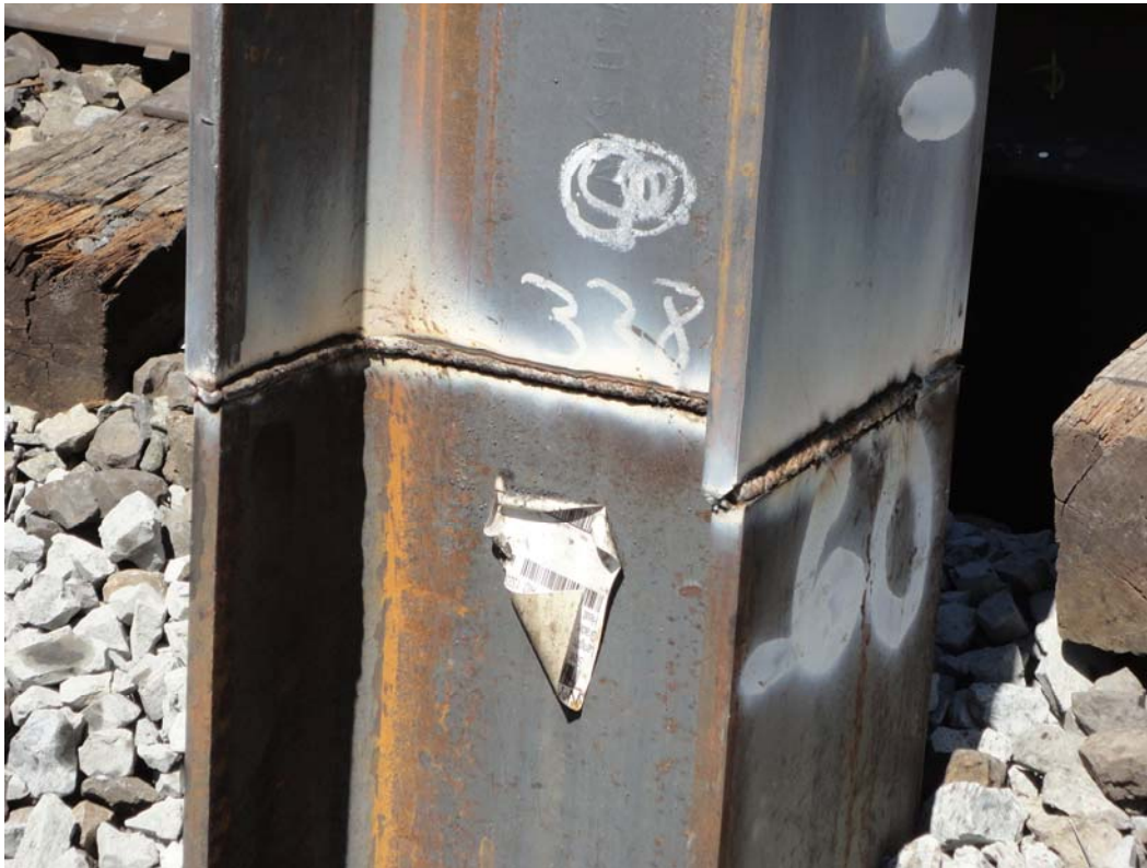
Photo 1: View of the weld at Bent 2 Pile 1.
