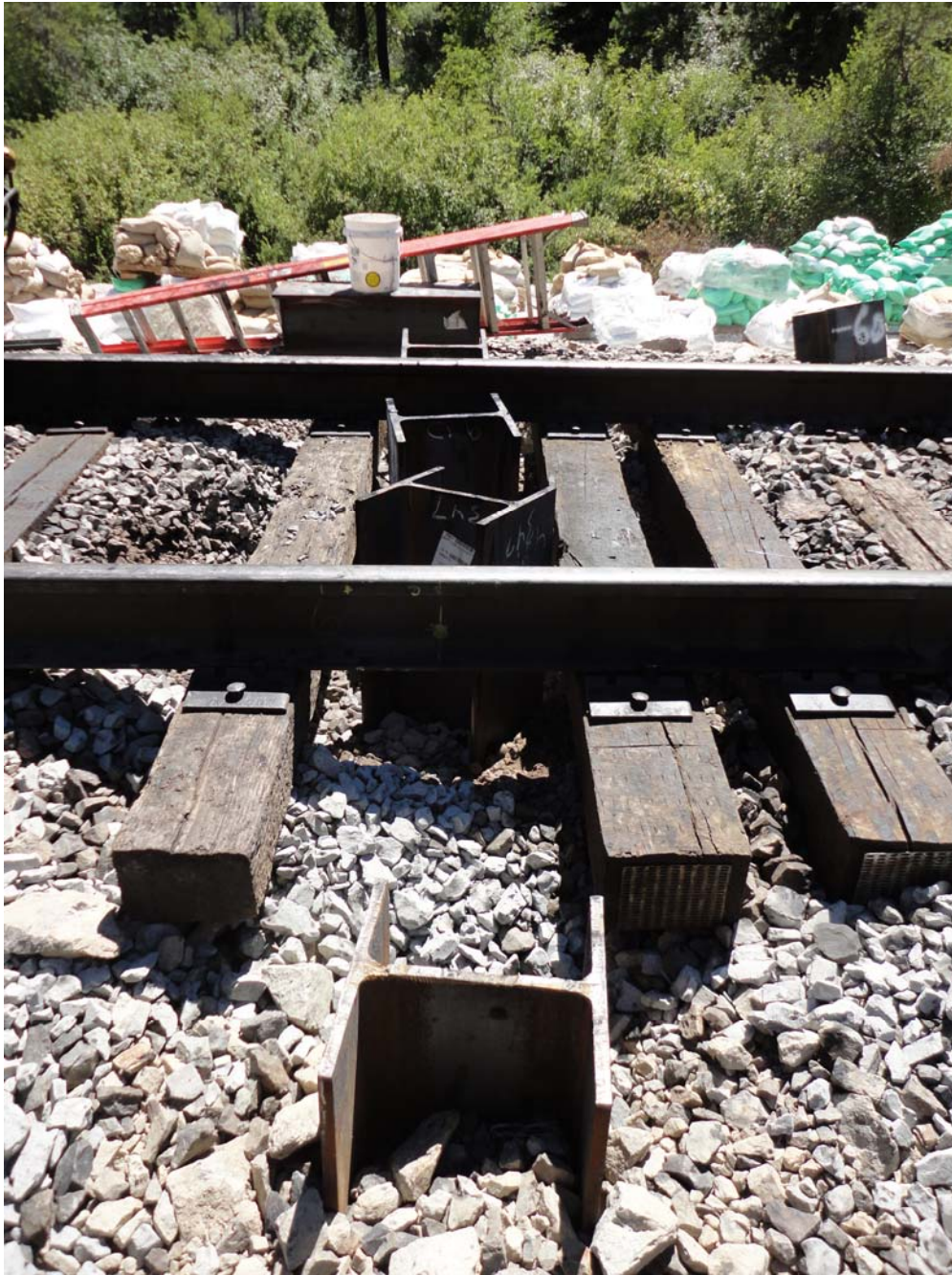
Photo 3: View of the pile group at Bent 3. Pile 4 is in the foreground, pile 1 is in the background. Note the rotation of Pile 3 that occurred during pile driving.
