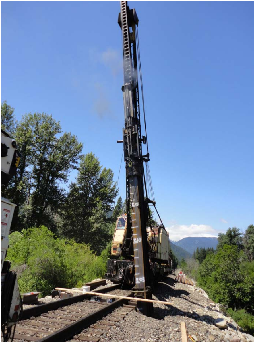
Photo 2: View of the Pier 3 Pile 4 during pile driving.
