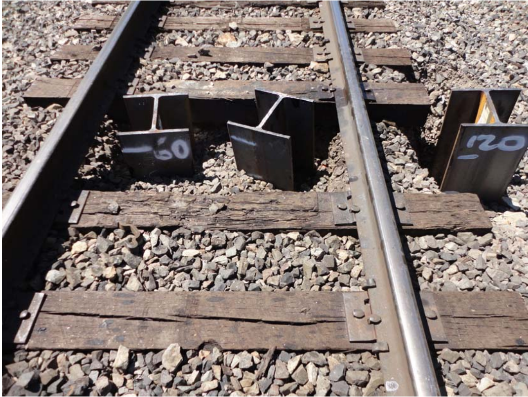
Photo 4: View of Piles 2, 3, and 4 (left to right) at Pier 3. Note the slight rotation of Pile 2 and Pile 3.
