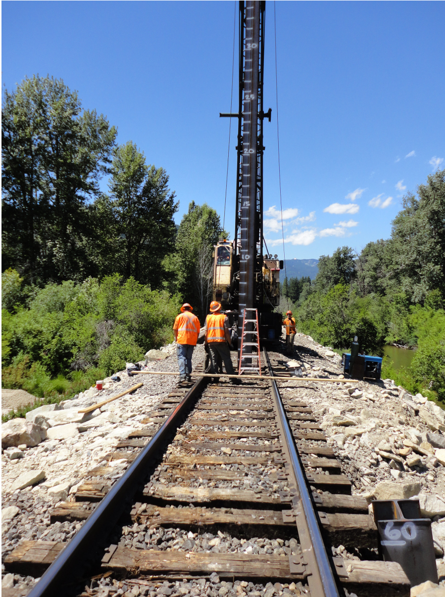
Photo 1: View of the the installation of Bent 2 Pile 1.
