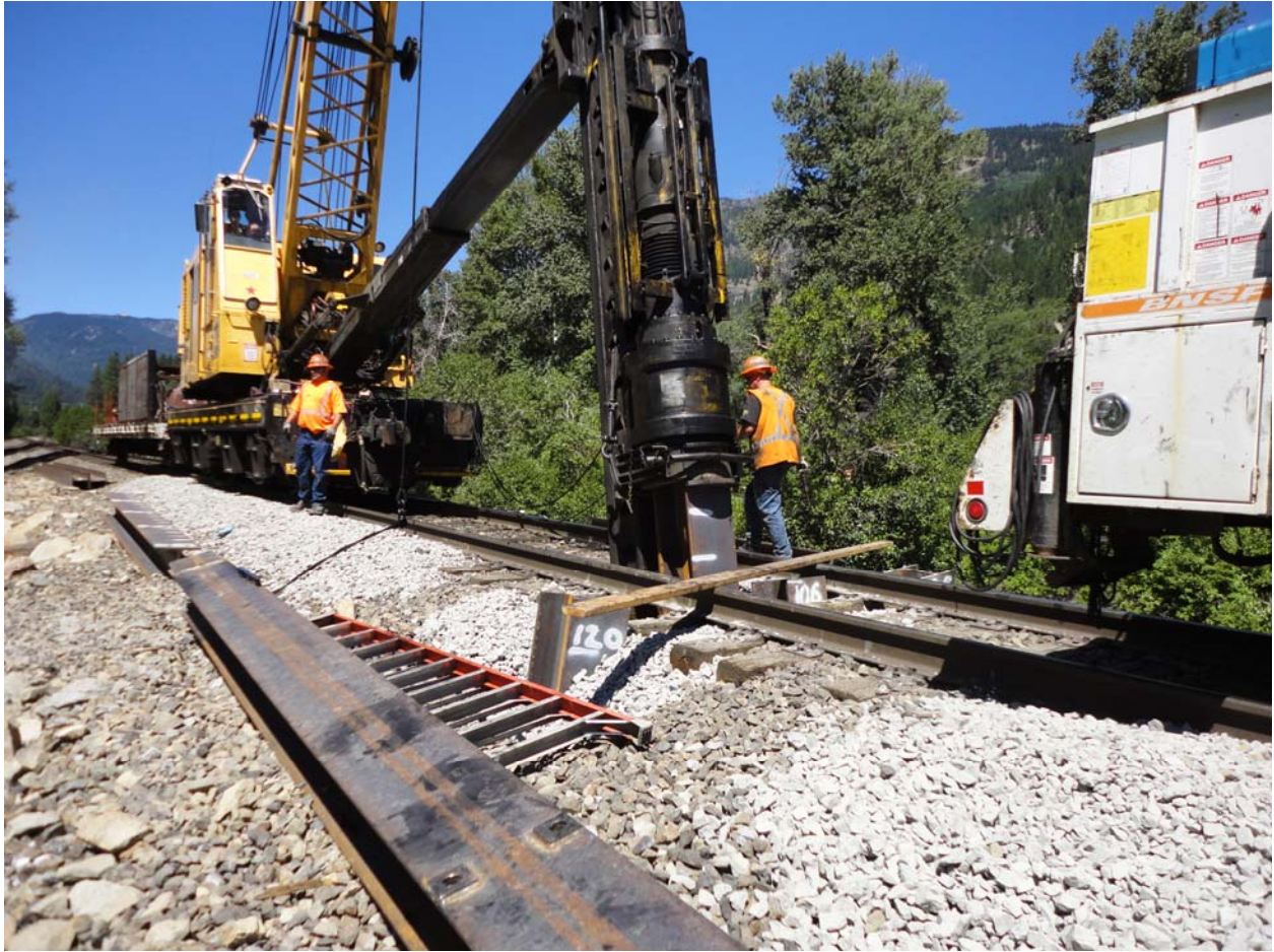
Photo 1: View of Bent 4 Pile 2 near the end of pile driving. The hammer had advanced the pile as far as possible and BNSF was about to pick up their follower and use that to advance the pile below the track elevation.
