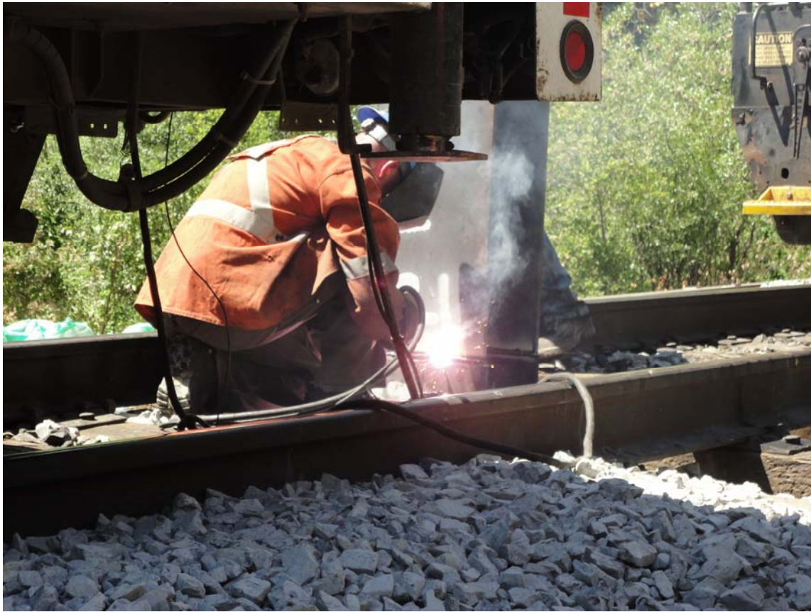
Photo 2: View of Bent 3 Pile 2 Segments 2 and 3 being welded together.
