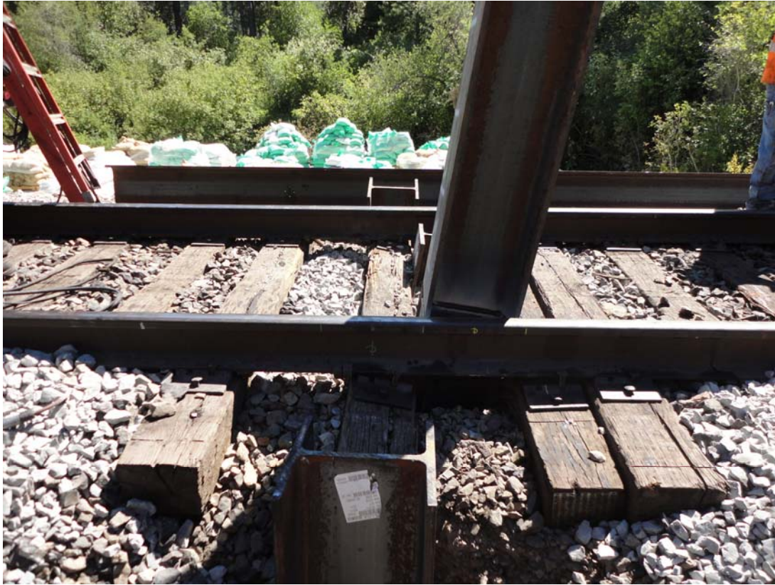
Photo 4: View of Bent 4 Pile 3 sticking above the ground. Note the inclination of the pile, which is intentional.
