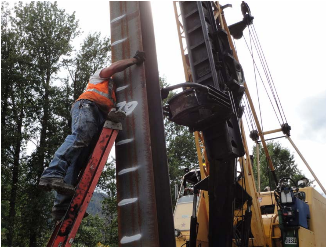
Photo 1: View of Bent 4 Pile 4 Segment 2 about to be attached to the pile driving hammer.
