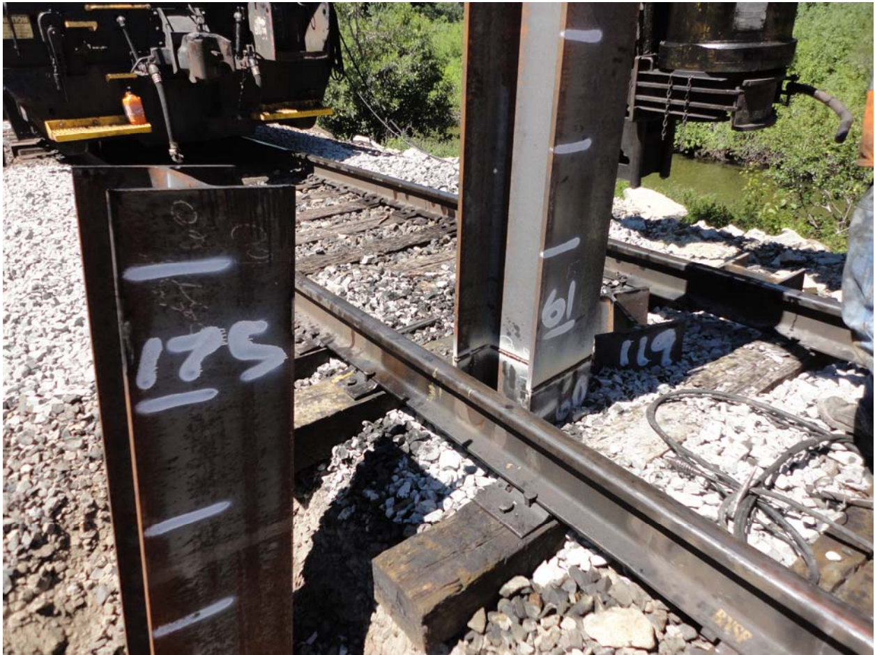
Photo 2: View of Bent 3 Piles 1 and 2 being installed.
