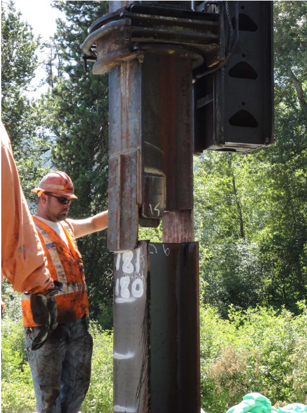
Photo 4: View of the follower being attached to the top of the pile to drive the final 4 feet of pile below the railroad track elevation.
