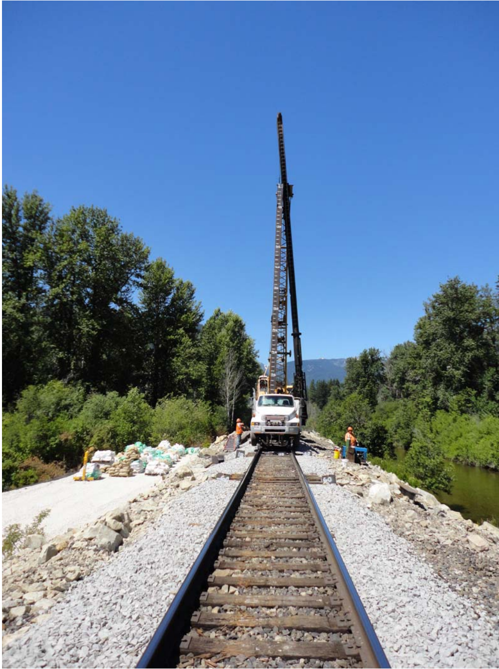
Photo 1: View of the crane picking up a pile segment and moving in into place at Bent 3 Pile 2.
