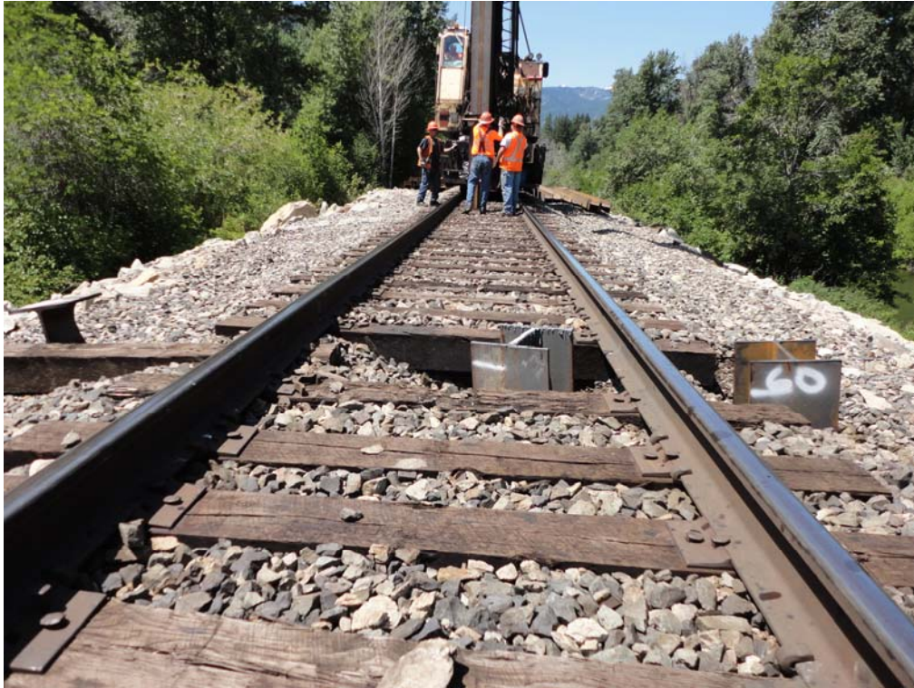
Photo 3: View of Pile 3 and Pile 4 at the end of the day. Note the slight rotation to Pile 3 that was driven yesterday.
