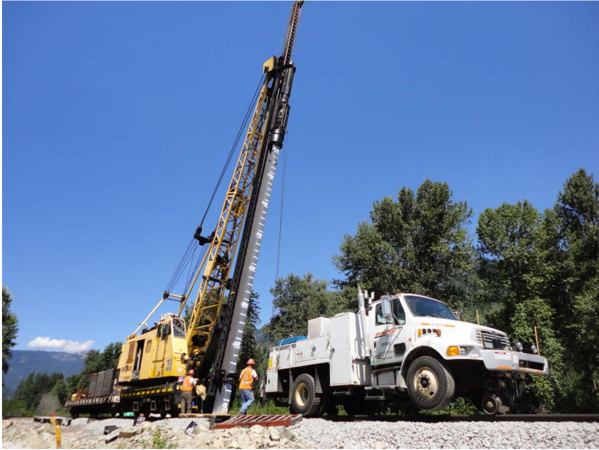
Photo 3: View of Bent 1 Pile 1 segment 3 at the beginning of pile driving.
