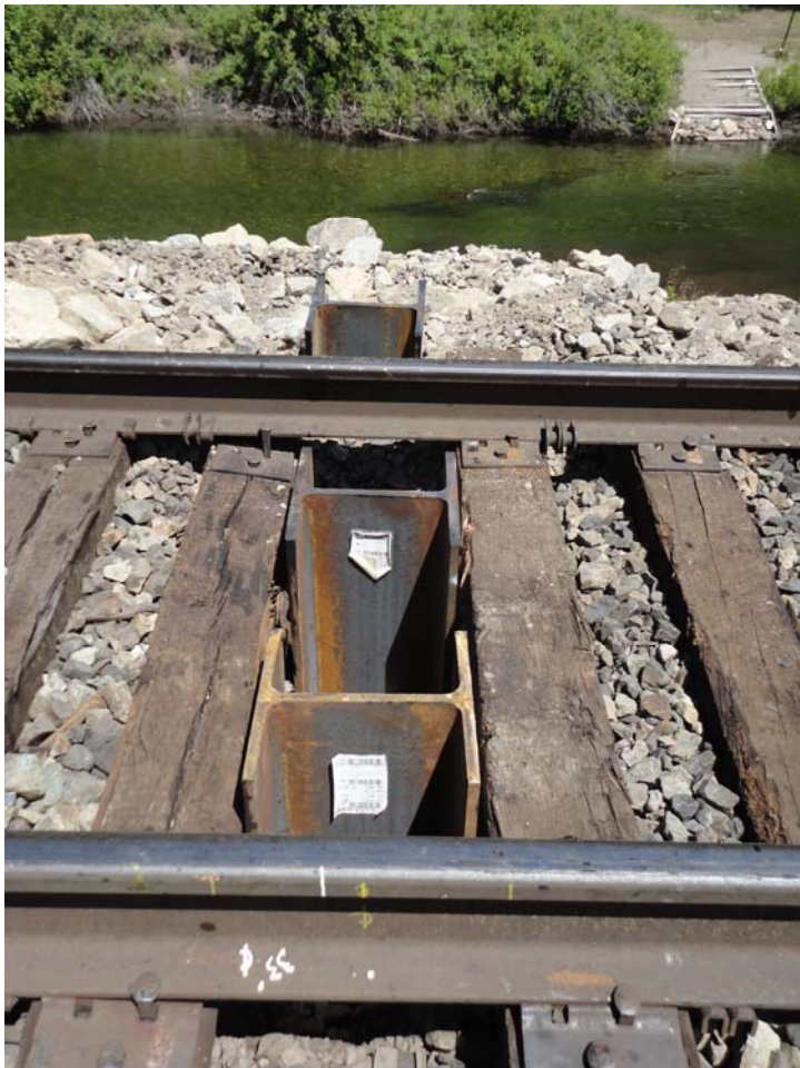
Photo 4: View of the piles that have been advanced so far at Pier 2 (Piles 4, 3, 2 – top to bottom).
