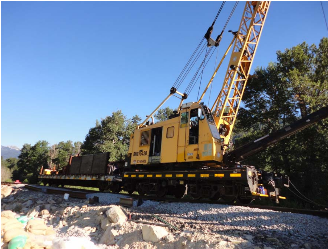
Photo 1: View of the rail mounted crane that was being used to drive the piles.
