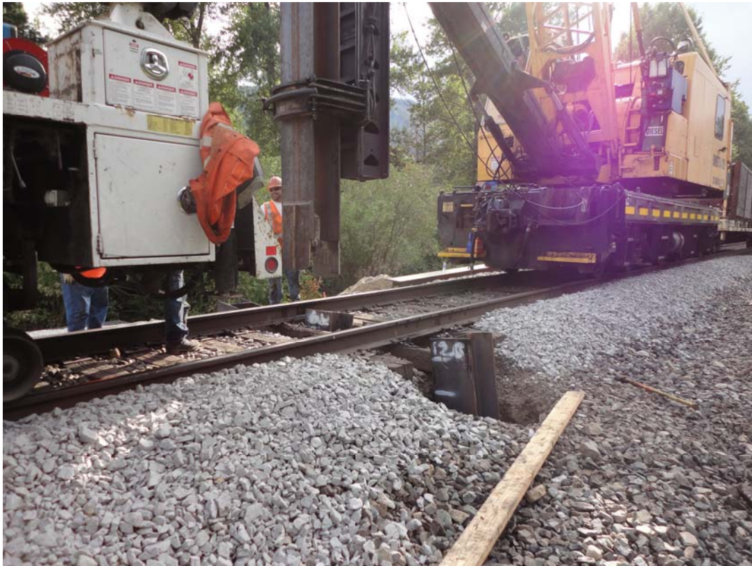
Photo 2: View of the follower being removed from Bent 4 Pile 4 Segment 2 after it has been used to advance the pile below the track elevation. The follower is typically used to advance the last 5 feet of each pile segment because there is not room for the hammer to drive the piles below the track elevation.
