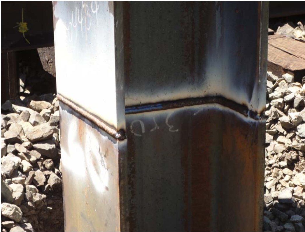
Photo 2: View of the weld between the first and second segment of Pier 3 Pile 4.
