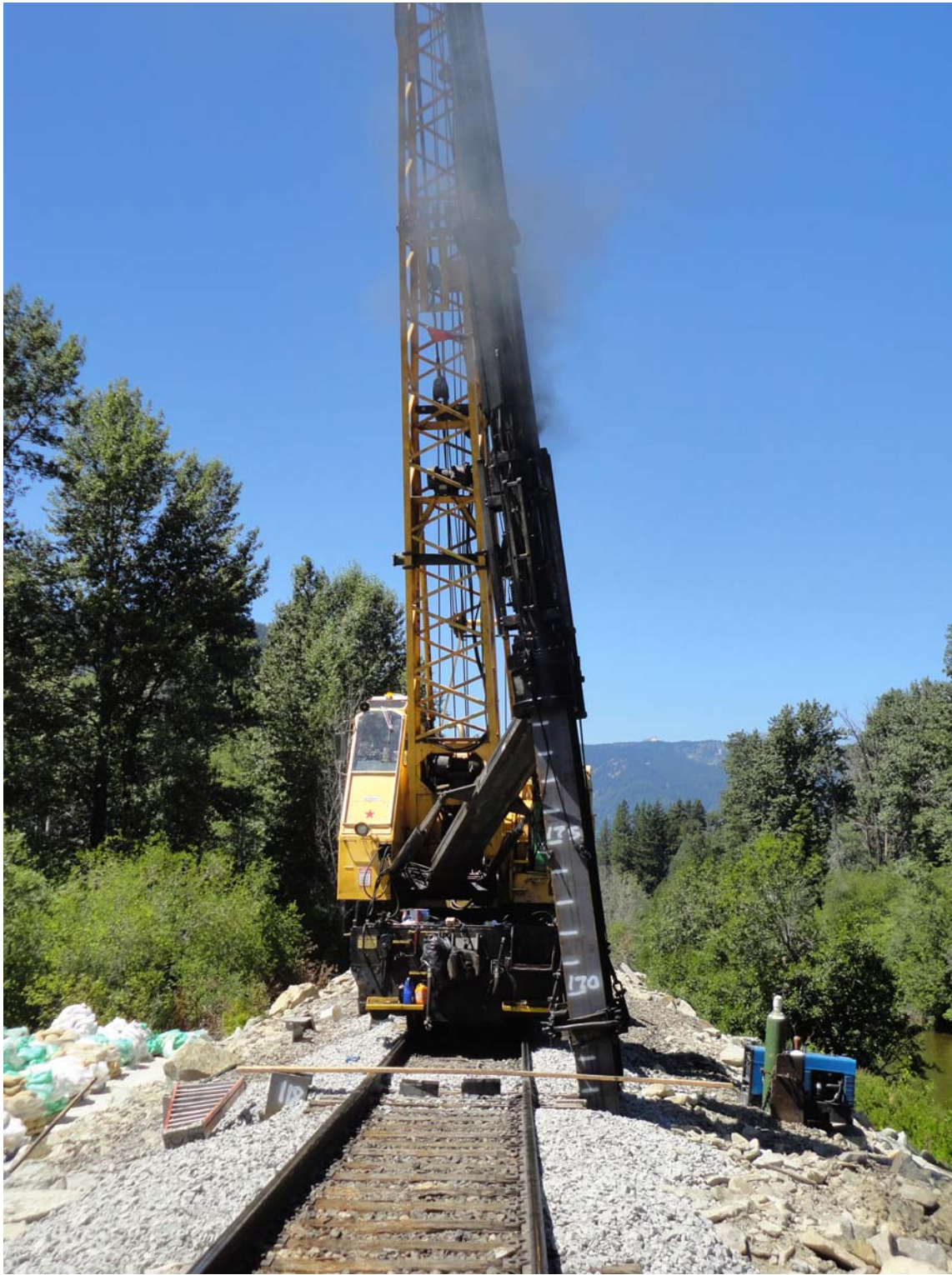
Photo 4: View of Bent 2 Pile 4 Segment 3 near the end of pile driving.
