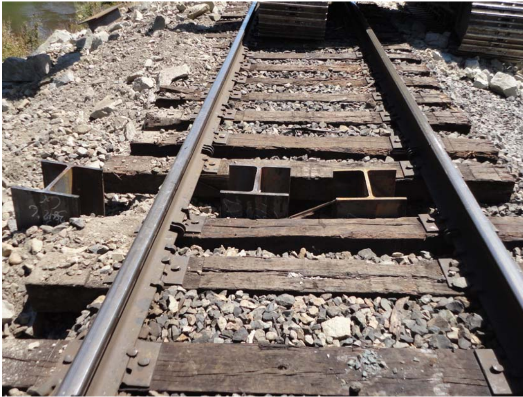
Photo 3: View of the piles that have been advanced so far at Pier 2 (Piles 4, 3, 2 – left to right).
