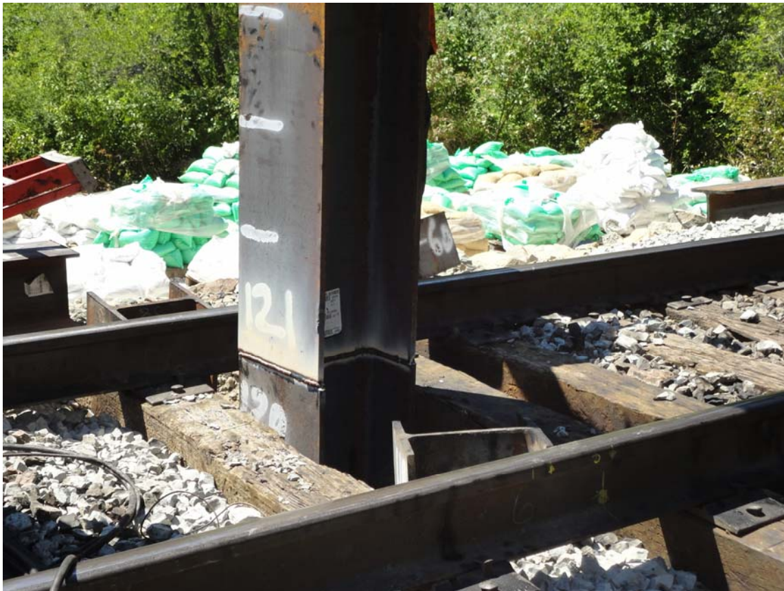
Photo 3: View of the weld at Bent 3 Pile 2 between pile segments 2 and 3.
