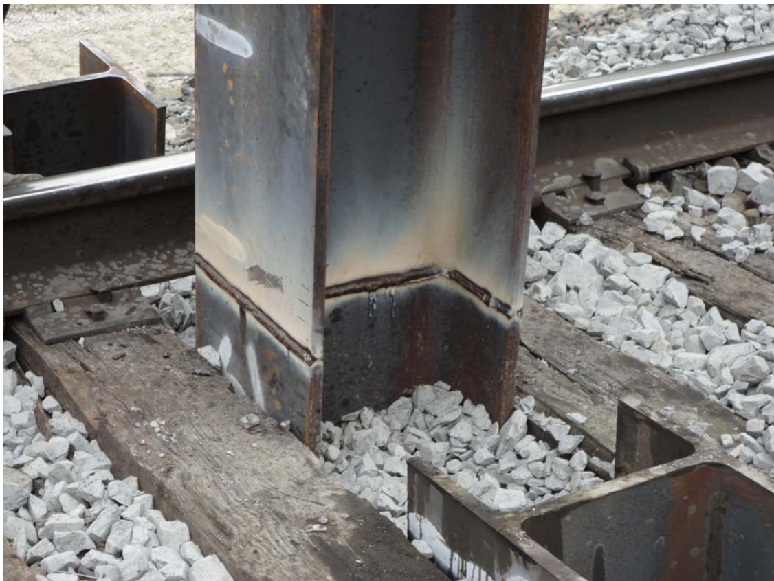
Photo 3: View of Bent 2 Pile 2 after the first and second segments were welded together.
