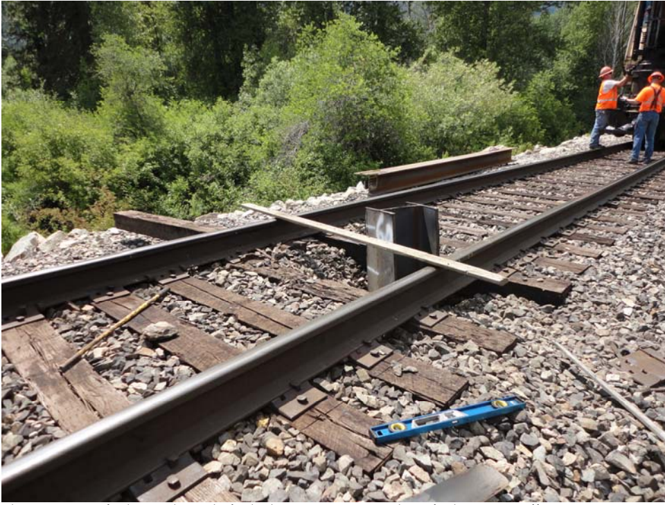
Photo 3: View of Pile 3 at the end of pile driving. Upper 8 inches of pile was cut off.
