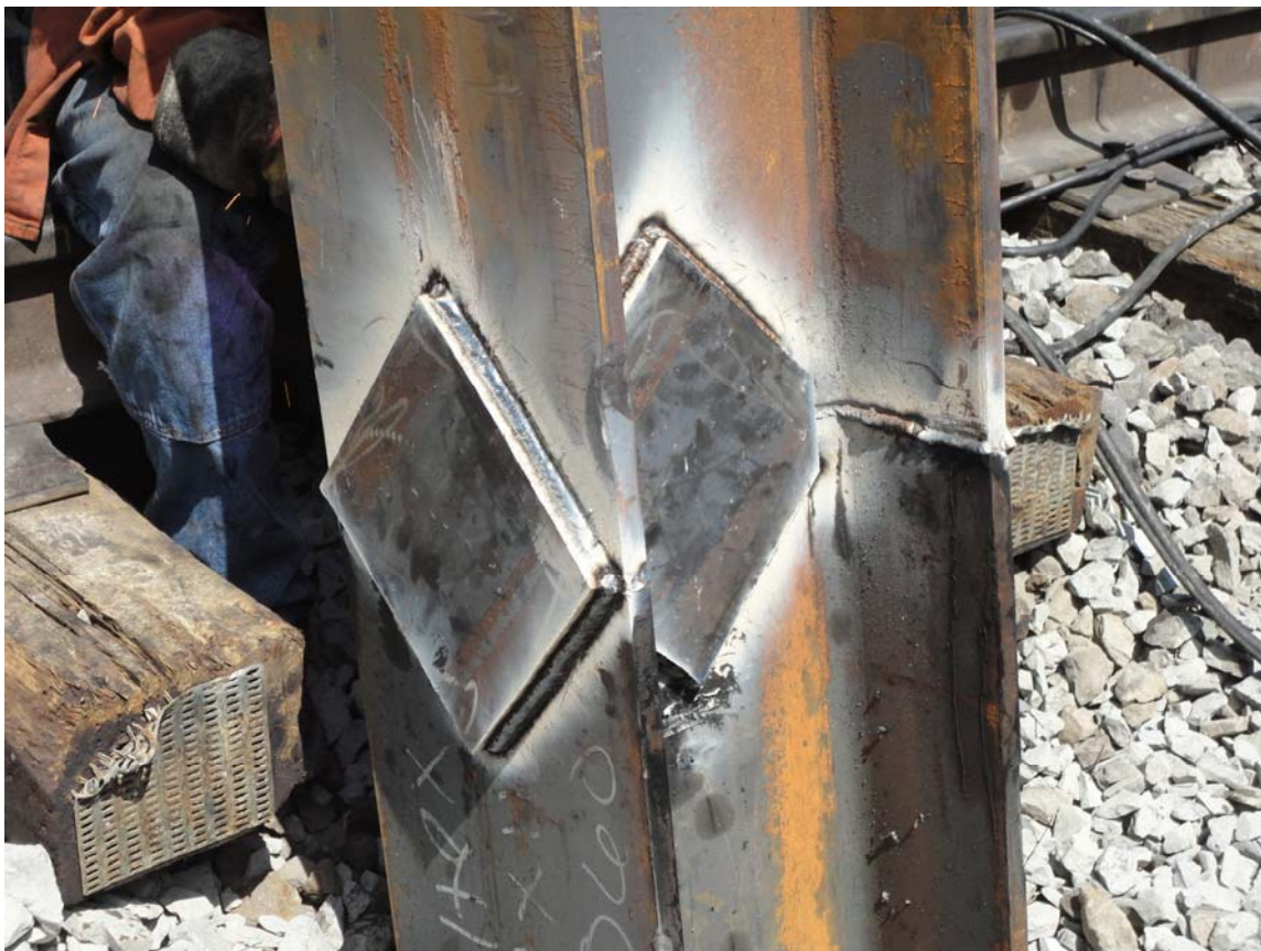
Photo 2: View of the weld at Bent 2 Pile 1 at a depth of 179 feet. Note the diamond shaped stiffener plates that were added because this splice location will be within 15 feet of finish grade.
