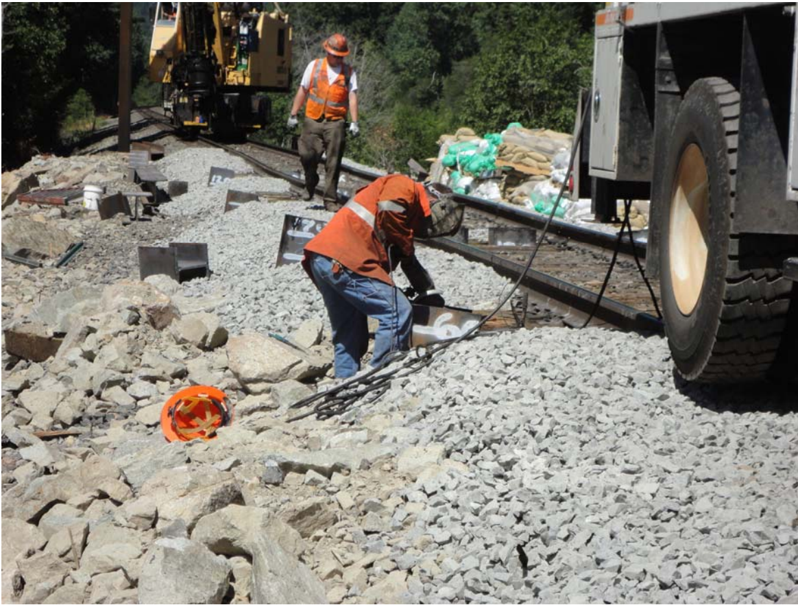
Photo 1: View of the top of Bent 1 Pile 1 being ground off in preparation for pile welding.
