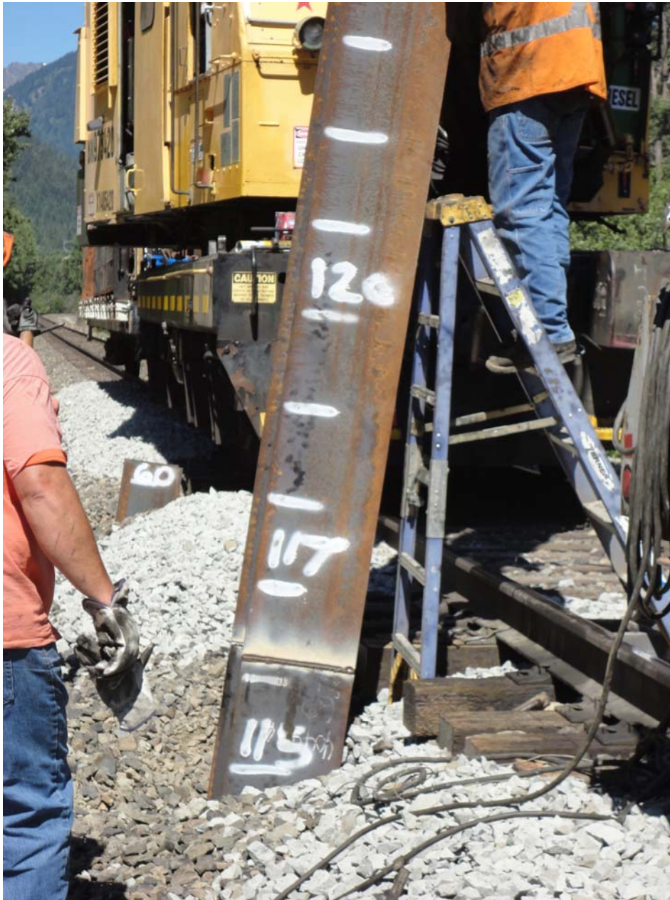
Photo 1: View of Bent 3 Pile 1 being installed.
