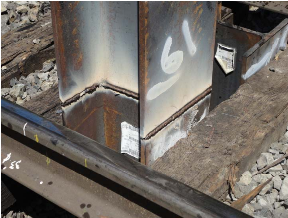
Photo 1: View of the the weld at Bent 2 Pile 2 at 60 feet.
