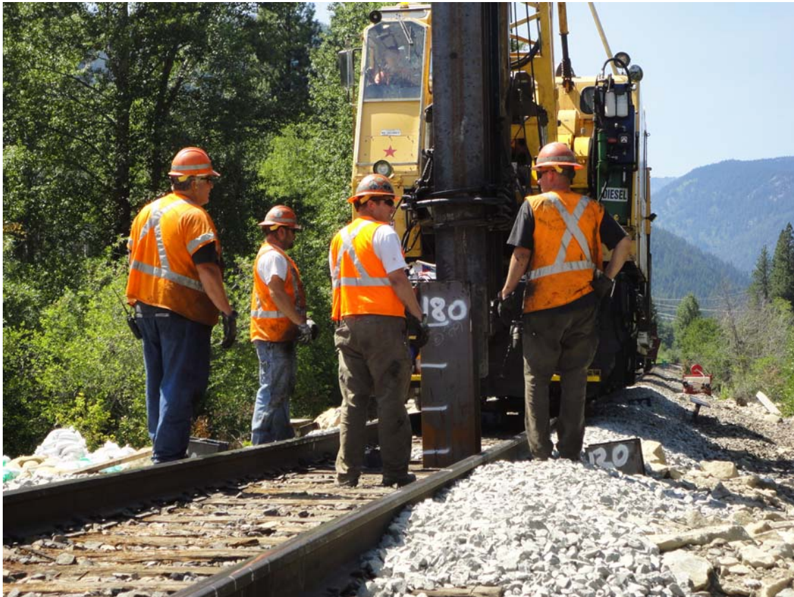
Photo 3: View of Bent 2 Pile 3 near the end of pile driving. The hammer has advanced the pile as far as it will go; BNSF is preparing to attach their follower to advance the pile below the track elevation.
