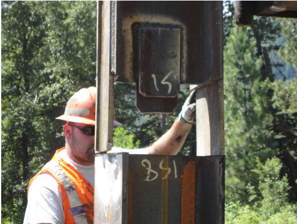
Photo 5: View of the follower that BNSF uses to drive the piles below the track level. (Follower at the top of the photo, pile at the bottom of the photo)
