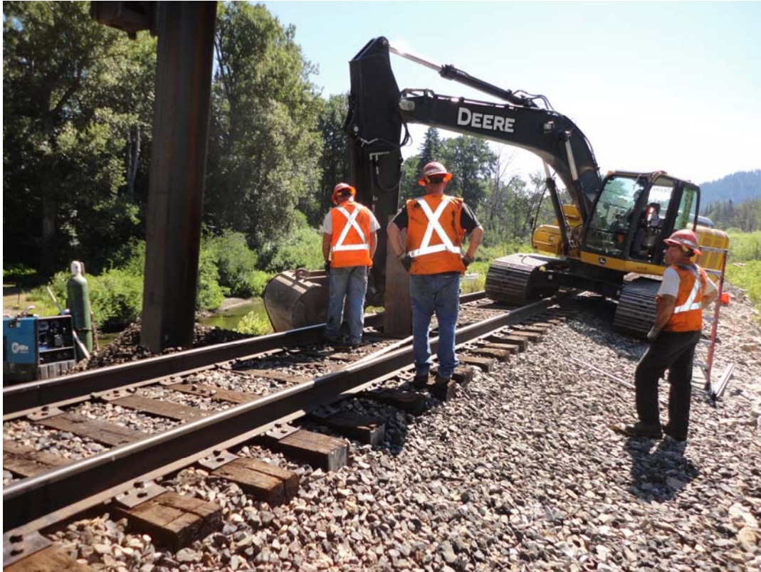
Photo 1: View of the excavator digging a hole at Pier 2 Pile 4 to remove the obstruction that was rotating the pile.
