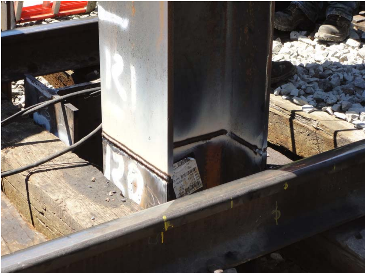
Photo 2: View of the finished weld on Bent 2 Pile 3 at a depth of 120.5 feet.
