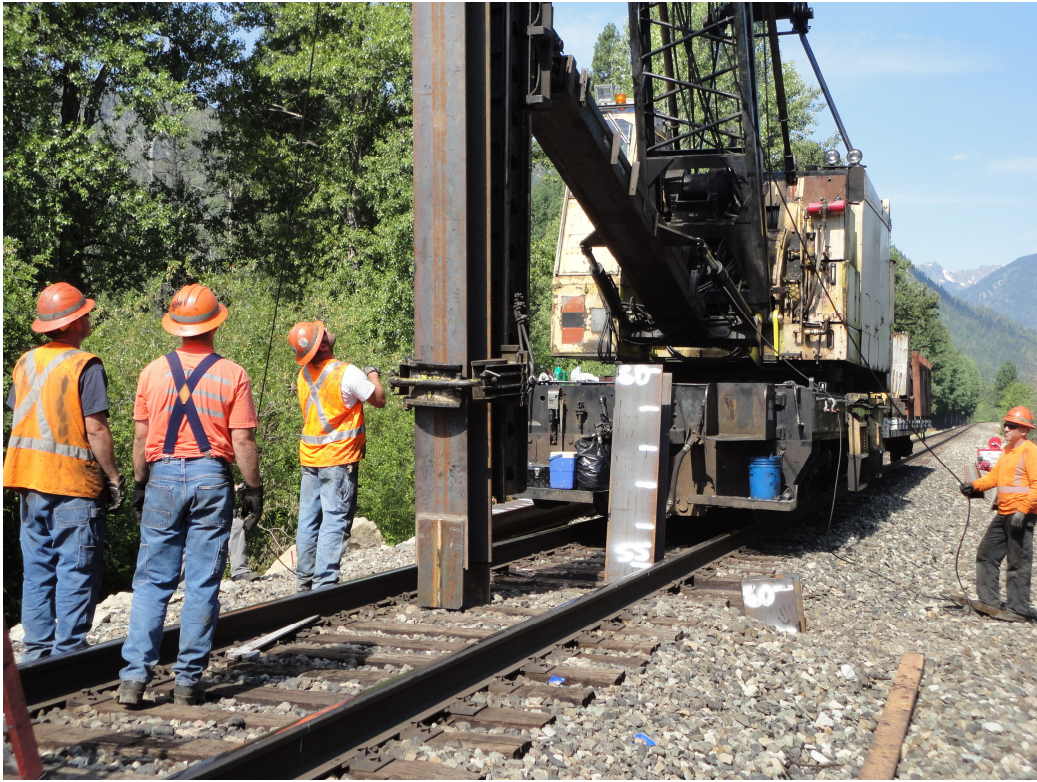
Photo 1: View of the the installation of Bent 4 Pile 3. Crew is preparing to use the follower to further advance the pile.
