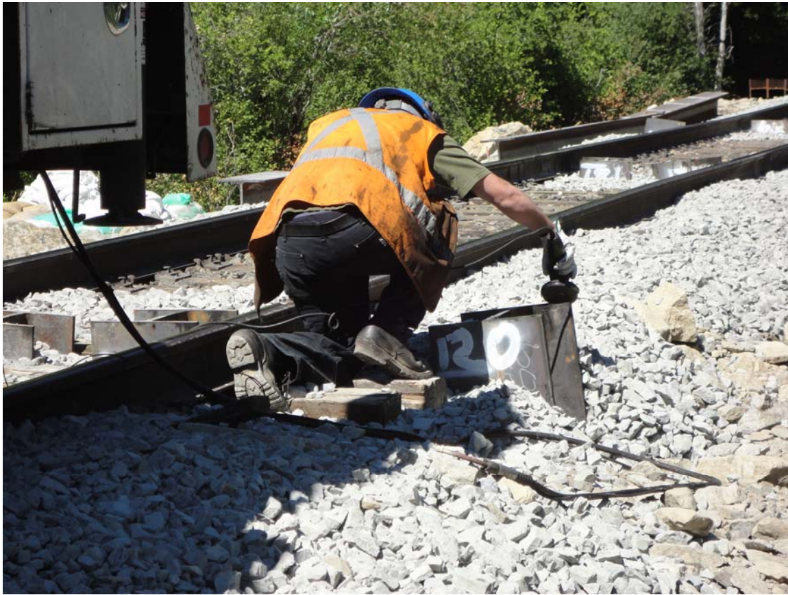
Photo 1: View of Bent 2 Pile 4 being ground off at 120 feet in preparation for welding on another pile segment.
