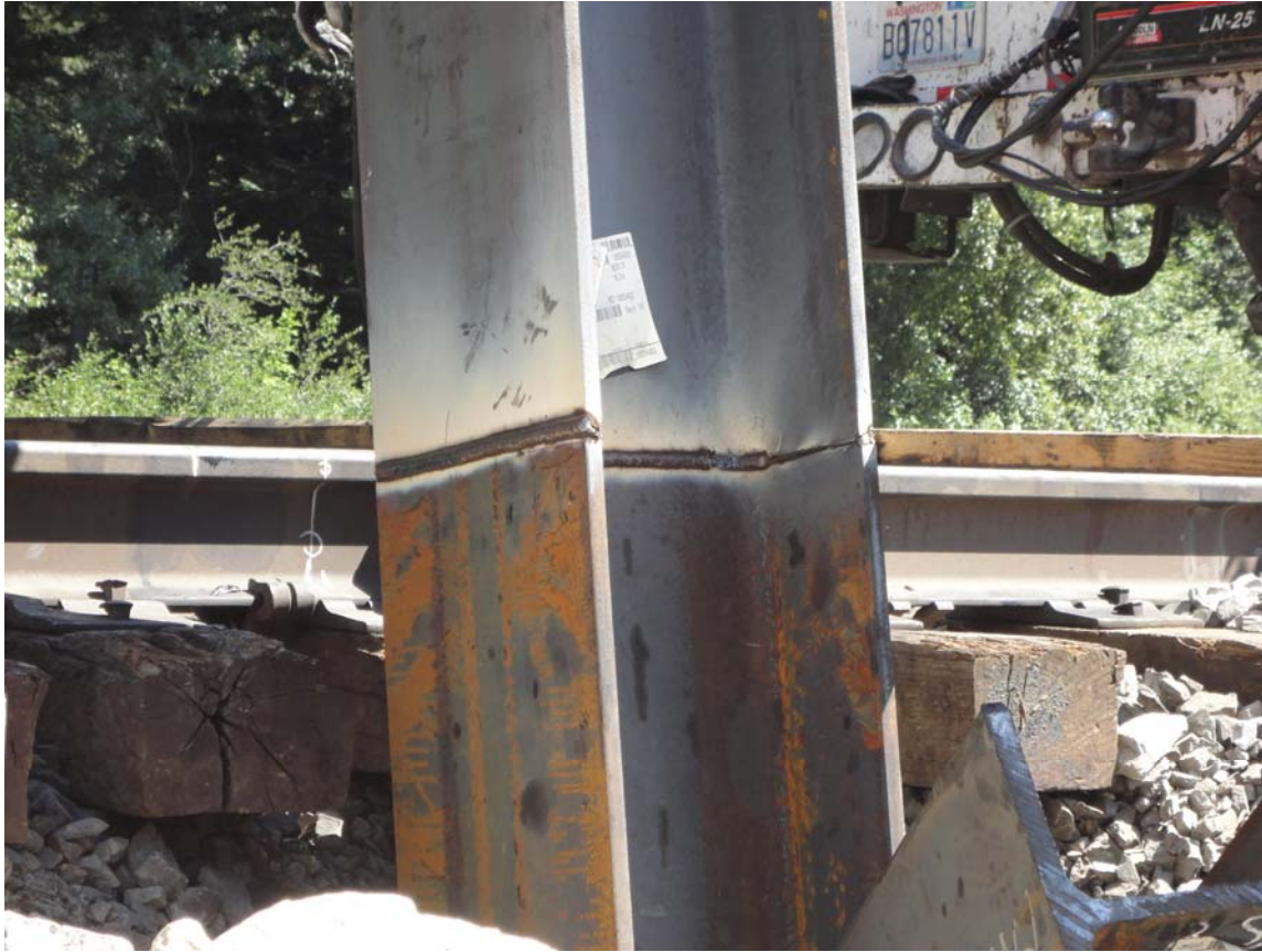
Photo 1: View of the weld at Bent 1 Pile 1 at a depth of 120 feet. Most of the splices on this project look similar to this.
