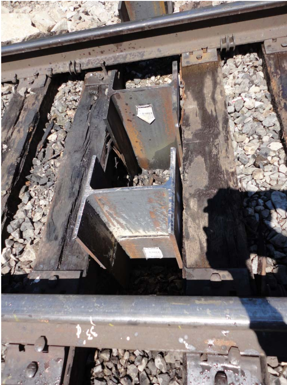
Photo 2: View of Bent 2 Pile 2 in the foreground. Note the weld that is 1 foot below the top of the pile, due to the pile needing to be cut off after only 1 foot of driving.
