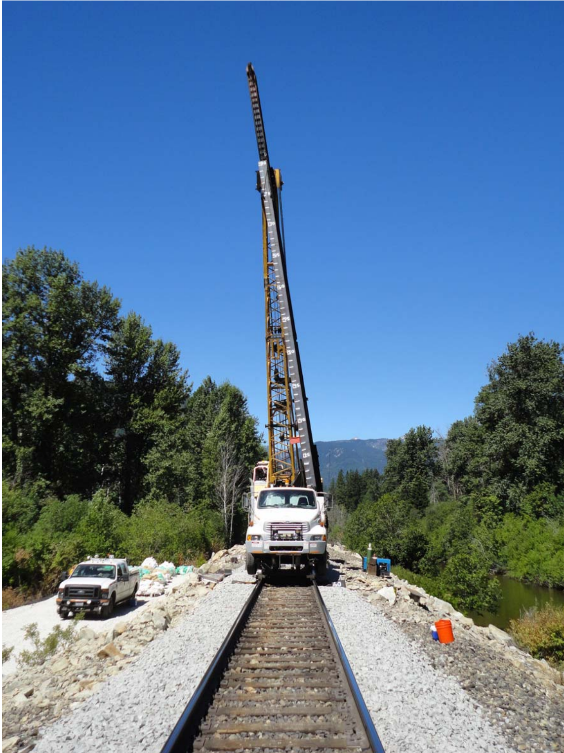
Photo 3: View of Bent 2 Pile 4. The third pile segment is being held in place by the crane as it is being welded together with the previous segment. Note the batter of the pile.
