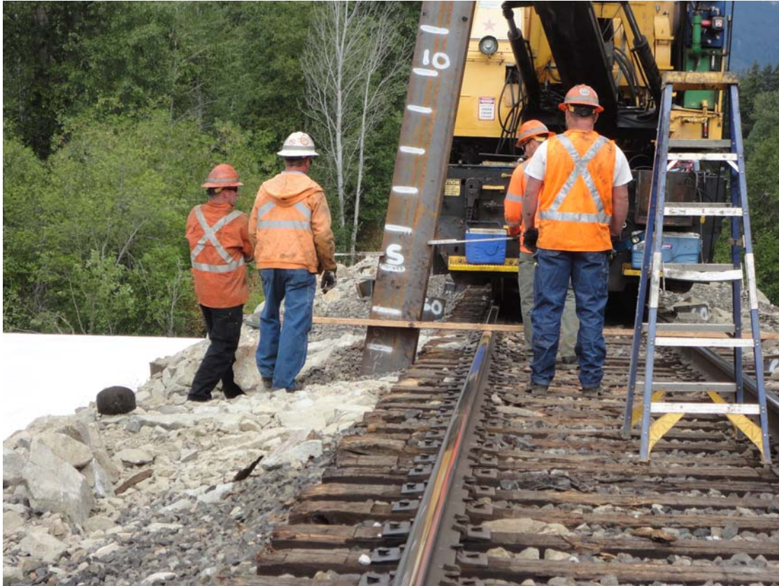
Photo 1: View of the installation of Bent 1 Pile 1. Note the levers being used to help the pile initially go in straight.
