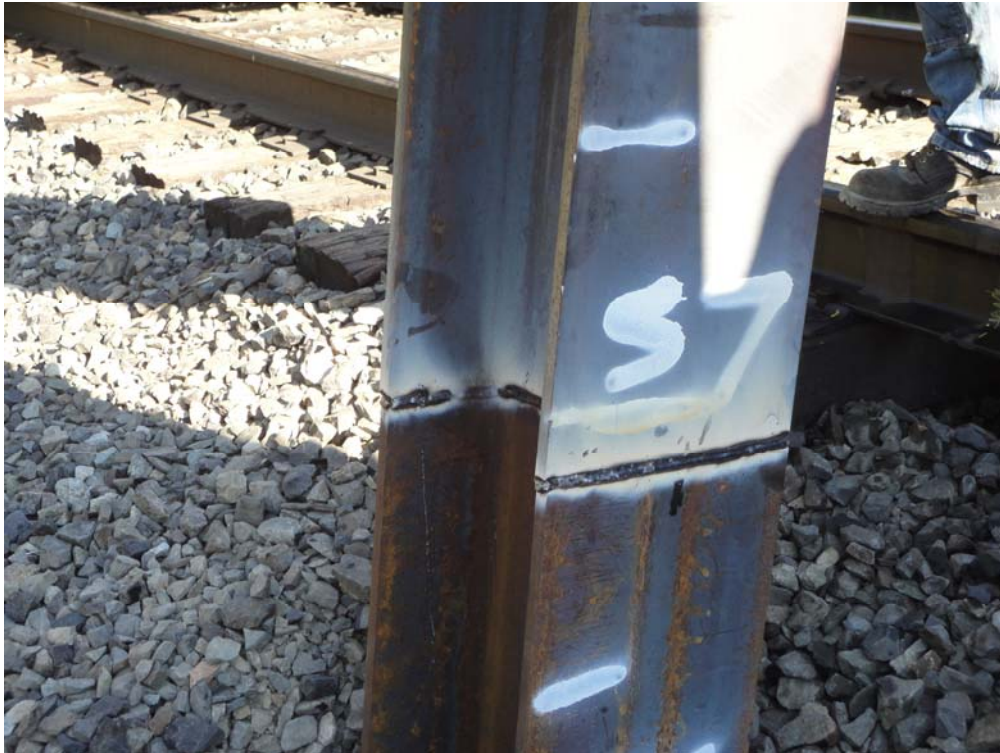
Photo 1: View of the weld on Pier 3 Pile 1 at 55 feet, between segments 1 and 2.
