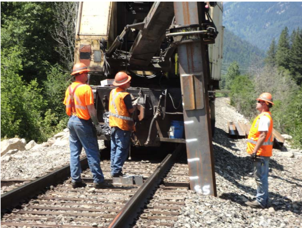
Photo 2: View of the temporary pile extension that was used to drive the pile from 55.5 to 60 feet.
