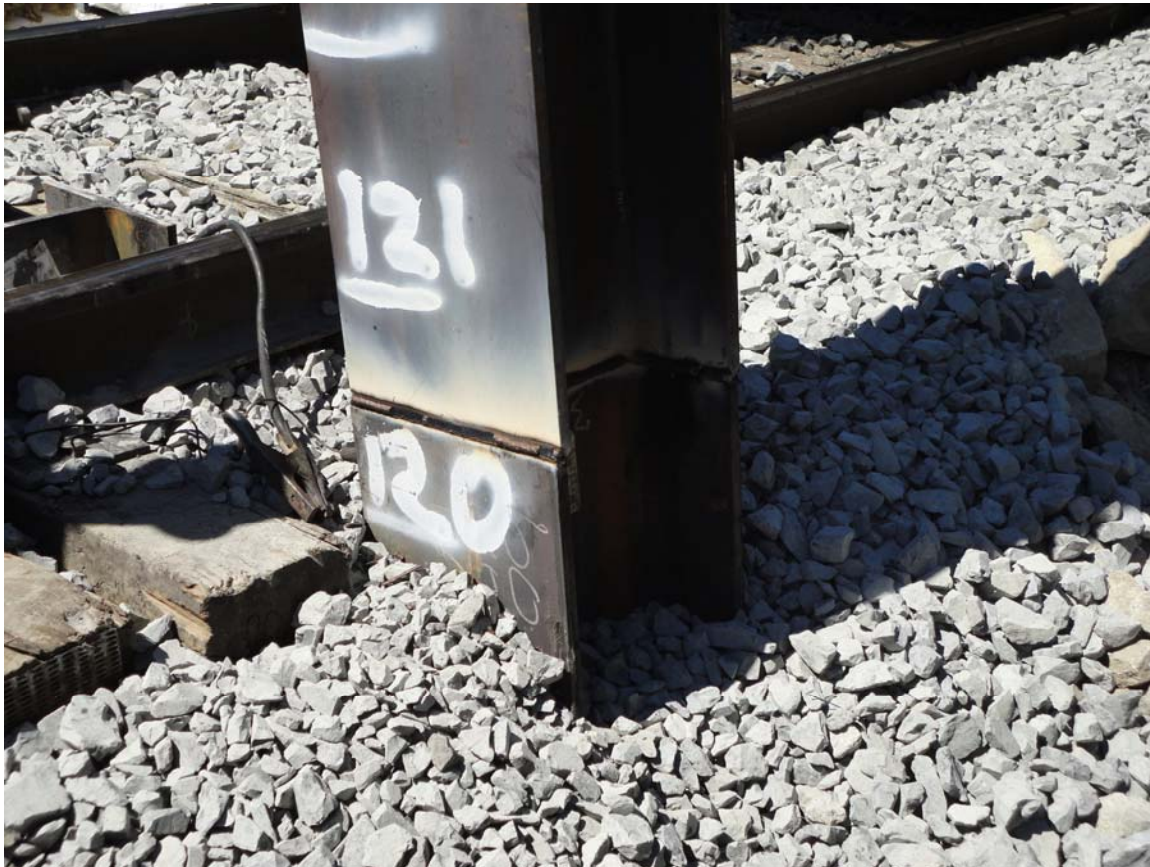
Photo 2: View of the finished weld on Bent 2 Pile 4 at a depth of 120.5 feet.
