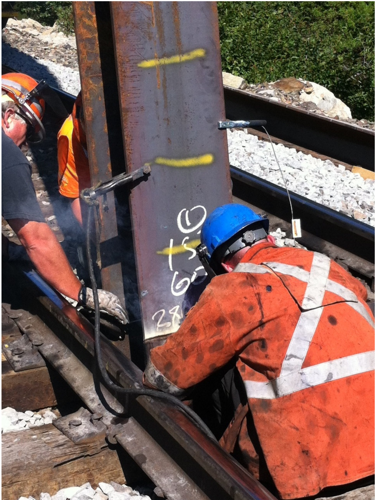
Photo 1: Welding segment 3 at Bent 4 Pile 2 at a depth of 120 feet.
