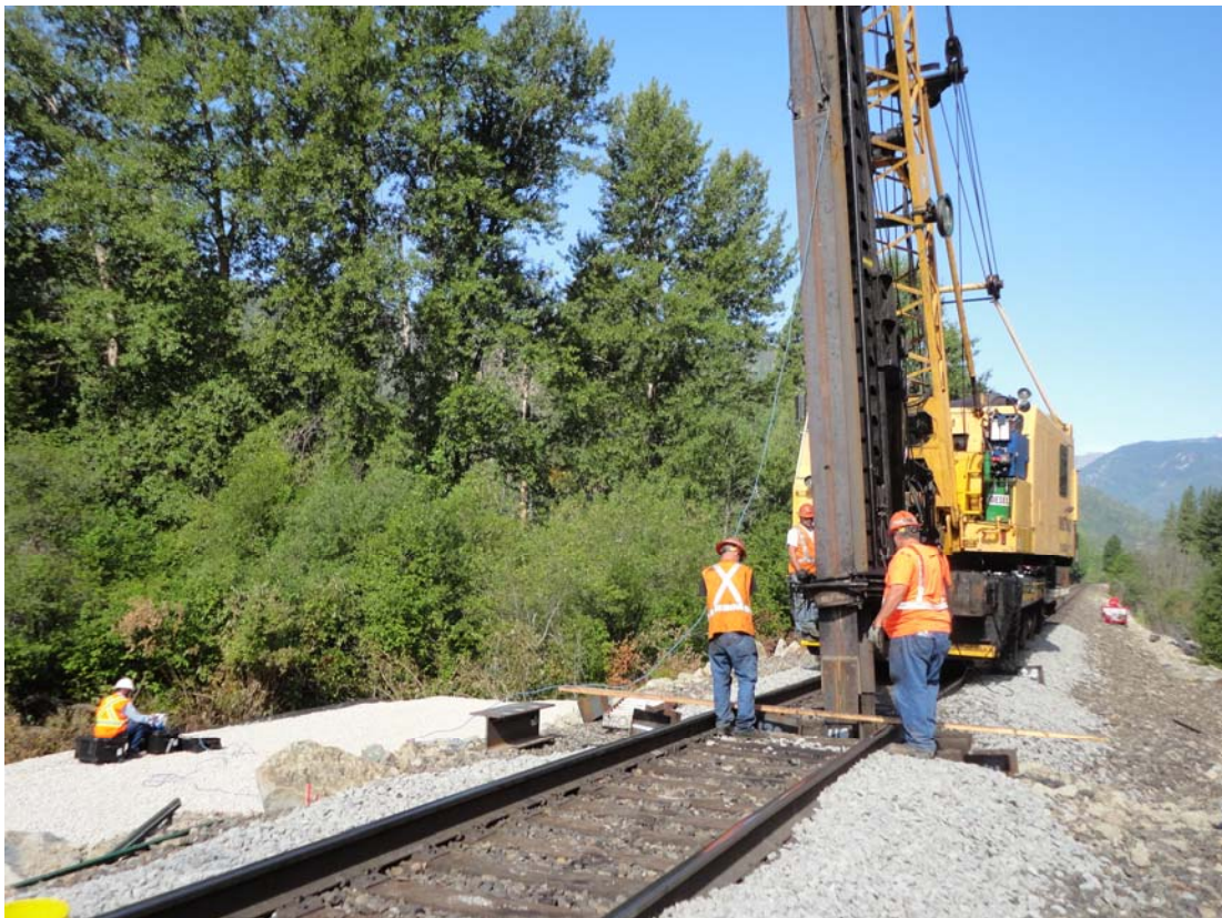
Photo 2: View of BNSF using the follower to collect restrike data from Bent 3 Pile 3. Note the blue wire going from the follower to the computer that Bert had setup.
