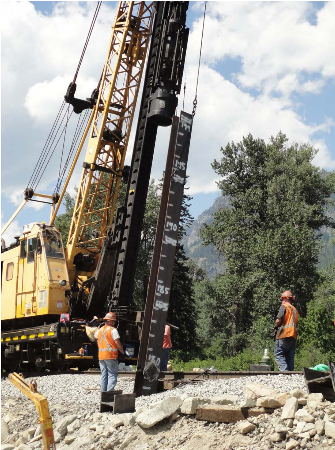
Photo 4: View of Bent 2 Pile 1 Segment 4 at the beginning of pile driving. Note the splice stiffener plates at 179 feet.
