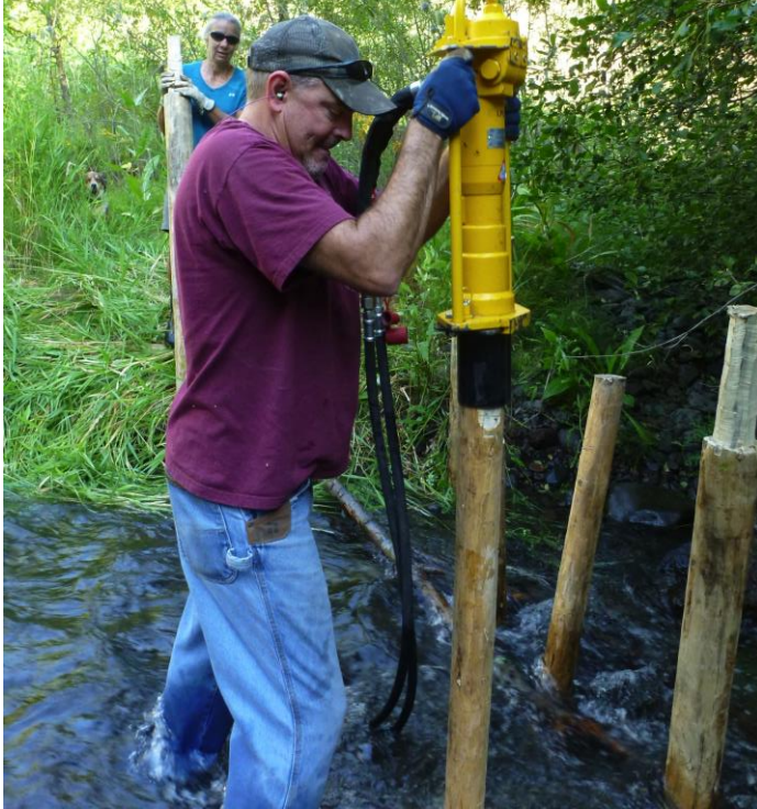
Figure 7. Example of the hydraulic post driver that is used to install large woody debris structures in Asotin Creek.
