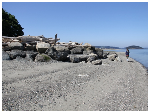
Rock groin extending into lower intertidal (5-9-13)
