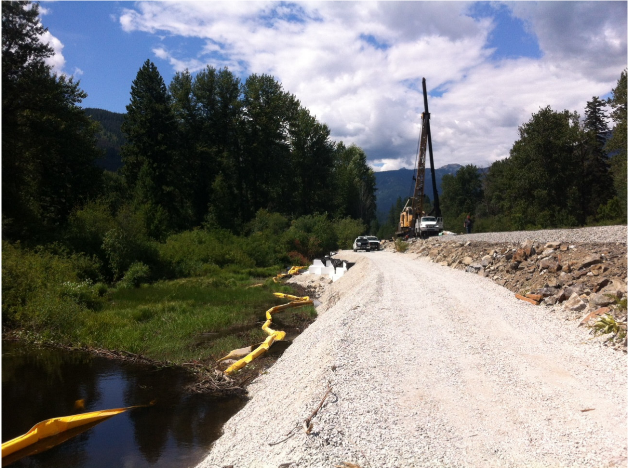
Photo 2: View of the site looking west. BNSF crew is welding segment 3 at Bent 4 Pile 1 at a depth of approximately 121 feet.
