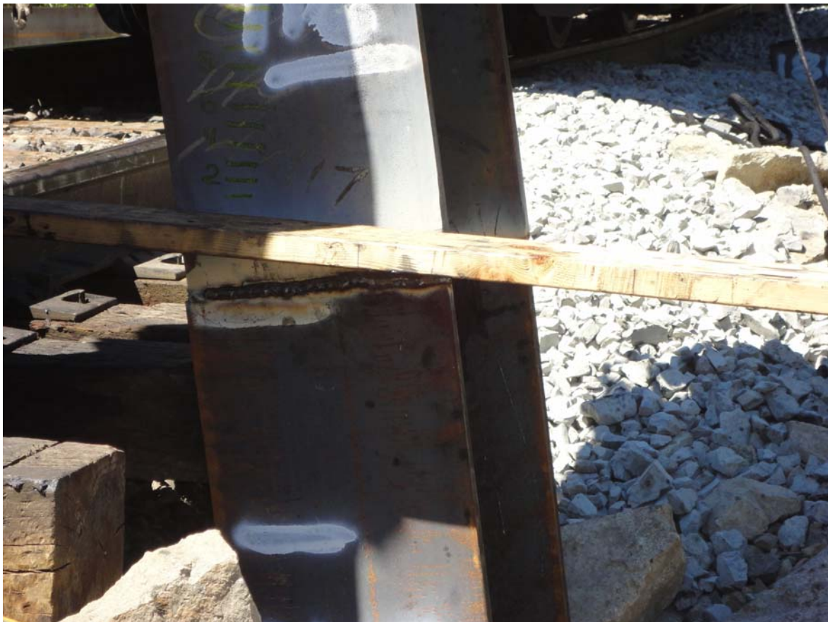
Photo 2: View of the Bent 1 Pile 4 weld at 117 feet. Yellow crayon marks used for collecting restrike data are visible on the pile.
