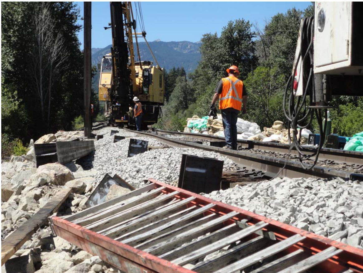
Photo 4: View of the railroad tracks. Note the deflection in the railroad tracks that has been caused by pile driving.
