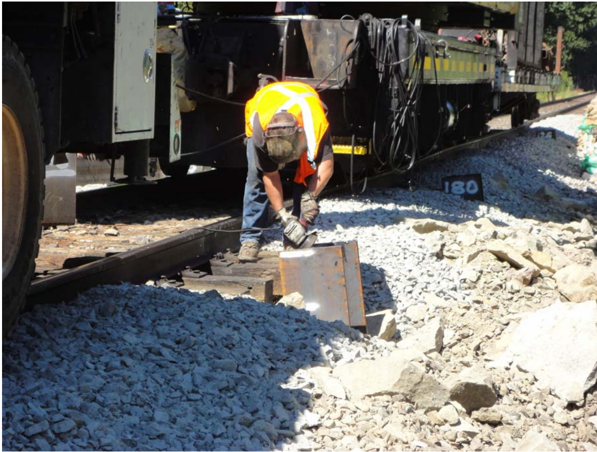
Photo 1: View of the top of Bent 1 Pile 4 being ground off in preparation for pile welding.
