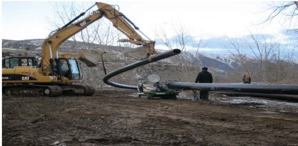
On the left- 3 foot steel pipe from the old gravity canal system, on the right is the new 14 inch HDPE pipe being installed.
