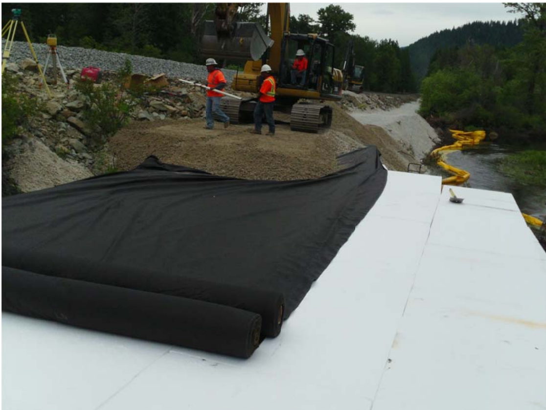
Photo 3 – Placing 1' Thick Layer of Gravel over Completed GLF
