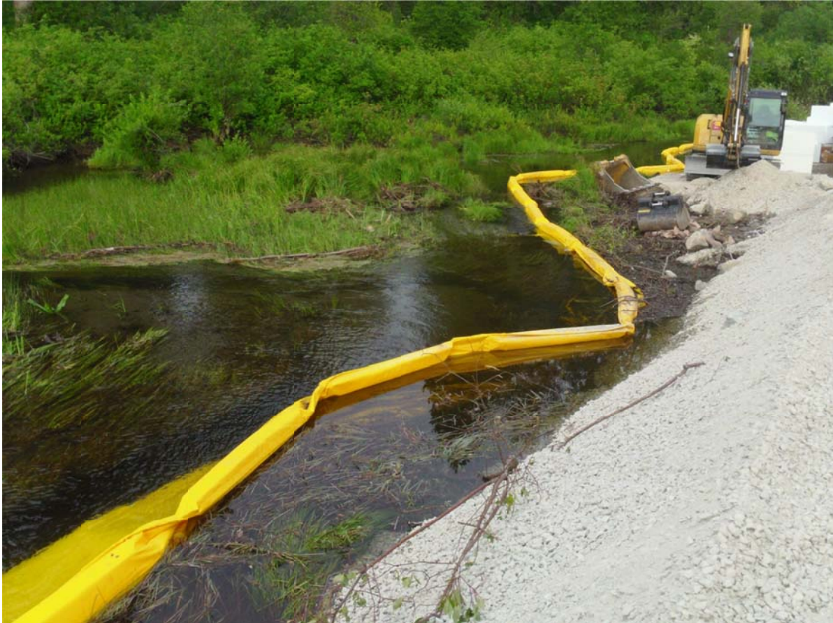
Photo 1 – Floating Silt Curtain Separating Gravel Placement from Oxbow Trib Flow into Nason Creek
