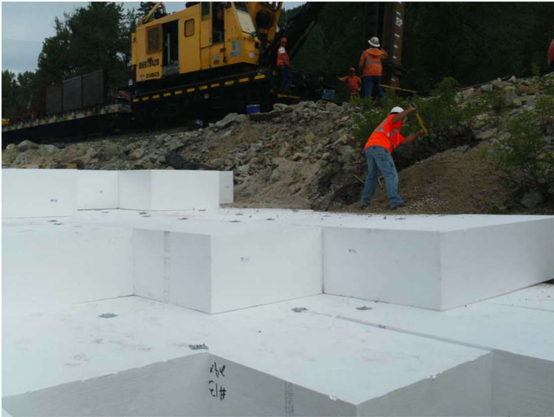
Photo 2 – Filling Gravel in Void between GLF Block and Railroad Embankment
