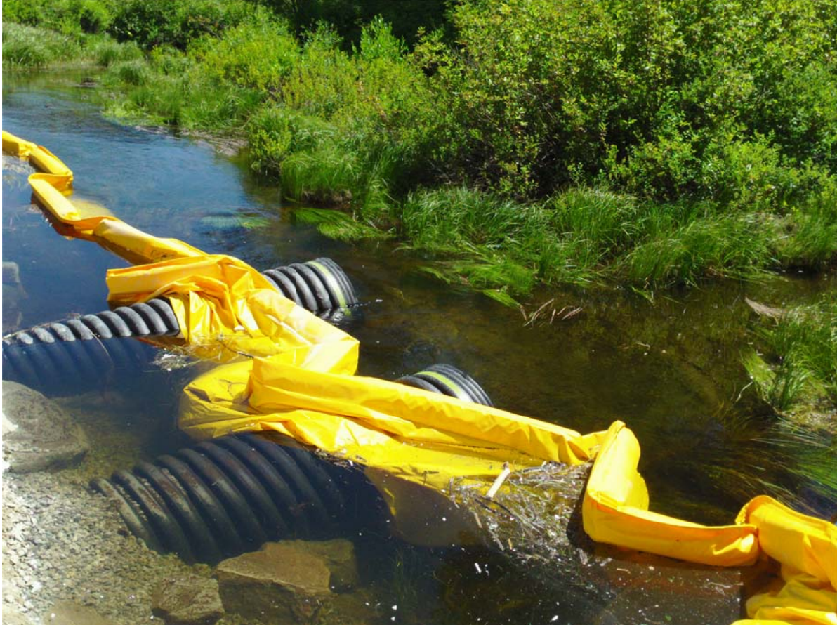
Photo 1 – Two of the Three Culvert Extensions, and Floating Silt Curtain
