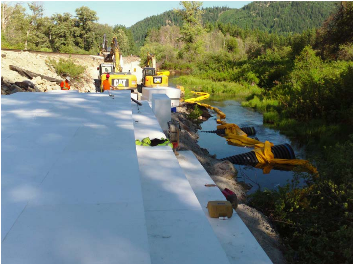
Photo 3 – Geofoam Lightweight Fill Completed to STA 100+56
