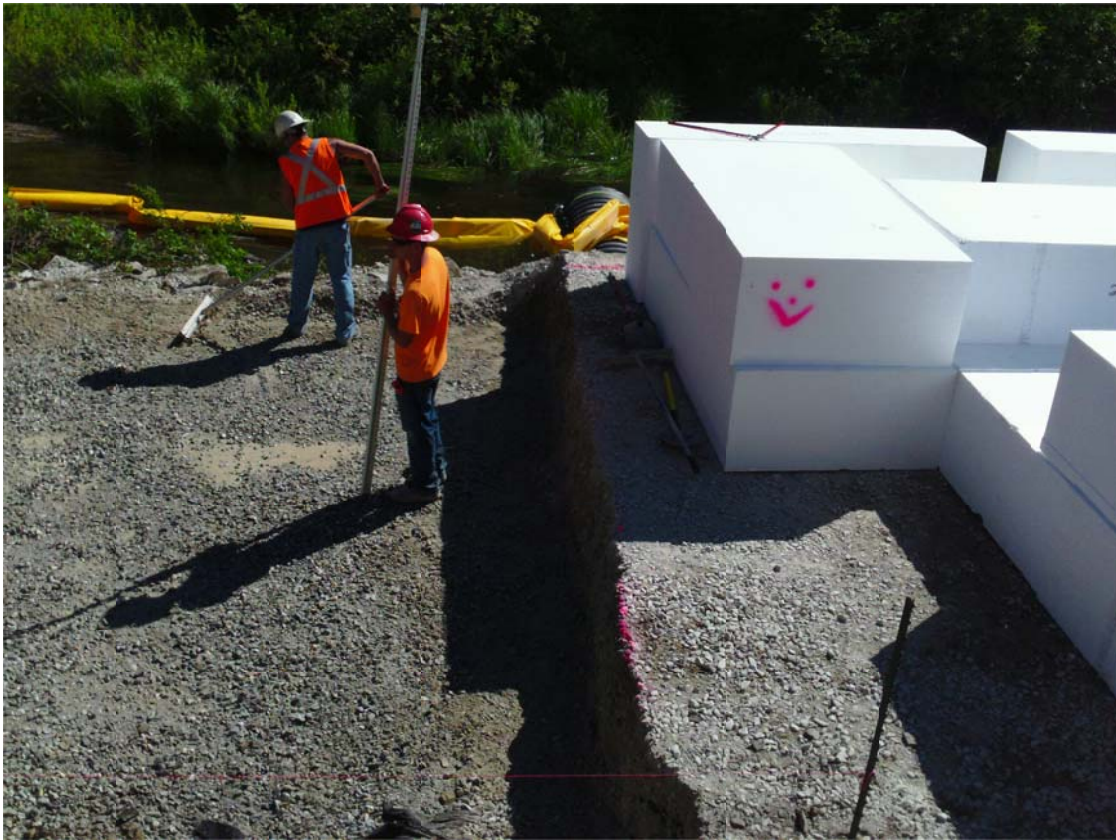
Photo 2 – Preparation of Gravel Fill for Geofoam Lightweight Fill blocks
