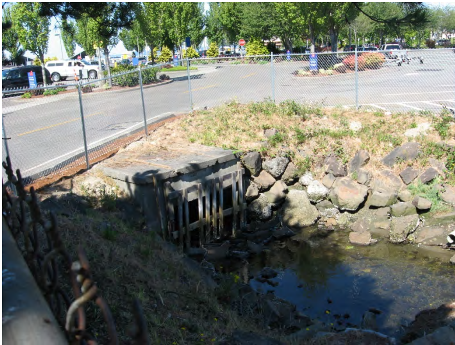
Photograph 10 – Looking downstream Willow Creek outlet to vault underneath Admiral with 48-inch concrete pipe.
