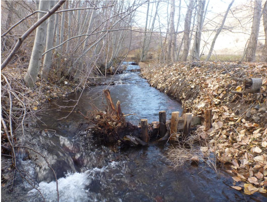
Figure 28. Example of a trial restoration structure on Charley Creek (CC-TX1). A root wad was added to this DWS to aid in forcing a width constriction to this straight and homogenous portion of channel (flow is towards the reader, structure is placed on river left). Note the steep banks and coarse material. CC-TX2 and CC-TX3 can be seen 25 m and 50 m upstream from CC-TX1.
