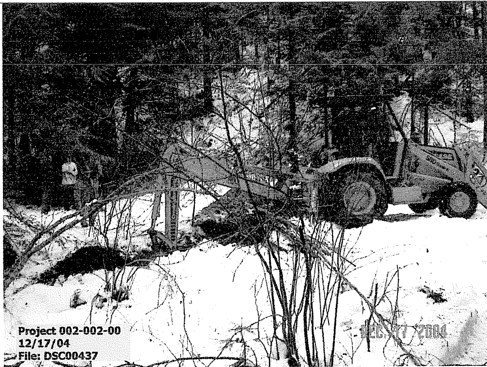
Photograph 1. View looking to southeast from existing bridge. Explorations completed with Case 580 backhoe. Test Pit 1 location.
