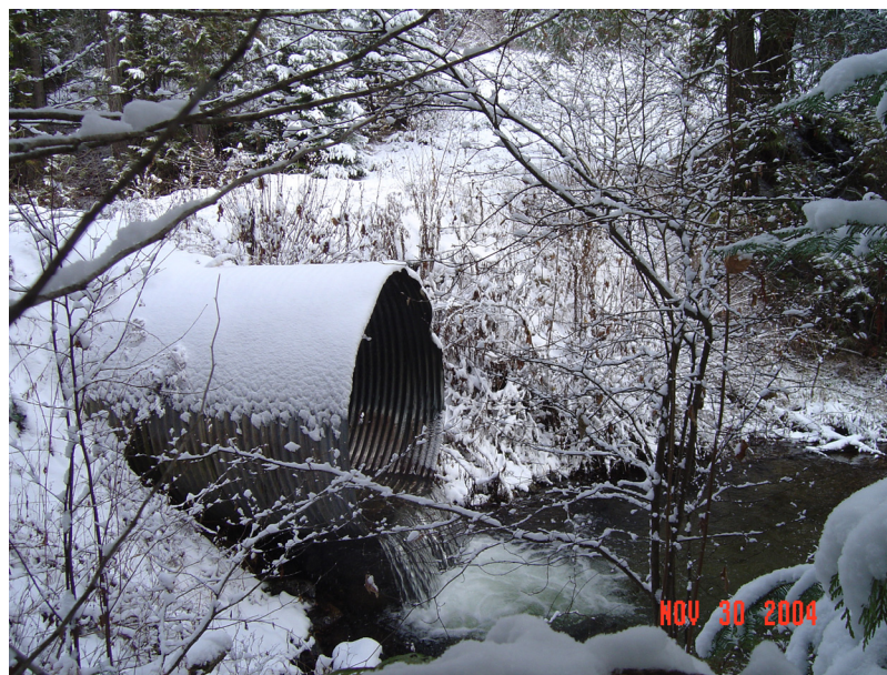
Figure 2: Fish blockage at existing culvert located approximately 1.5 miles upstream on Barnaby Creek.
