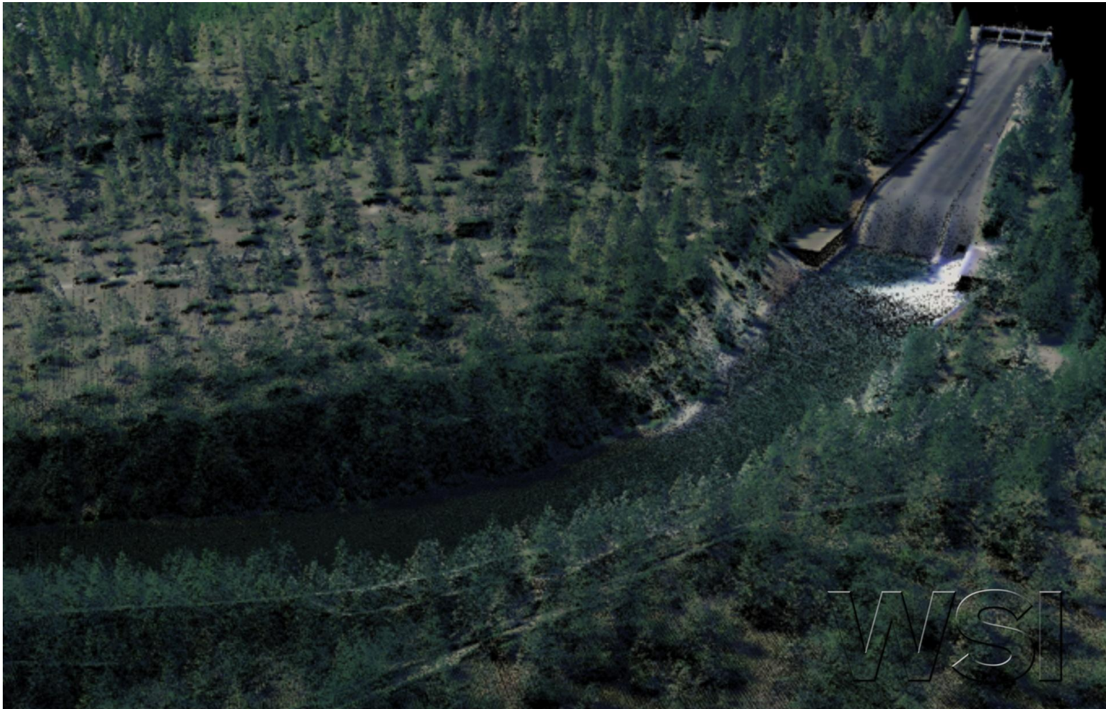
Figure 14. 3D point cloud colored by 2009 NAIP imagery, looking northwest at the Cle Elum Dam
